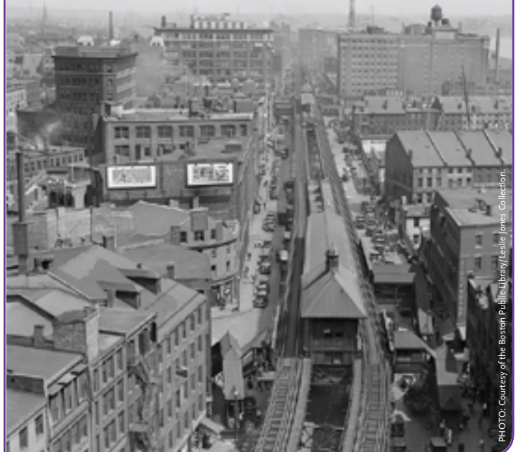
Elevated station at Rowe's Wharf on Atlantic Avenue.
