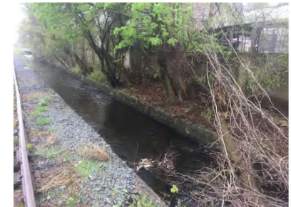
Photo of Existing North Canal Wall
