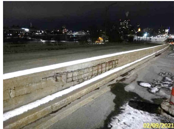
Typical Spalling along the Median Barrier
