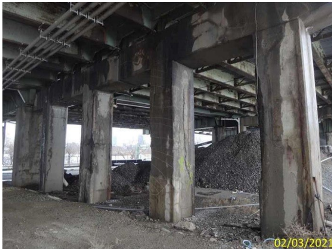
Typical Deterioration to the Pier Bent
