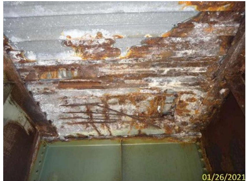
Typical Corrosion to the Stay-in-Place Forms with Spalling to the Deck
