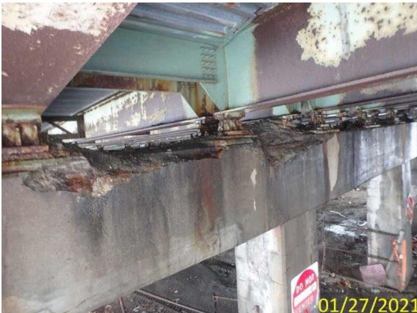
Concrete Spalling at Pier along Bridge Seat
