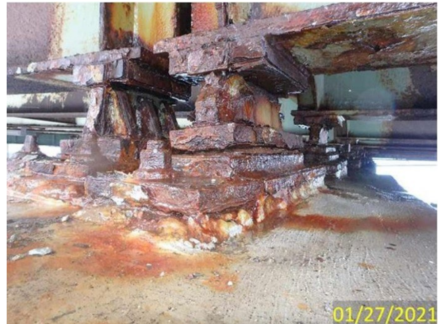
Typical Corrosion to the Stringer Ends and Rocker Bearings
