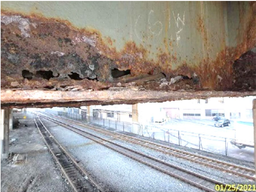
Heavy Corrosion in Lower Web of Steel Pier Cap Cross Girder
