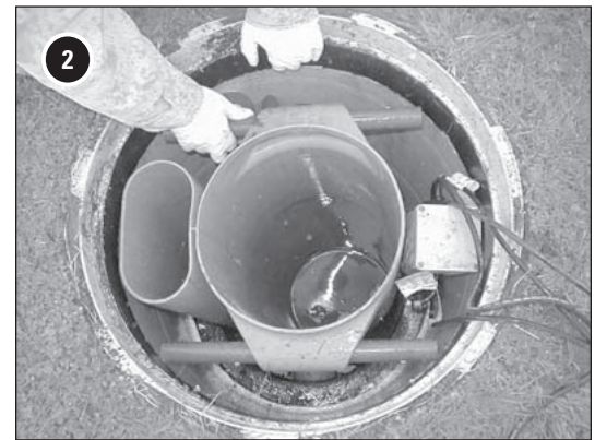
Step 2: Lowering vault into riser
