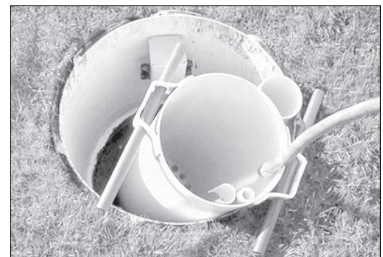
Important: Sinking the vault
