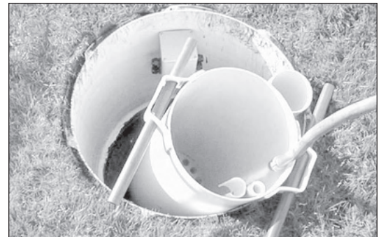
Important: Sinking the vault
