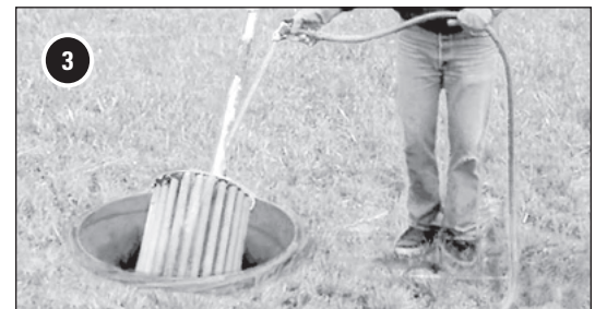
Cleaning the filter cartridge
