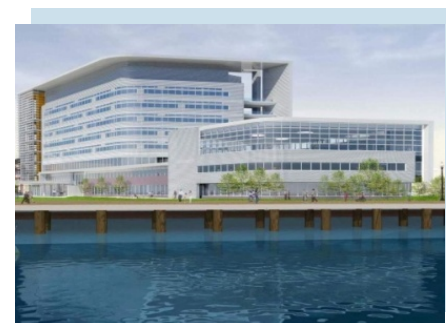
Spaulding Rehabilitation Hospital's new facility in Charlestown Navy Yard.
