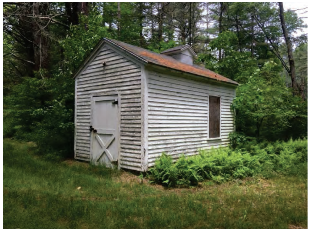
Figure 4-32. QPC Pump house
