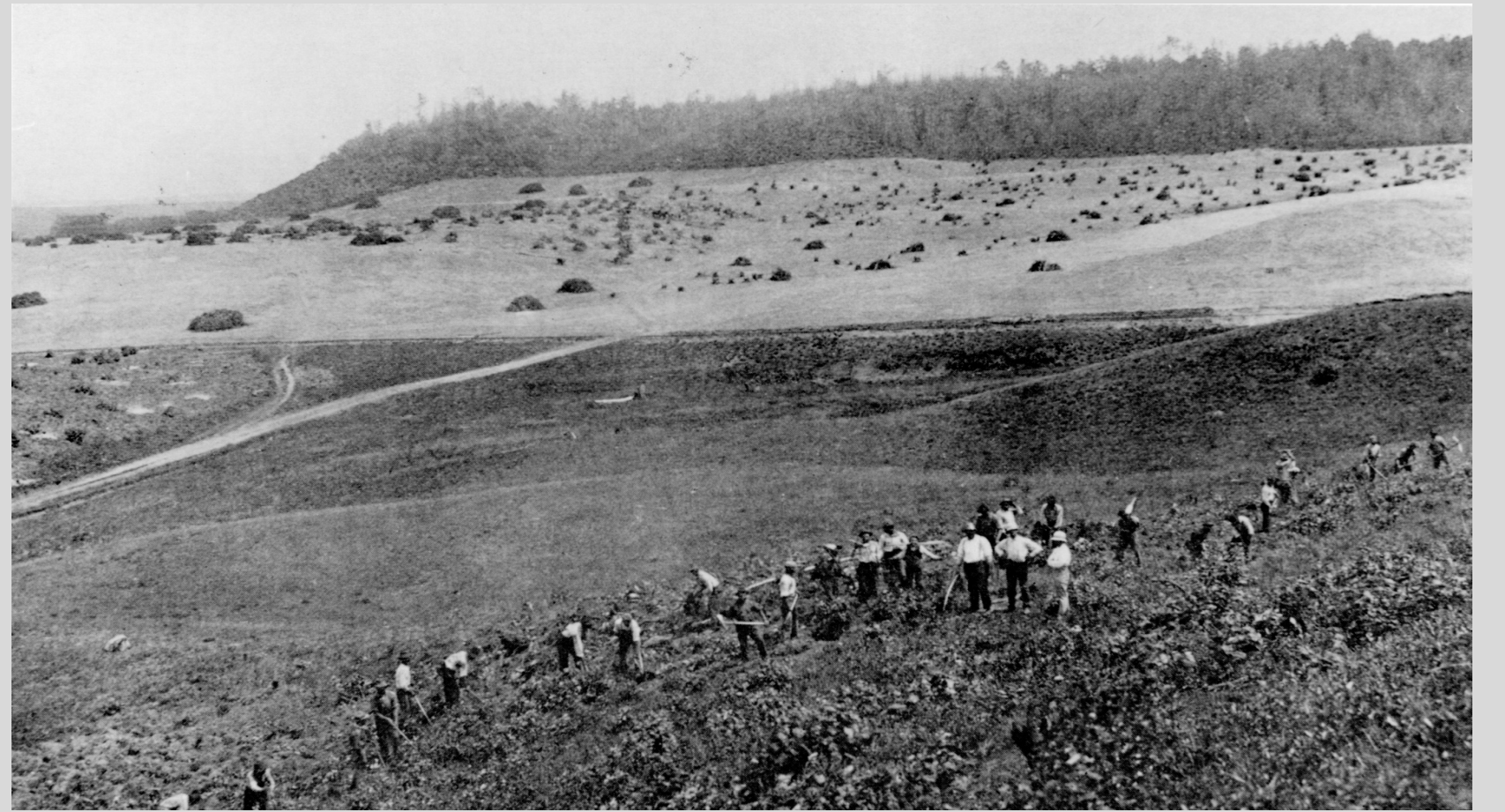
Laborers clearing the area to be flooded to create the Wachusett Reservoir. Built between 1896-1906, the construction came just before the availability of gasoline powered hydraulic engines.
