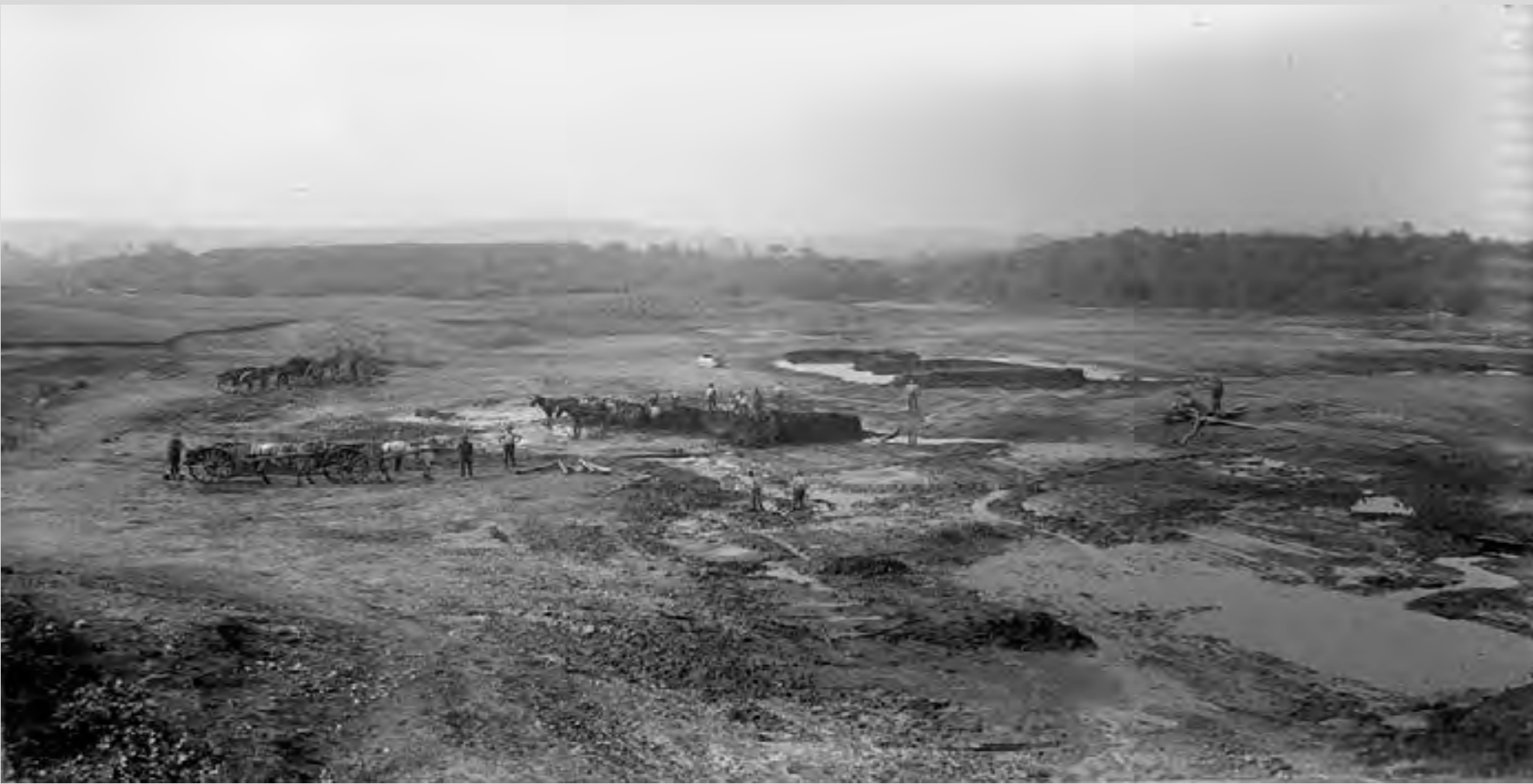
Photo of laborers clearing land for Sudbury Reservoir c. 1875. All told, construction required moving about 4.5 million cubic yards of soil and boulders.
