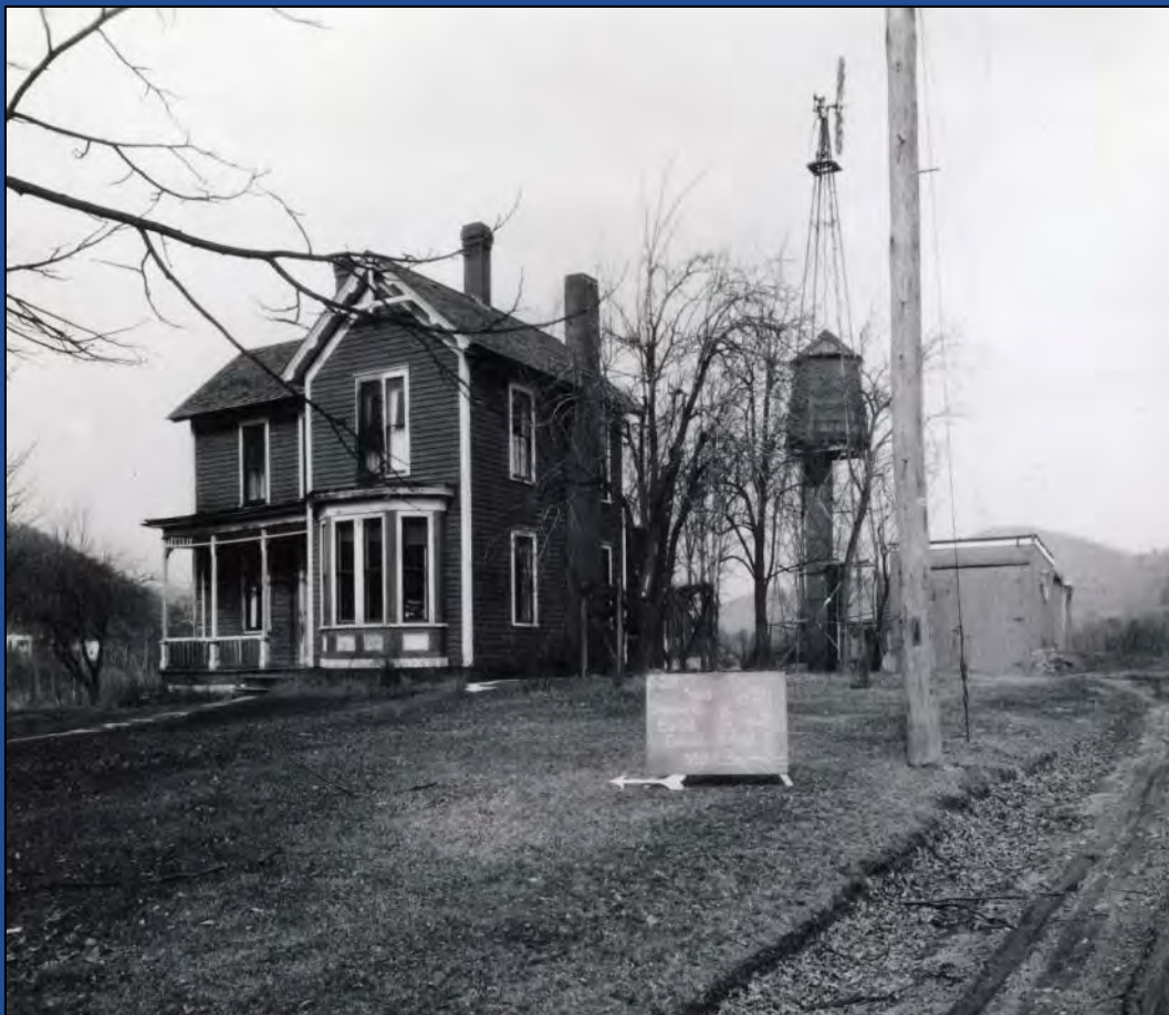
A rare photograph of the water tower in Enfield. The trains would stop to refill water supplies which were used to produce steam. The water was pumped up into the tower by windmill visible over it. (DCR photo)
