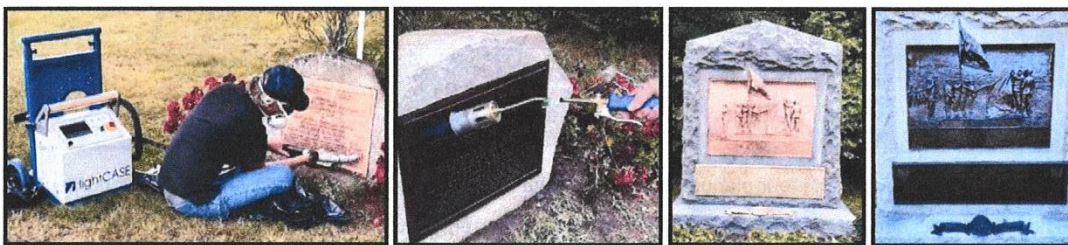
Above, left to right: Chris Henry of Ponsford, Ltd using the LightCase CL100 light laser to remove the patina from the Apremont Park gift plaque, patina is applied with a brush and heated, the 104th Infantry monument plaques after being cleaned with the laser, and an after photo from the patina applied, waxed, and buffed.
