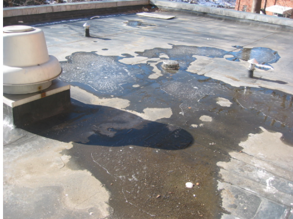
667-3 Development 95 Martensen Street Water-Damaged Roof
