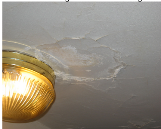
200-1 Development 14 Traffrail Road Paint Peeling on Bedroom Ceiling
