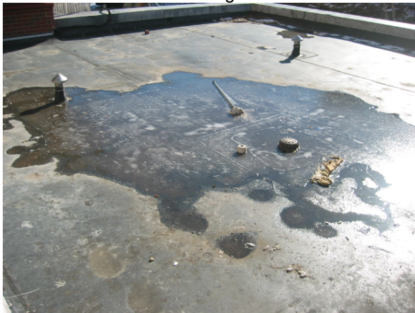
667-3 Development 95 Martensen Street Water-Damaged Roof
