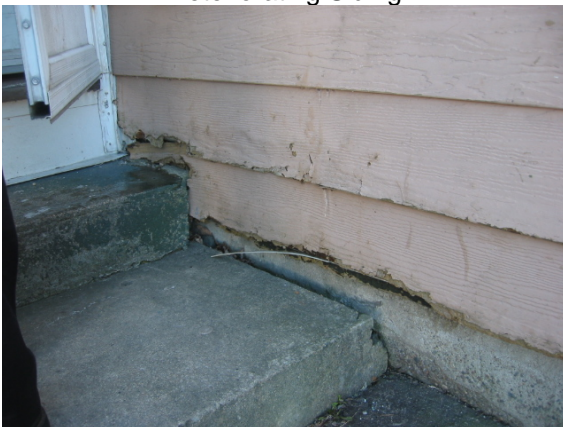
705-2 Development 39 Sullivan Road Deteriorating Siding
