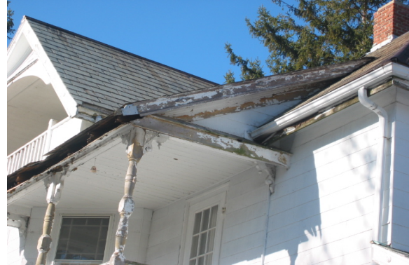
689-1 Development 215 Safford Street Rotted Soffits and Missing Gutters
