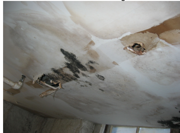
689-1 Development 215 Safford Street Mold and Mildew on Ceiling in Cellar
