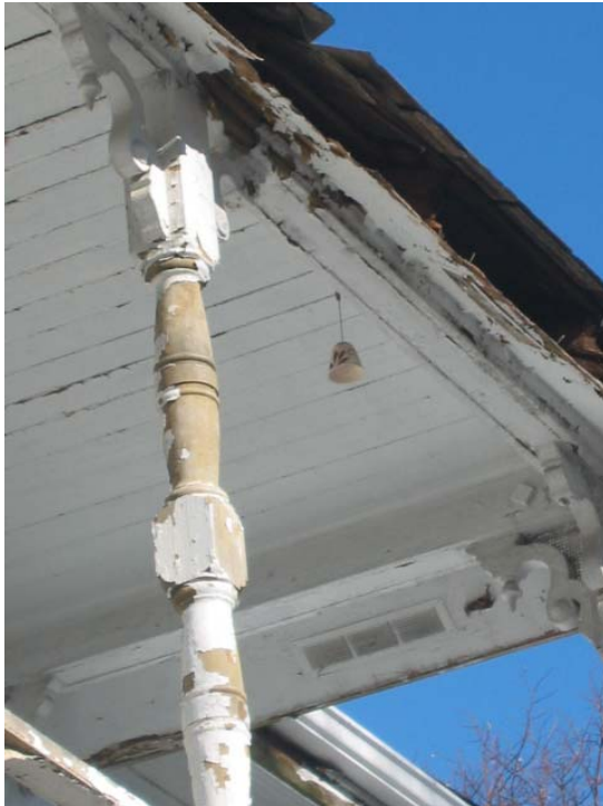
689-1 Development 215 Safford Street Hole in Roof Soffits
