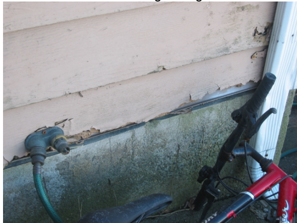
705-2 Development 39 Sullivan Road, Unit #1 Deteriorating Siding
