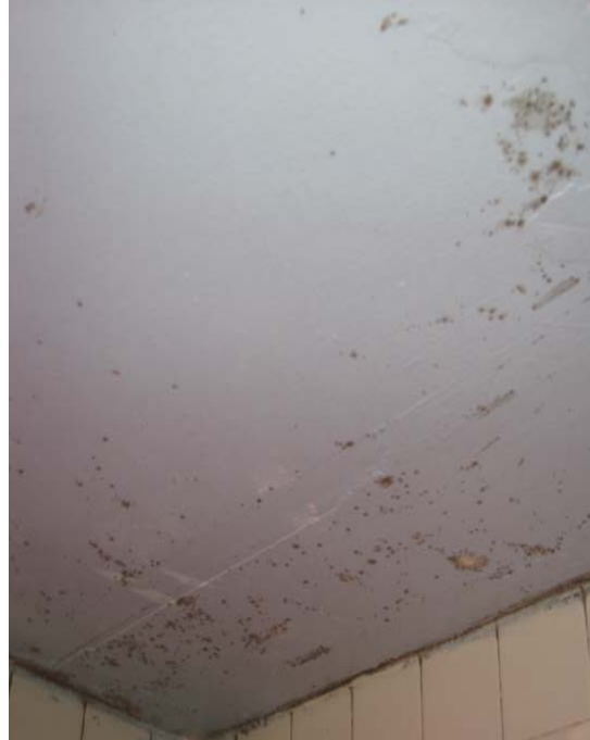
200-1 Development 95 Traffrail Road Mold and Mildew on Bathroom Ceiling
