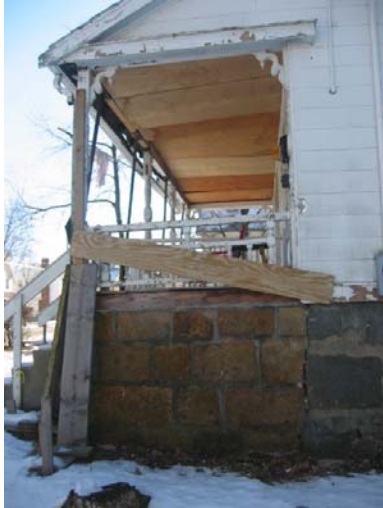
689-1 Development 215 Safford Street Wooden Beams Supported by Two-by-Fours
