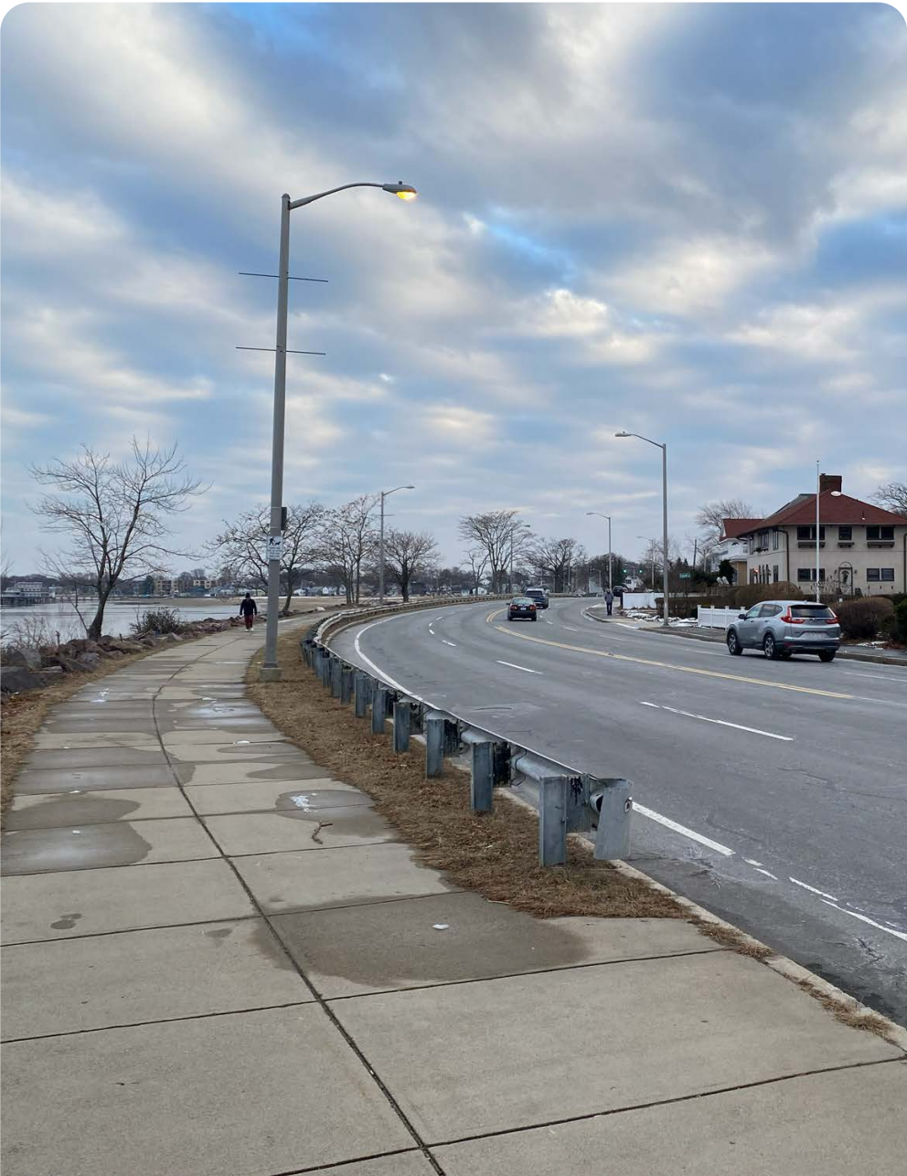
View of Project Site, February 2025
