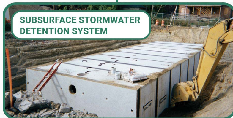
Precedent Image (Source: Advance Concrete Products)
