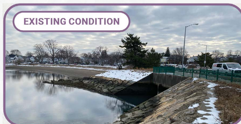
Photo approaching the bridge looking South
