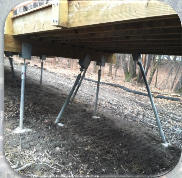
Helical Pile Supports
