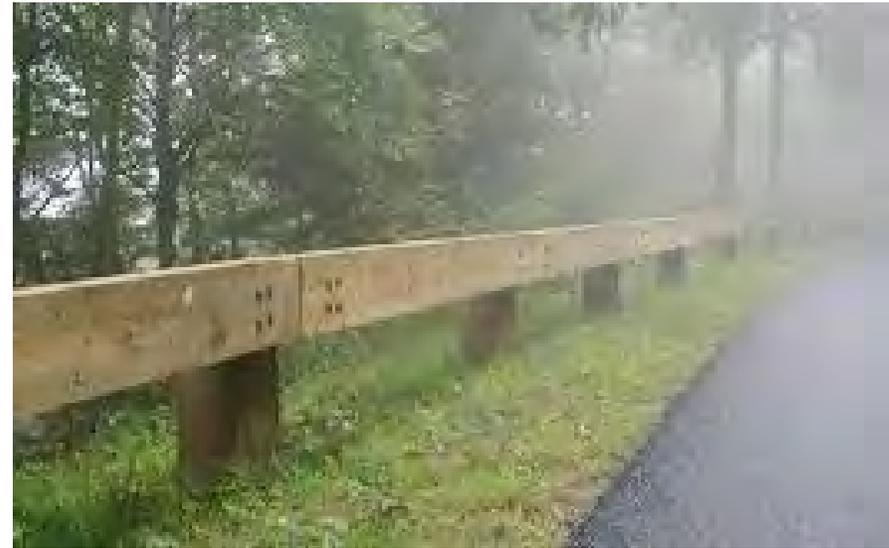
Steel-backed wood guardrail—front
