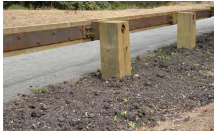
Steel-backed wood guardrail—back
