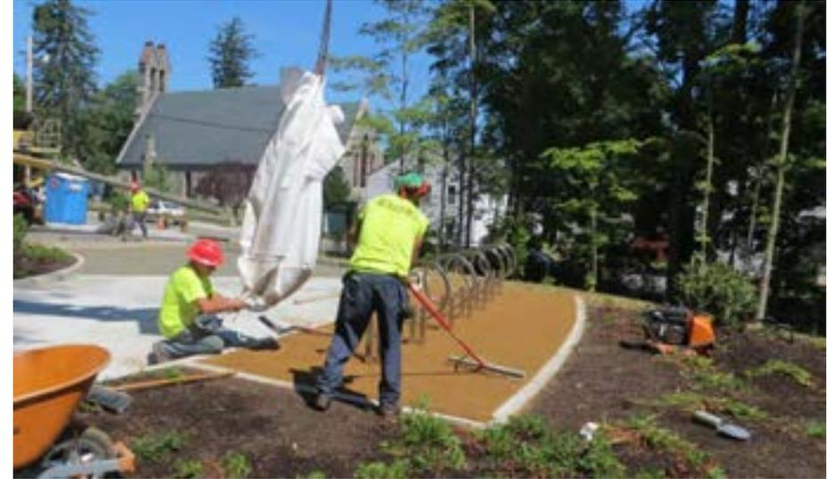
StaLok aggregate—high traffic/slope
