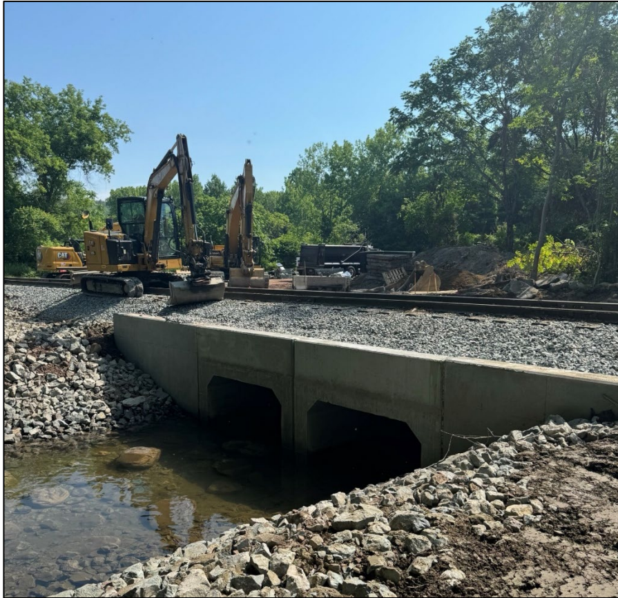
A recently-reconstructed culvert in Adams, MA
