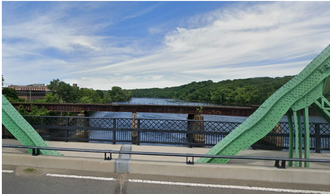
View of the rail bridge, looking northeast, from the Willimansett Bridge over the Connecticut River
