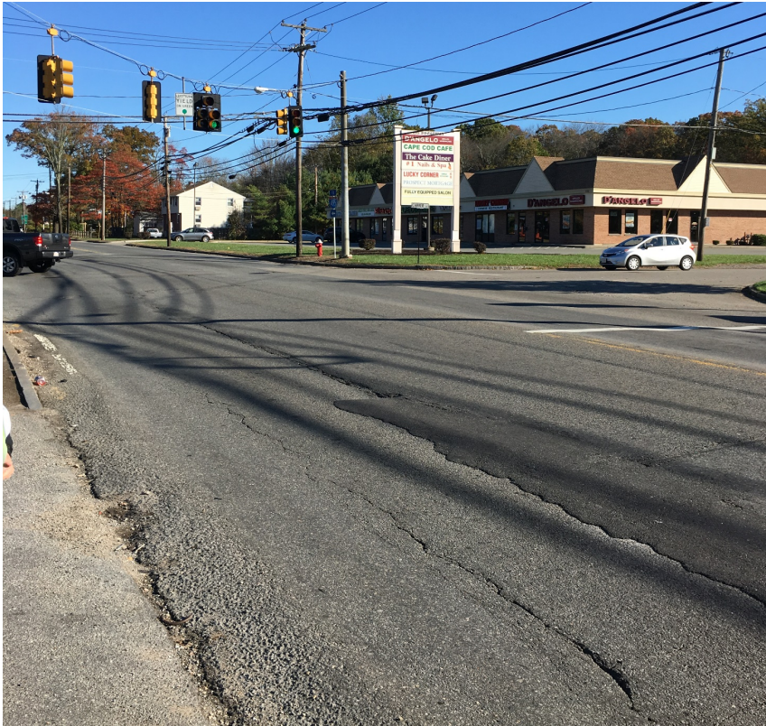
Poor pavement and missing markings at Carver Street intersection looking north
