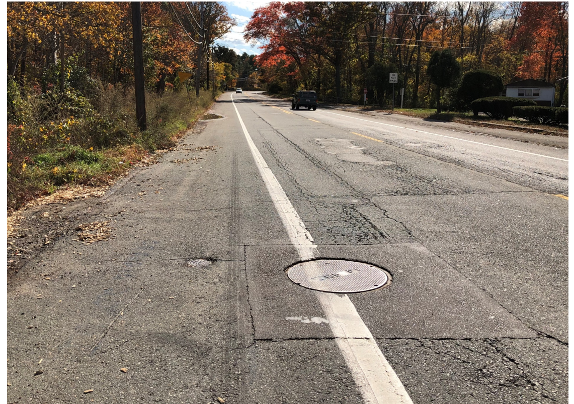
Patching and cracking on the Route 138 Northern segment looking south
