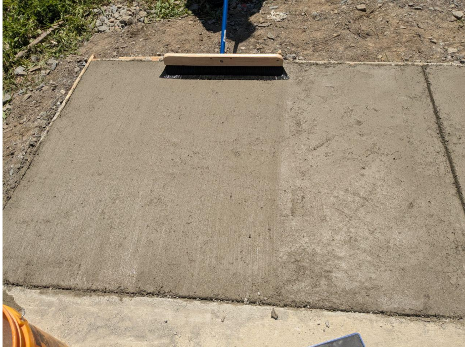
Figure 3.21: Broom finish application for sidewalk texture
