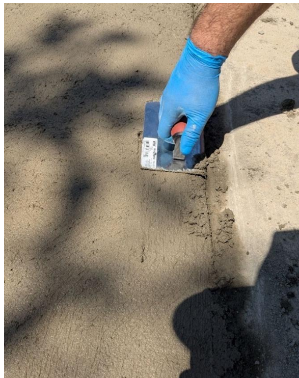
Figure 3.18: Edging process for sidewalk slabs
