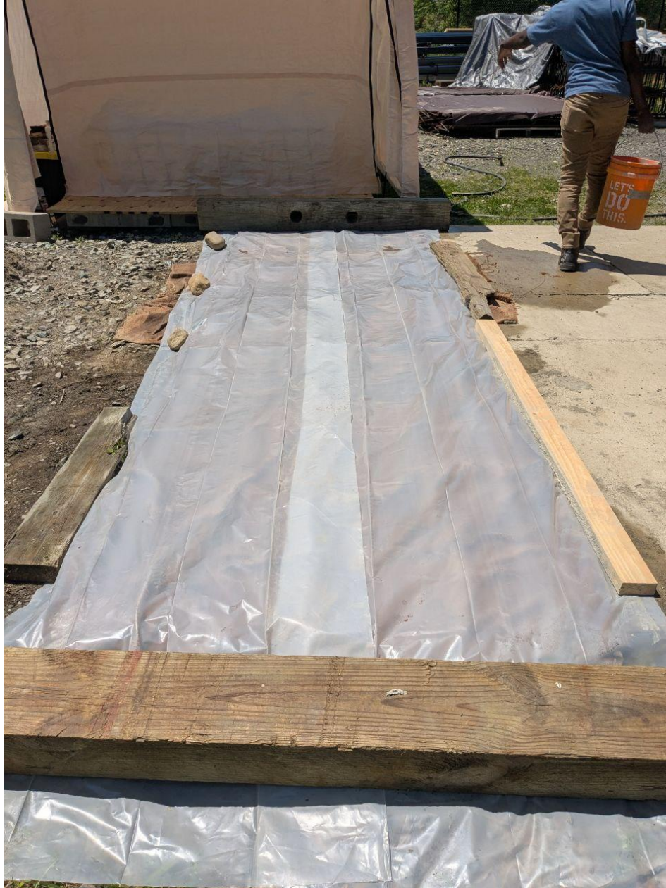
Figure 3.22: Wet burlap and plastic covering for moisture retention
