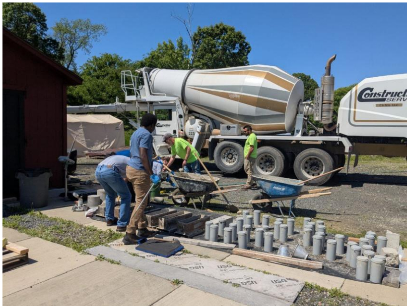
Figure 3.14: Concrete beam and cylinders cast alongside slab placement
