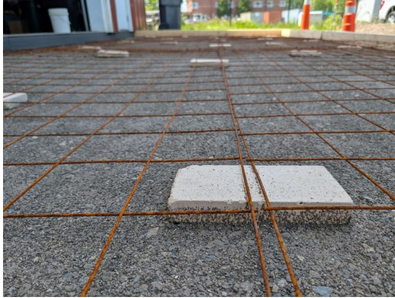
Figure 3.12: Pre-placement setup for sidewalk construction with 100% hydraulic cement concrete
