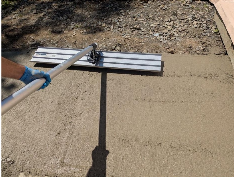
Figure 3.17: Initial finishing of concrete sidewalk with magnesium bullfloat
