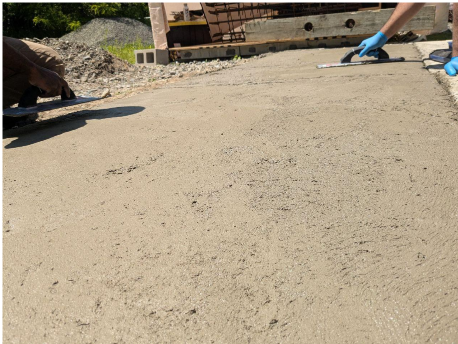
Figure 3.20: Magnesium troweling for surface finishing
