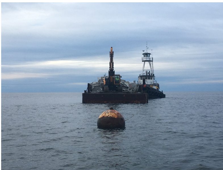
Figure 2. Material Deployment on January 6, 2020.
