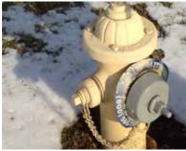
Fire hydrant fitted with EchoShore-DX smart nodes.
