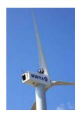
**Wind**—Two 600 kW "conventional" turbines, generating approximately 2 million kWh of electricity per year, and one 100 kW FloDesign prototype turbine.
