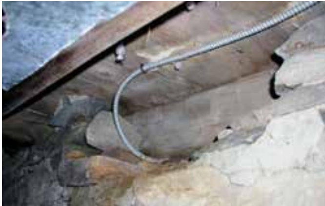
Fig. 6.9. The sill of the house is exposed to the basement interior in only a couple of spots; therefore an accurate determination of its condition is difficult without more extensive testing and/or removal of exterior cladding.
