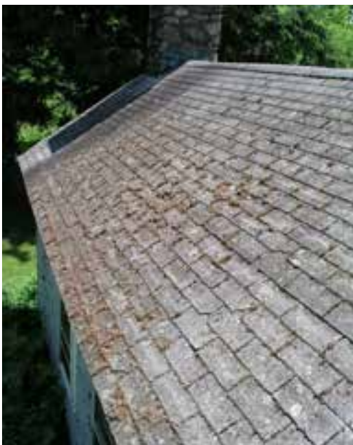
Fig. 5.2. Condition of shingles at ell.
