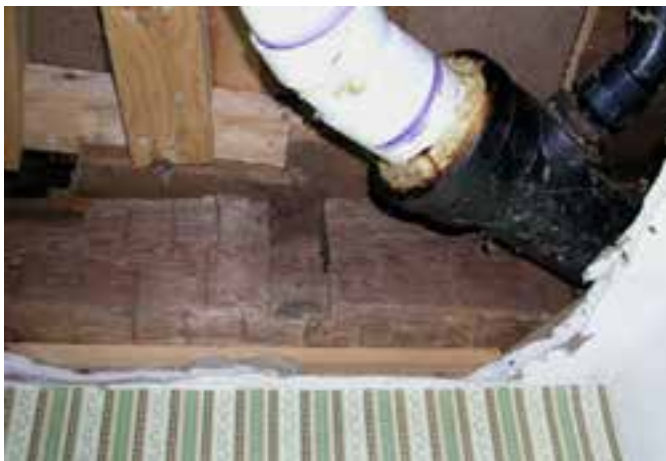
Fig. 6.11. Hand-hewn beam and modern additions.
