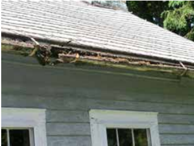
Fig. 5.4 Rotted gutter section.
