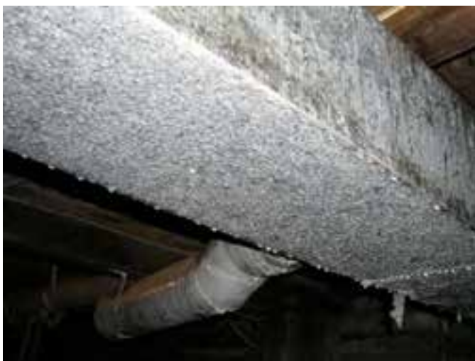
Fig. 5.5. Extreme humidity in basement aggravated by uncontrolled roof runoff is deteriorating structural framing and HVAC equipment.
