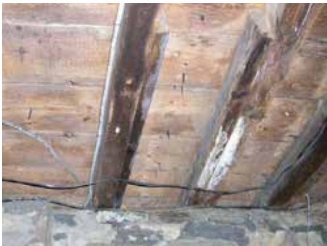
Fig. 6.10. First floor framing evidencing mold growth.
