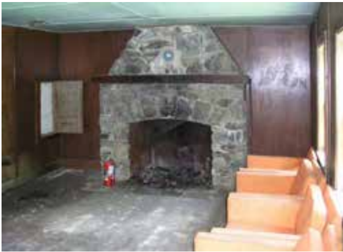
Fig. 6.8. Stone fireplace in ell. Note also the wood paneling, which is in need of renewal.
