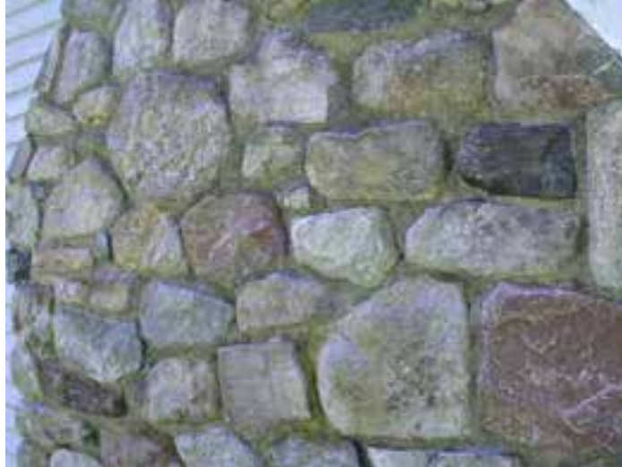
Fig. 5.9. Stone masonry needs spot-repointing.
