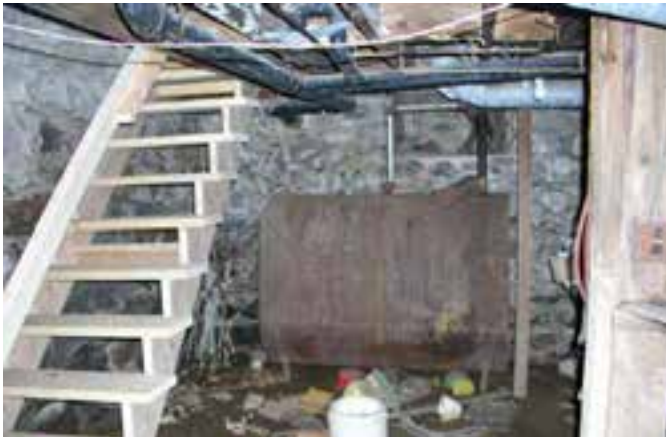
Fig. 4.5. Existing 275-gallon oil tank.
