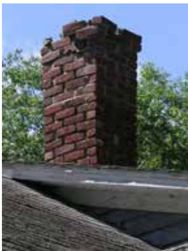
Fig. 5.10. Brick (flue) chimney.
