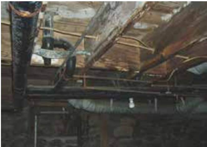
Fig. 4.1. Typical condition, basement ceiling (first-floor framing).
