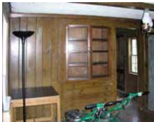
Fig. 6.6. Paneling and beams at Dining Room. Note apparent difference in wood species between paneling and glass-fronted cupboard.
