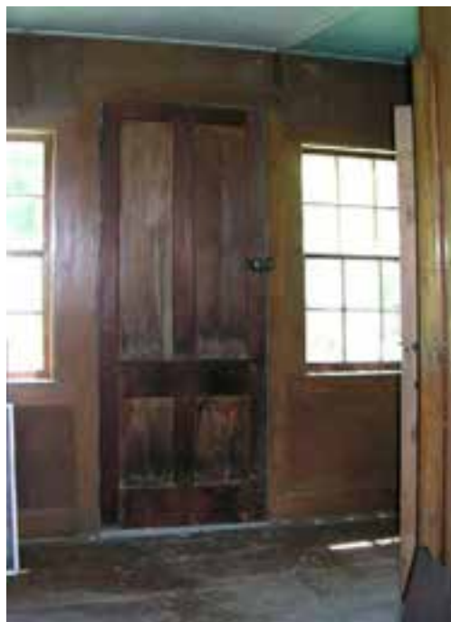
Fig. 5.13. Interior face of recessed-panel door at ell.
