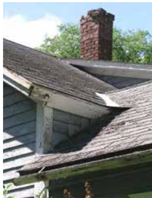
Fig. 5.3. Existing valleys and stepped flashing.
