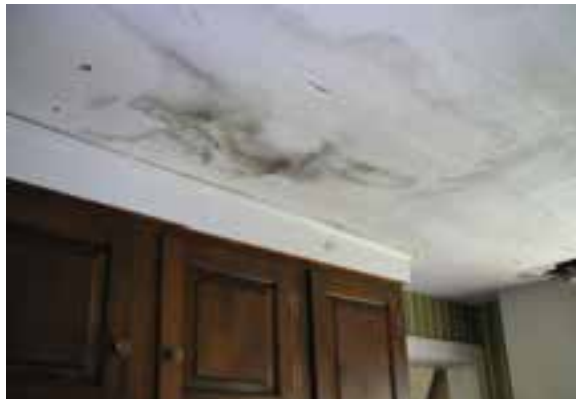
Fig. 6.5. Water damage and mold at kitchen ceiling.
