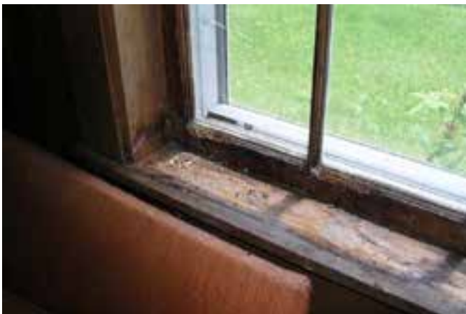
Fig. 5.7. Ell window; note damage to stool and sash.
