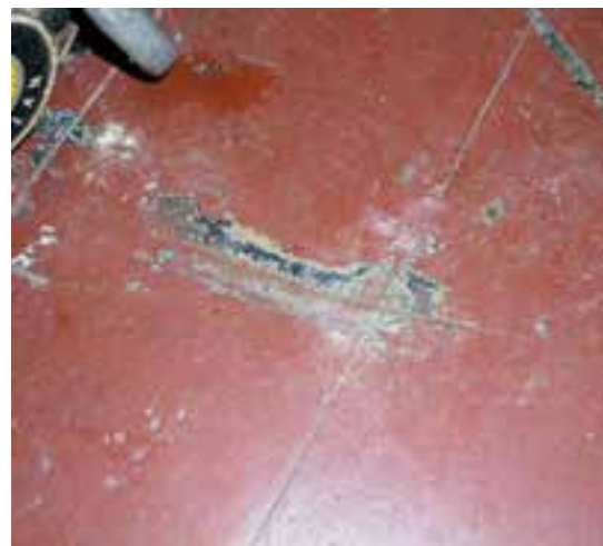
Fig. 6.4. Scratches on painted pine wood floor at NW parlor reveal an interesting "paint history."
