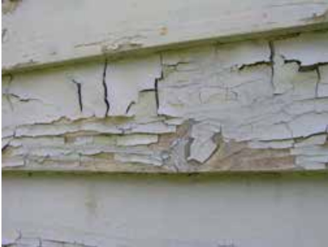
Fig. 5.6. Typical condition at clapboard siding, 2007.
