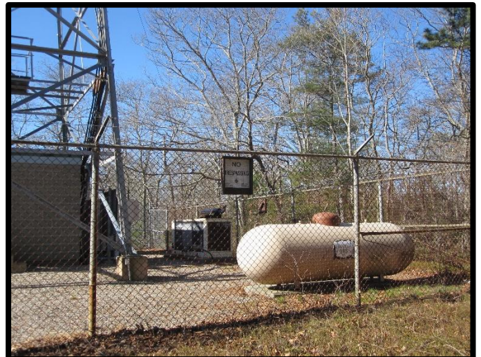
Propane Tank and generator
