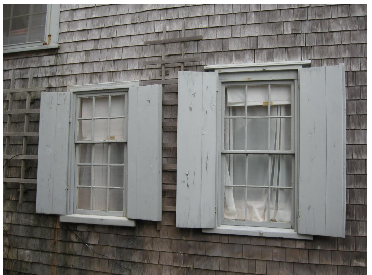
The solid wood storm shutters at 23 Front Street in Siasconset protect the original windows when they are closed during storms.
