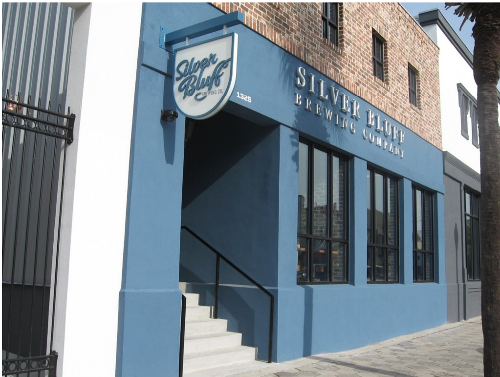
New commercial buildings should have flood-resistant storefronts. This building was designed with a concrete first floor, stairs to the main entrance and an ADA compliant entrance on the side elevation.
