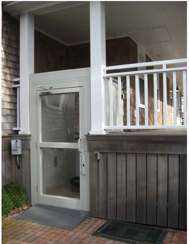
This chair lift design provides access from a dedicated parking space and required only a small section of the porch to be removed (4 Whaler's Lane).
