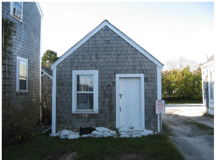
Temporary barriers such as sandbags can be placed at doorways and along foundations (53 Washington Street).
