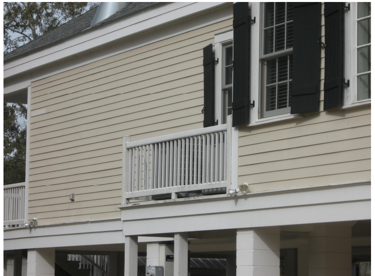
For high elevation projects HVAC units must be on platforms above the required flood elevation level.
