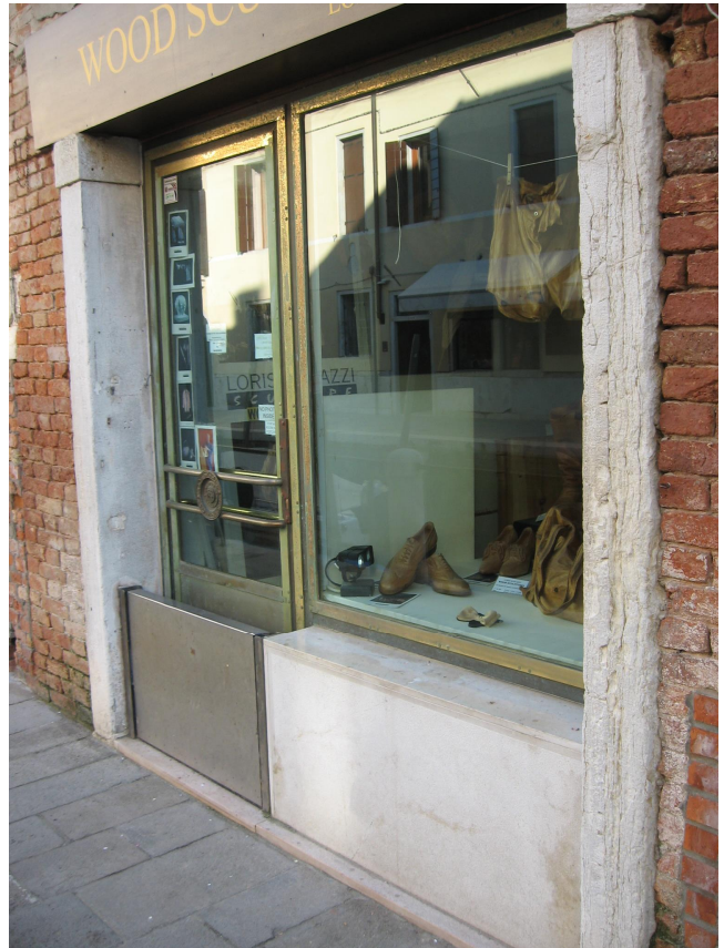
Dry flood proofing may include the installation of temporary flood panels at storefronts (above) or residential doors
