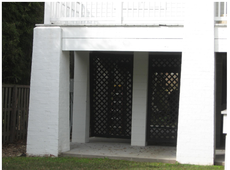
The tapered painted brick foundation piers are designed to match the tapered Bungalow style porch columns on this elevation project.
