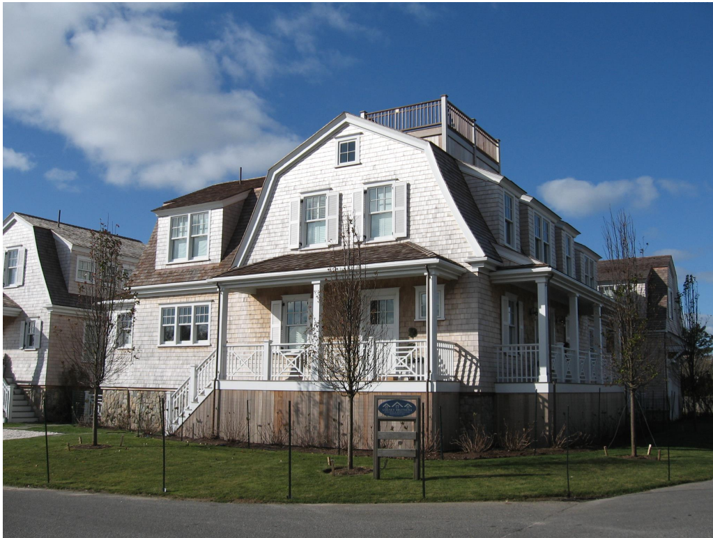
New construction must be built to be above the DFE such as this dwelling at 2 Hulbert Avenue completed in 2019. This dwelling is elevated with a stone foundation and vertical board panels beneath the porch.
