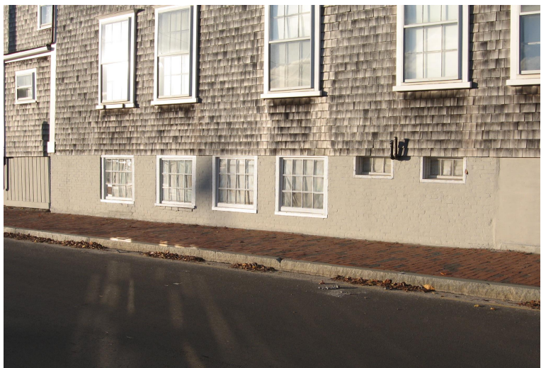
Filling the basement and adapting basement windows into flood vents may be a future strategy for properties in the flood zone ( 6 Union Street).
