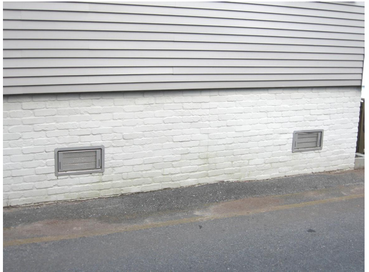
Appropriate flood vents in the brick foundation at 42 Fayette Street (above and below).
