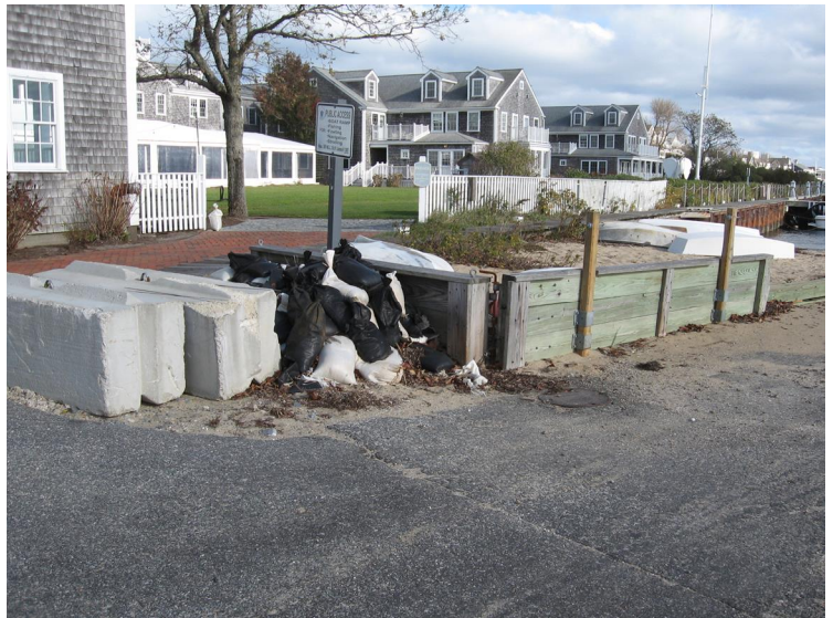
Temporary barriers include movable concrete panels. At Harbor View Way, these panels are combined with wooden gates and sandbags during periods of high water.
