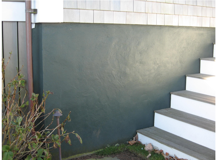
The elevated dwelling at 57 Washington Street has a rebuilt concrete foundation with a parged surface providing a uniform appearance.
