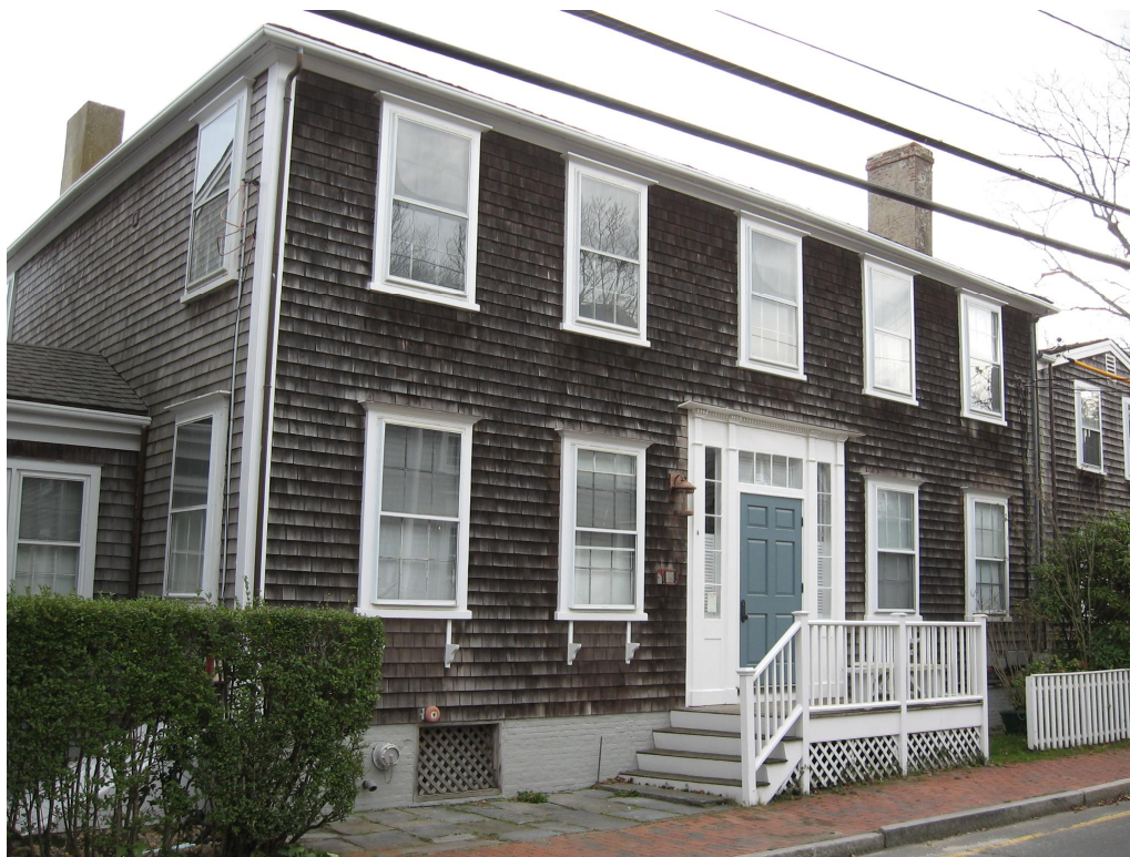
The ca. 1850 dwelling at 6 Union Street has a brick foundation with lattice vent panels, a staircase with square newels and balusters and lattice panels beneath the stair landing.
