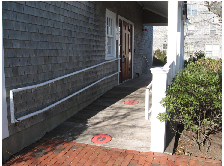
Some low-elevation projects may be able to utilize ADA ramps on the primary façade. Such ramps should be in traditional designs and screened as at 95 Washington Street.
