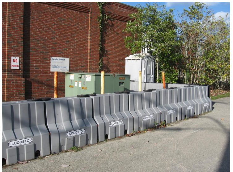
Temporary barriers also include water-filled interlocking plastic units known as "Jersey" barriers (Candle Street Substation).
