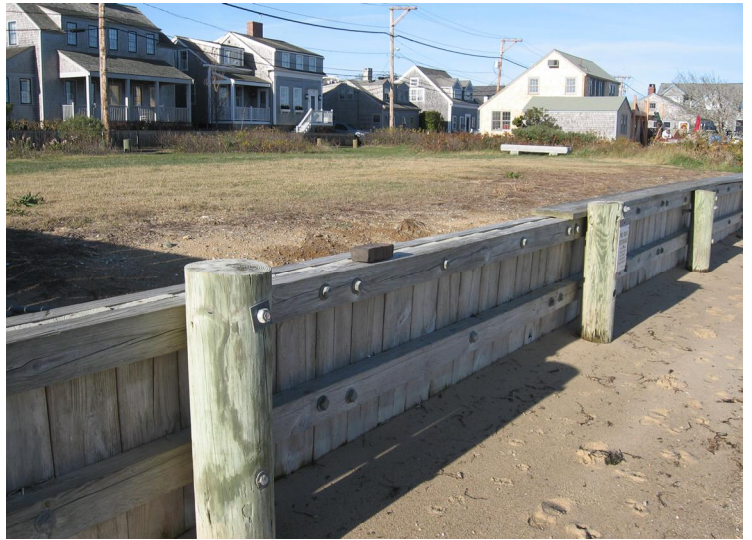
Permanent barriers include levees, berms, and concrete or wood flood walls as this example on Washington Street.
