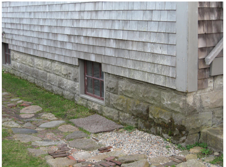
Historic materials such as early 20th century rock-faced concrete block should be salvaged and added to increase the height of the foundation on the primary façade and readily visible side elevations (52 Union Street).
