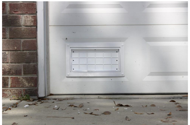
Garage doors must be designed with appropriate flood vents to meet FEMA standards.
