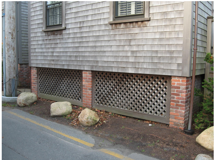
The 2016 dwelling at 11 Fayette Street was designed with an appropriate brick pier foundation and lattice panel screening (above). The front porch and stair have traditional designs with lattice panels beneath (below).
