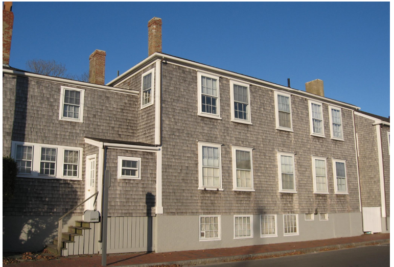
Filling the basement and adapting basement windows into flood vents may be a future strategy for properties in the flood zone ( 6 Union Street).
