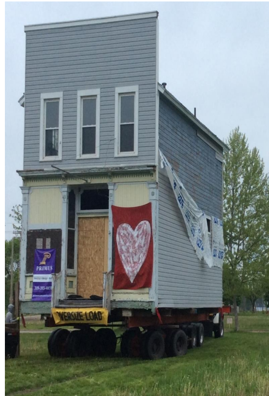
This historic building experienced frequent flooding and was moved to a compatible site. It was relocated on a terraced and elevated foundation.
