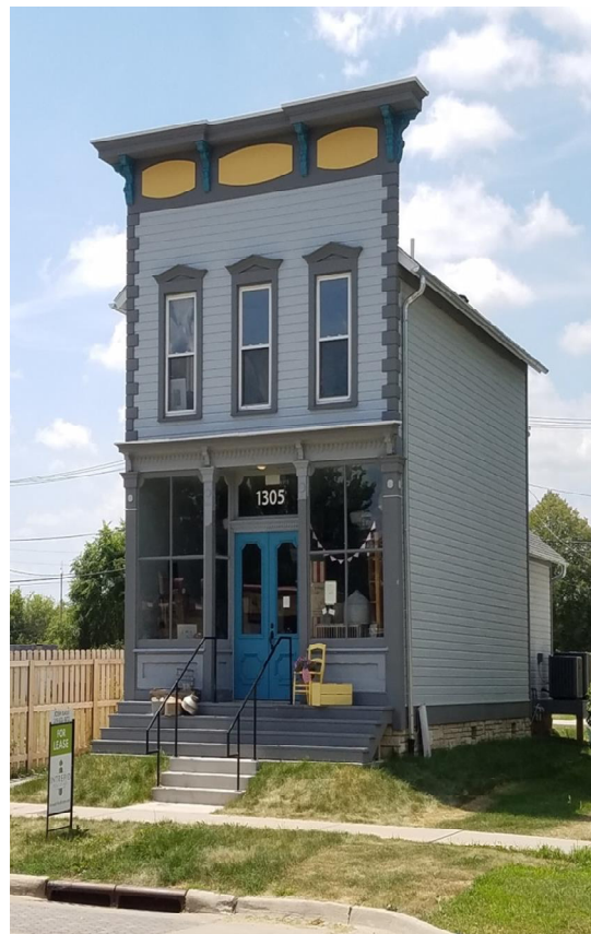
This historic building experienced frequent flooding and was moved to a compatible site. It was relocated on a terraced and elevated foundation.
