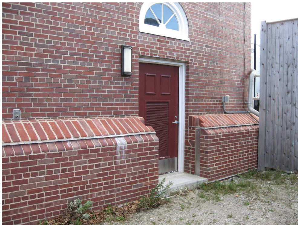
Doorway openings in the added brick skirt wall were fitted with flood shields which could be closed during flooding.
