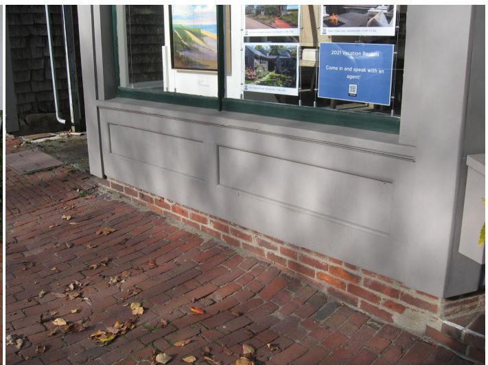
Storefronts with frame bulkheads below the display windows include those at 19 Washington Street (left) and 17 Main Street (right). The design of these bulkheads are appropriate but they are not of flood-resistant materials.
