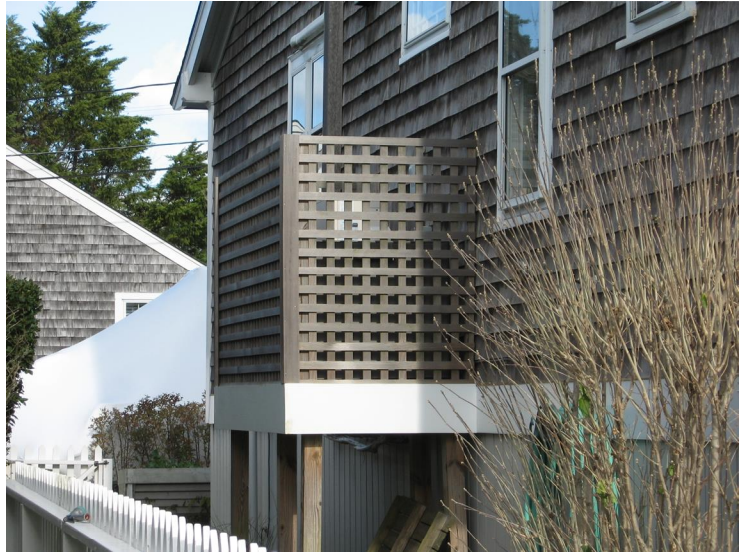
For low-elevation projects, site HVAC units on platforms at the rear on non-readily visible side locations (8 Harbor View Way).
