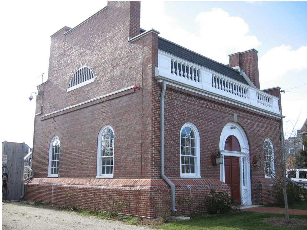
An example of dry flood proofing is the Sea Street Pump Station. The building was hardened through the addition of a concrete and skirt wall which closely matched the original brick material. Pumping equipment was added in the basement which could be submerged during flooding and other equipment was relocated to an elevated platform.
