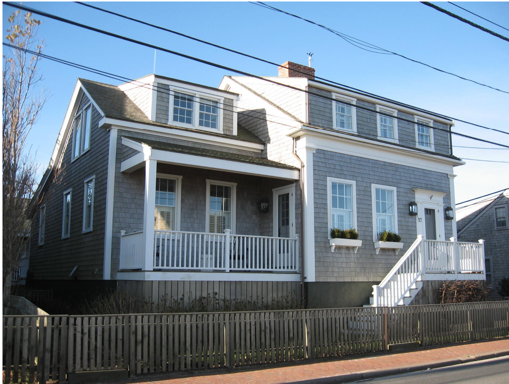
The elevation of 57 Washington Street is another successful elevation project in the Nantucket Historic District (above). This project included adding a new concrete foundation and retaining the chimney at the roofline. The staircase was extended with appropriate detailing and vertical panels were added at the porch foundations (below).
