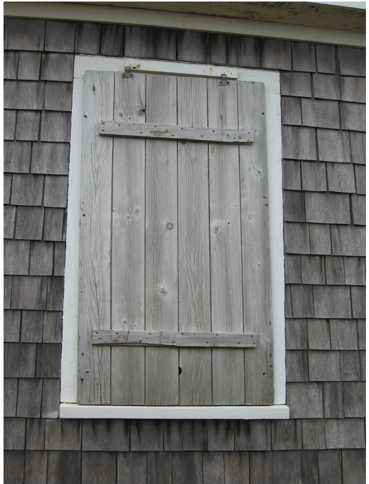
Storm panels are applied to protect windows over the winter and during storms (9 Codfish Park Road).
