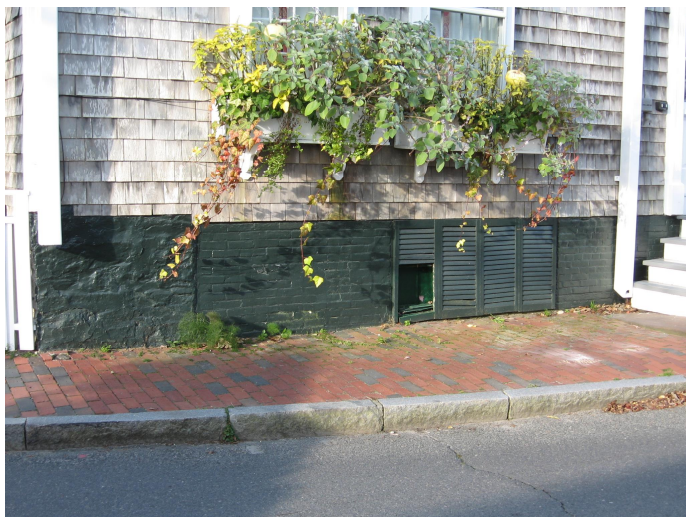
Some dwellings have a variety of foundation materials such as the stone and brick foundation at 7 Union Street (left). Beneath the porch at 33 Union Street are appropriate lattice panels (right).
