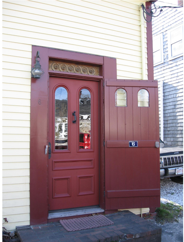
Appropriate building resilience includes protecting the doors and windows at 6 York Street with a storm door (above) and storm windows (below).
