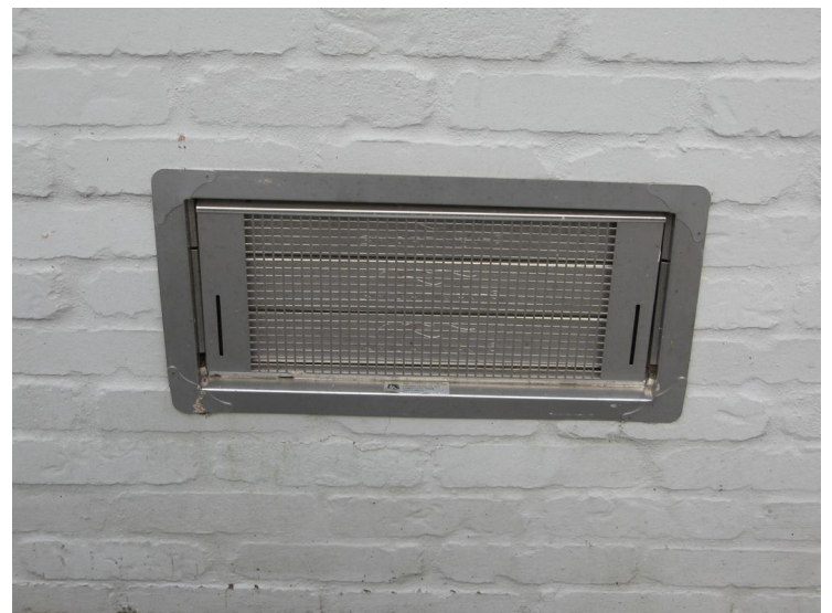
Appropriate flood vents in the brick foundation at 42 Fayette Street (above and below).
