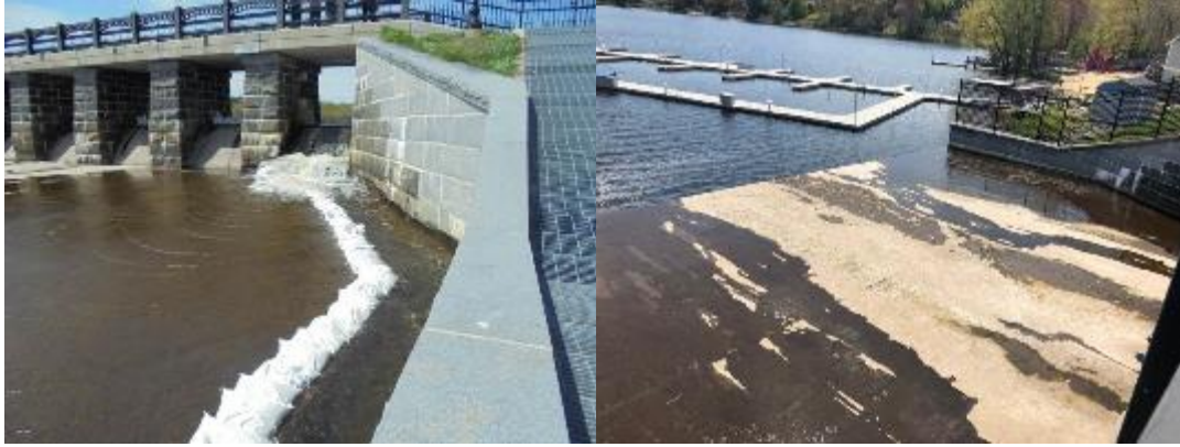
Figure 18. Mystic Lake Dam and Shallow Flow onto Spillway (right image) and Sandbags Used a Temporary Solution to Promote Fish Passage (left image)
