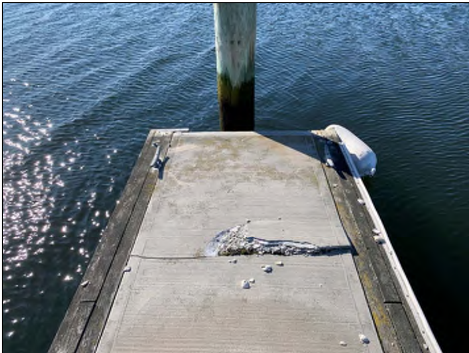
Photo No. 4: Cracking and deterioration of concrete with a trip hazard.
