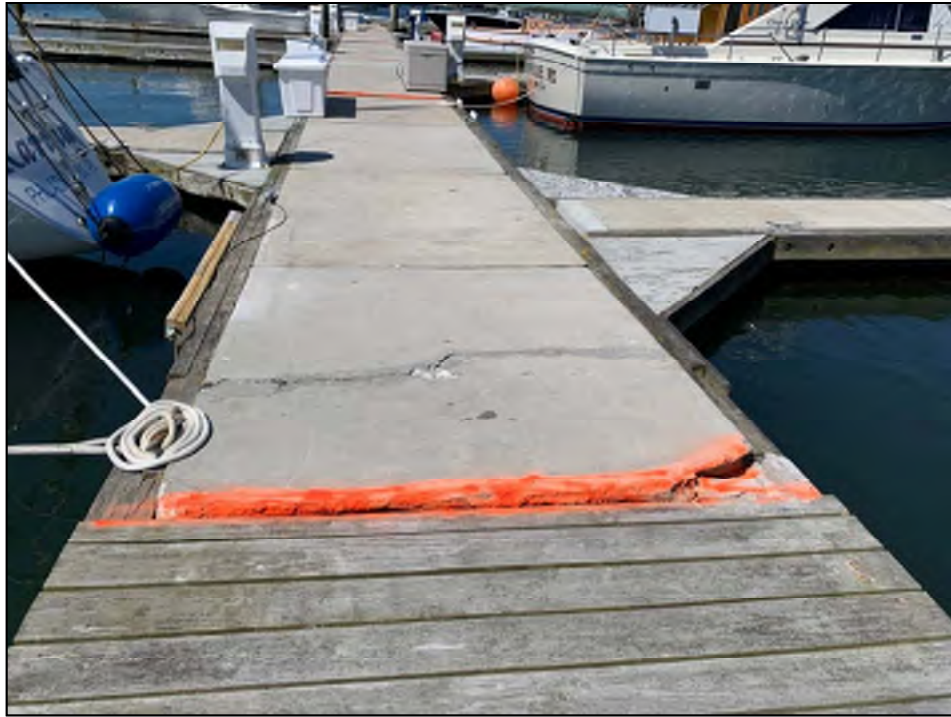
Photo No. 31: Concrete deterioration with trip hazard. Note previously repaired spall with continued deterioration..
