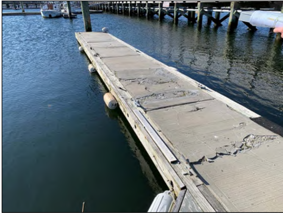
Photo No. 3: Typical spalling, cracking, and deterioration of fiber reinforced concrete modules.
