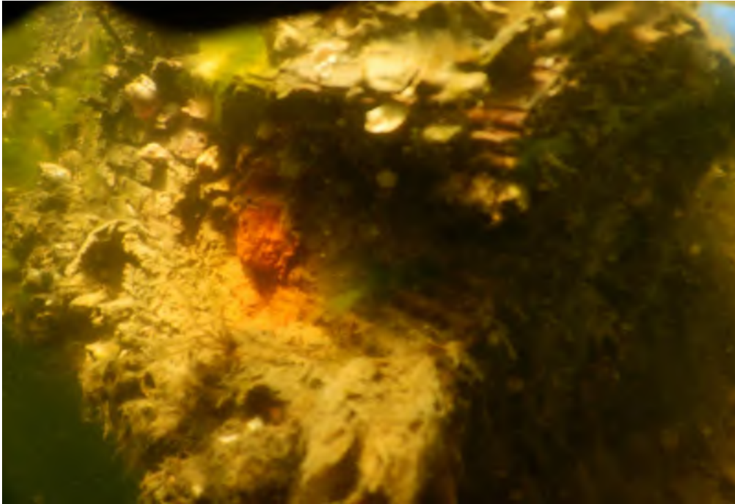
PHOTO #3 Photo of a fractured brace end and deteriorated fastener.
