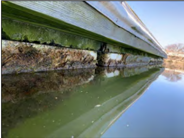
Deterioration of the concrete modules along the waterline.
