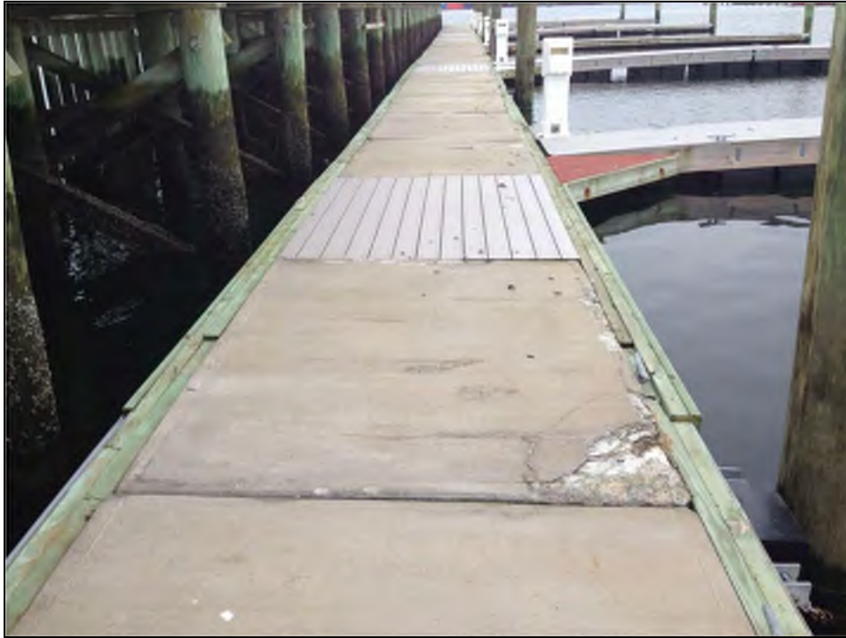
Photo No. 27: Composite decking replacing a concrete deck panel.
