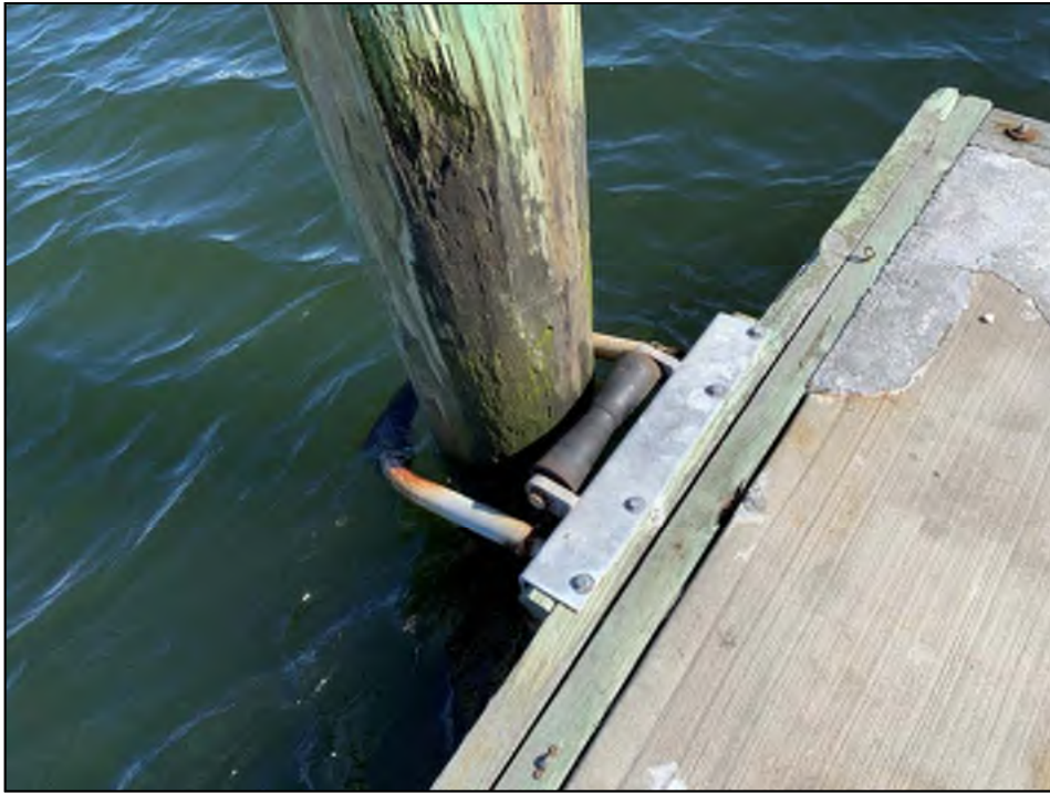
Photo No. 19: Guide pile hoop with loose connection.
