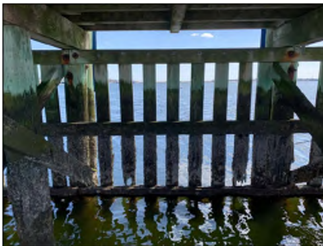
Timber wave fence along T-head of pier
