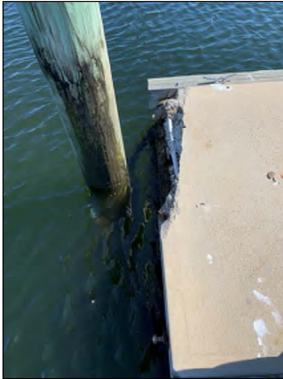
Photo No. 29: Concrete deterioration with exposed polystyrene float unit and steel reinforcement.
