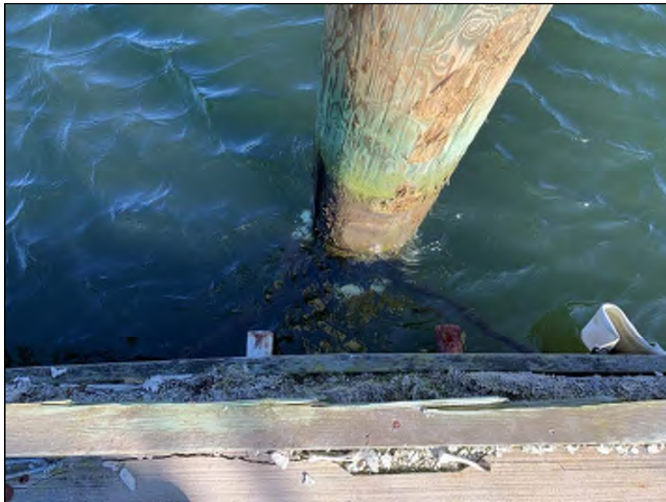
Photo No. 8: Deterioration at end of concrete module with exposed polystyrene flotation unit. Note absence of pile guide and replacement with rope.
