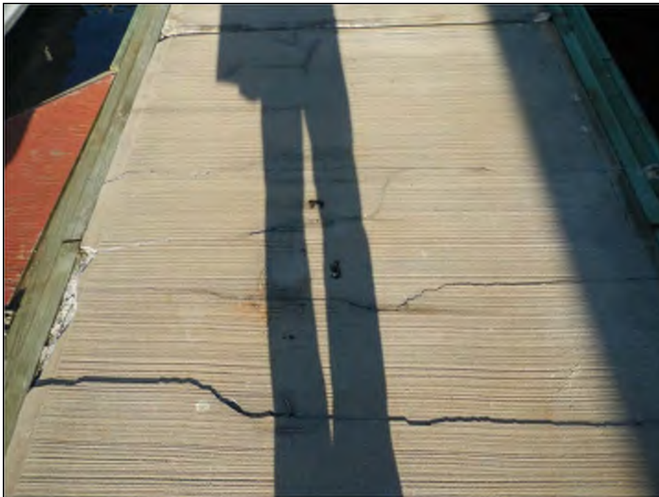
Photo No. 16: Cracking and trip hazards along the concrete deck panels.
