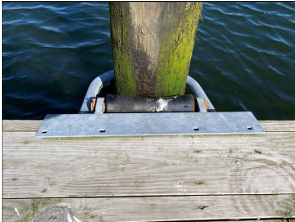
Photo No. 16: Typical top bolts missing on top of steel angle for guide pile.
