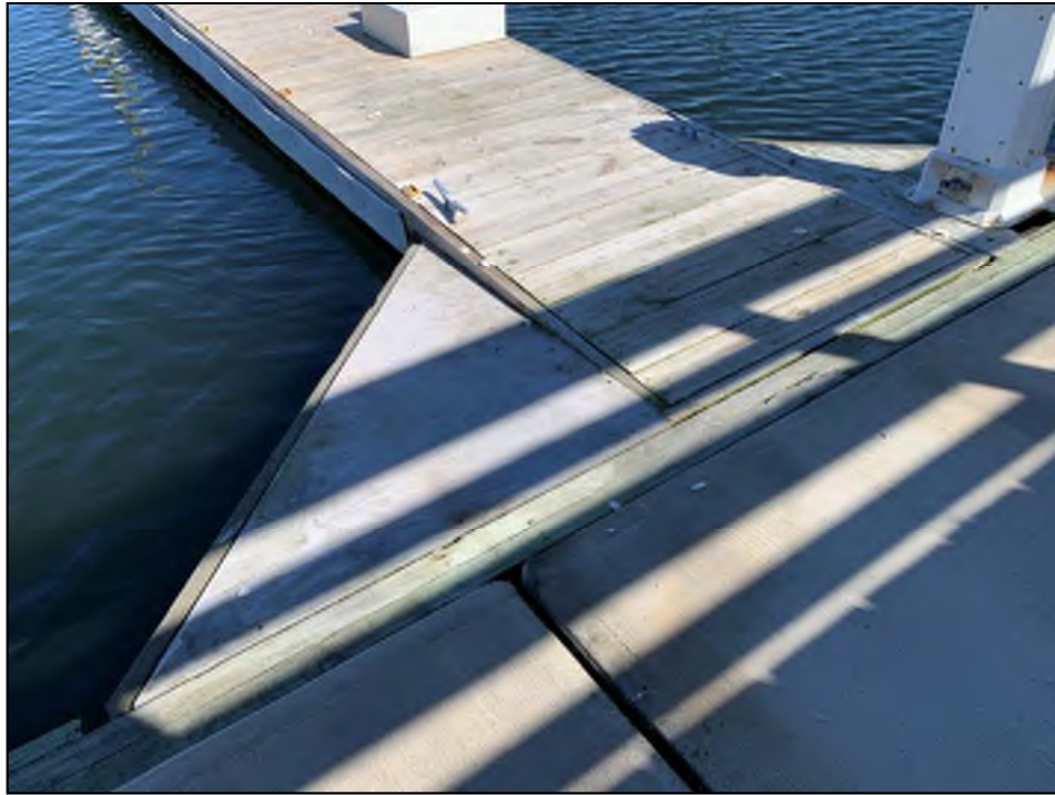
Photo No. 15: Typical uneven timber triangle for finger float connection.
