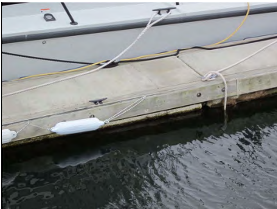
Photo No. 20: Deterioration of the concrete modules with exposed polystyrene at a finger float.
