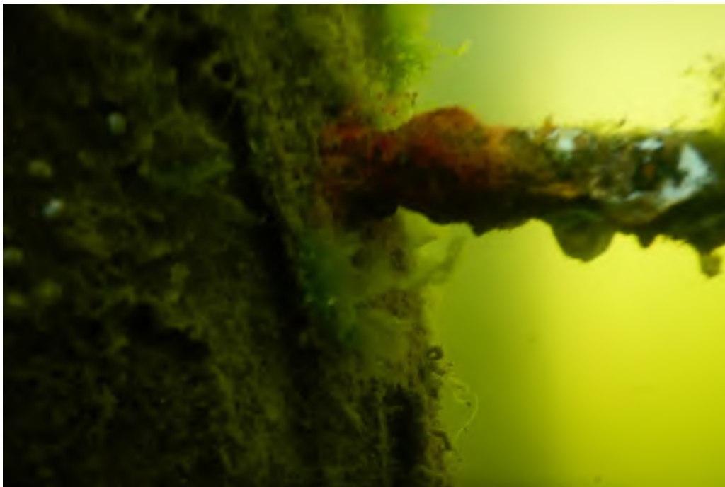
PHOTO #1, This is a typical fastener at low water holding a cross brace.
