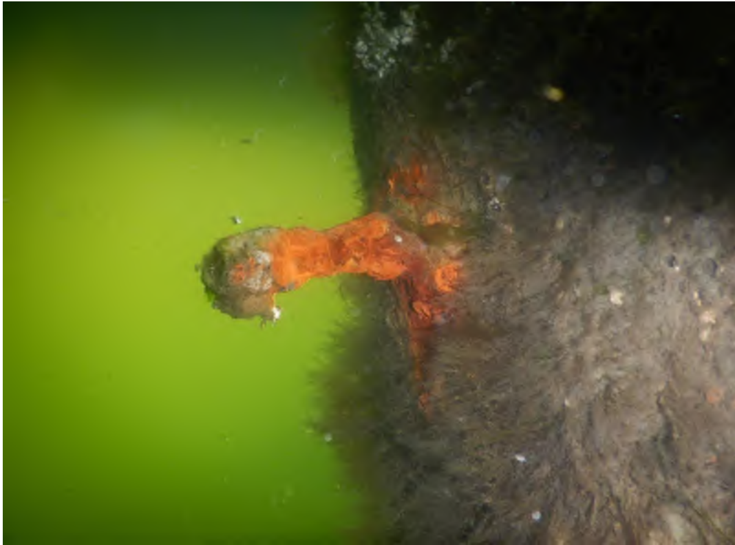
PHOTO #8, typical X brace fastener at low water.
