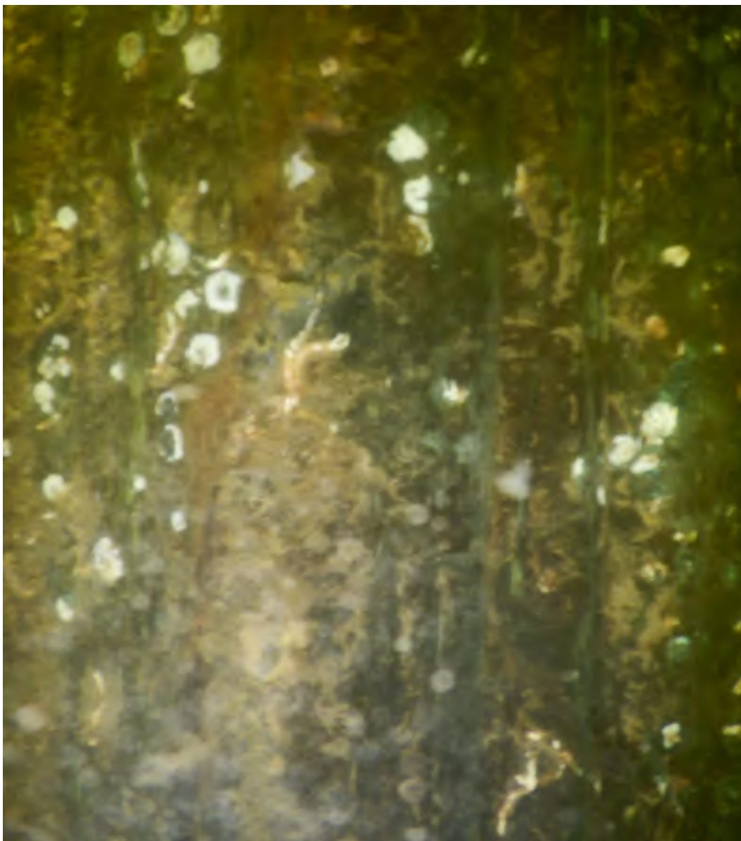
PHOTO #4, Typical pile in the West section. Piles were relatively smooth with some barnacle scars. The vertical scrapes in the picture are from the cleaning tool, the green wood treatment can be seen.
