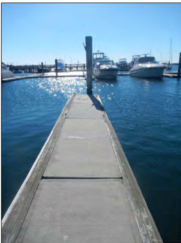
Photo No. 10: Typical view of displaced concrete panels with trip hazards.
