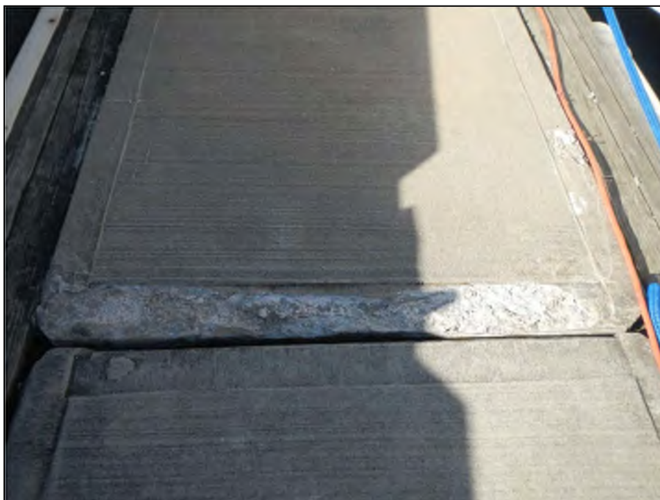
Photo No. 12: Deterioration at the edge of a concrete deck panel with a trip hazard.
