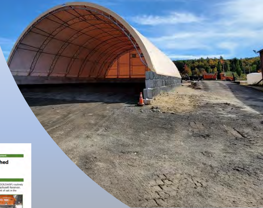
New salt storage building in Princeton
