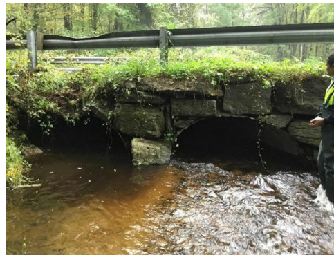
Image 2: View of crossing outlet on September 26, 2018. Note the different flow velocities between the structures.
