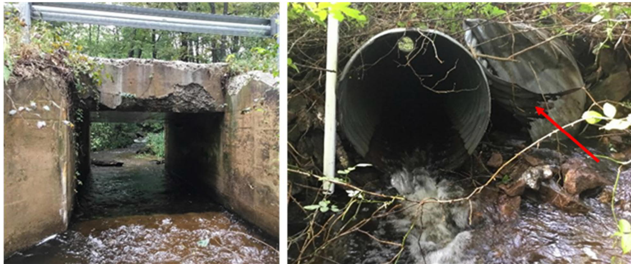
Figure 3. Examples of crossing structures in poor structural condition observed at various locations during field assessments.
