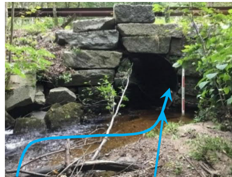
Image 1: View of current structure inlet taken during field assessment on September 21, 2018. Arrows indicate flow paths of Scarboro Brook during low and high flows.
