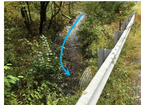
Image 2: Stream alignment relative to culvert inlet. Arrow indicates flow path entering culvert.
