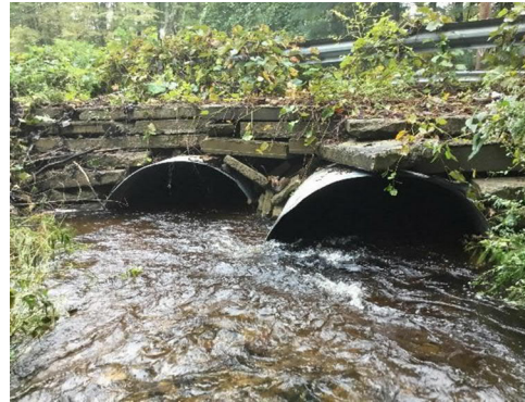
Image 1: View of current crossing inlet taken during field assessment on September 26, 2018. Note deteriorating headwall condition.
