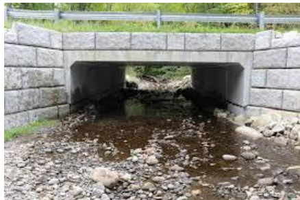
Image 3: Example of embedded box culvert (Maine Audubon).
