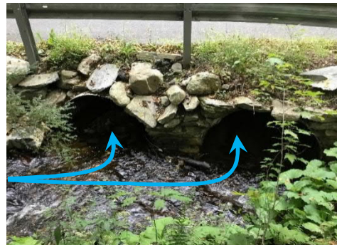
Image 2: View of inlet to middle crossing, September 17, 2018. As indicated by flow arrows, Scarboro takes a near-90-degree turn into the culvert.
