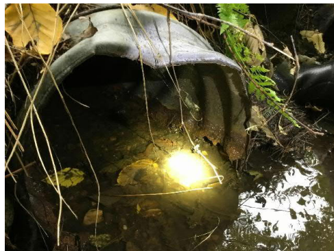
Image 3: View of deteriorated invert condition.
