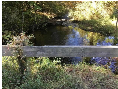
Image 2: Looking downstream from the crossing. Note the width of the scour pool immediately downstream of the crossing relative to the bankfull width of the channel further downstream.
