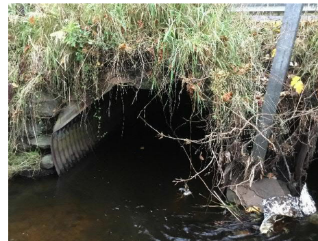
Image 2: Erosion of fill and protective armoring between the two structures at the crossing inlet.
