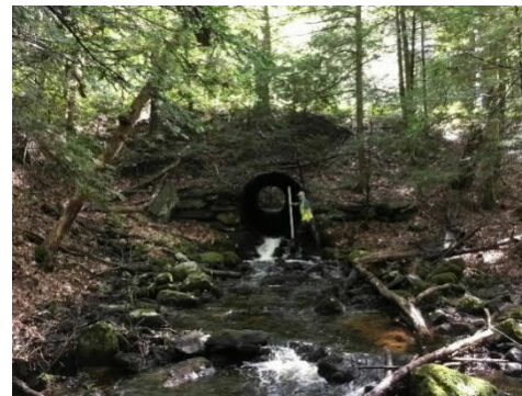
Image 2: View of outlet to middle crossing, September 17, 2018. Note that Scarboro Brook enters from the left of image and takes a near-90 degree turn into the culvert.
