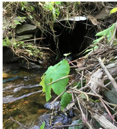
Image 2: View of inlet to current structure. The existing inlet is below the grade of the streambed, creating an inlet drop condition.
