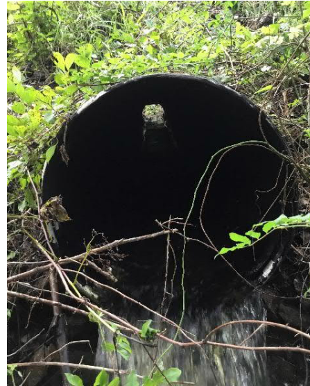
Image 1: View of current structure outlet taken during field assessment on September 27, 2018. Note that outlet has a freefall onto cascade condition which contributes to scour and geomorphic risk.
