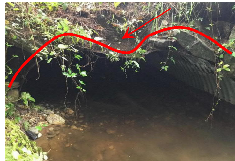
Image 4: View of structure deformation/crushing and poor headwall condition.
