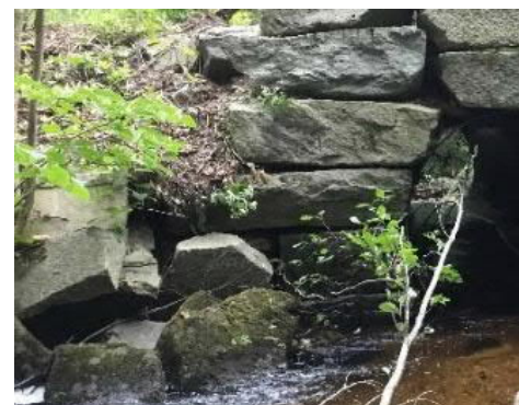
Image 3: Poor headwall condition at inlet.
