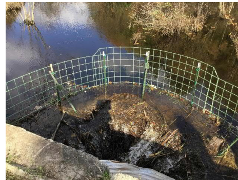
Image 2: View from above looking down on the structure inlet, beaver deceiver, and existing beaver dam/accumulated debris.
