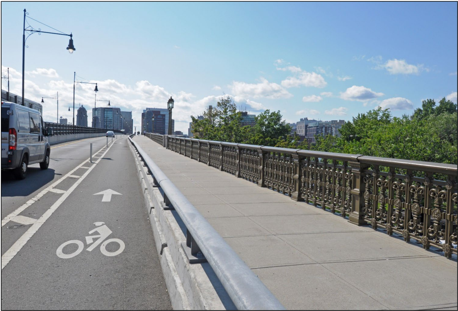
Crash-Tested Barrier with Decorative Barrier at Right
