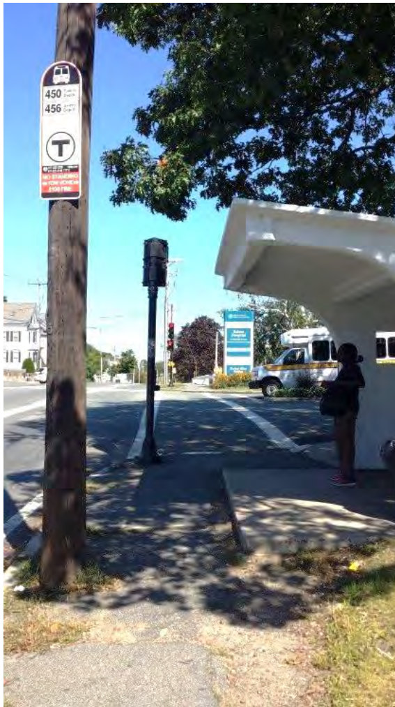
Image III.22: No level path from bus stop to shelter; concrete pad for shelter is raised above the sidewalk.
