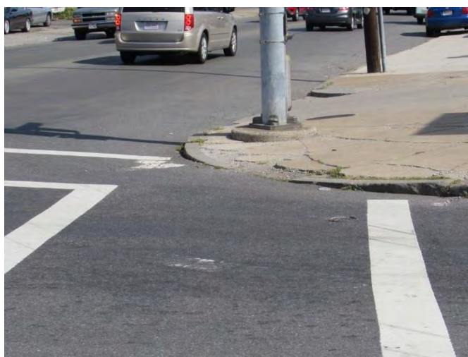
Image III.3: Crumbling curb ramp - eastside, north of Chestnut.
