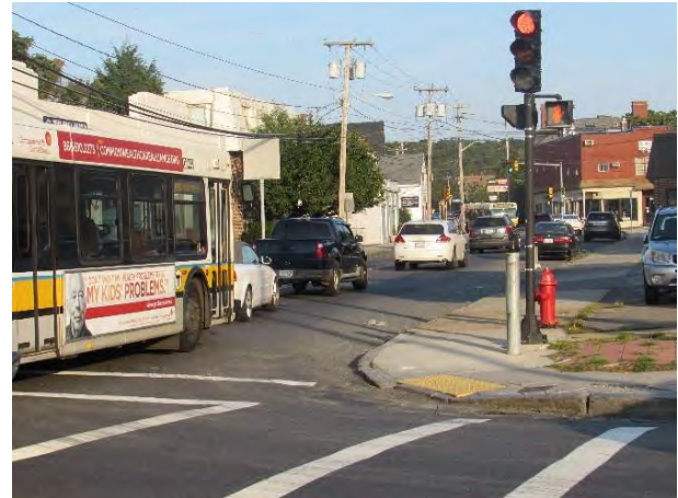
Signal-heads mounted on pedestrian poles.
