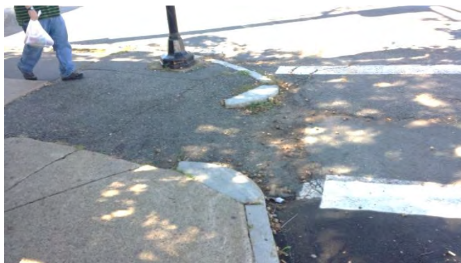
Image III.2: Narrow ramp (3') at entrance to Salem Hospital.
