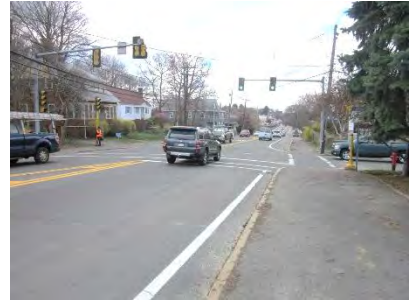
Image III.19: Sign not visible – set too low, on pedestrian signal, set back from curb and obscured by a tree, inbound at Fays.
