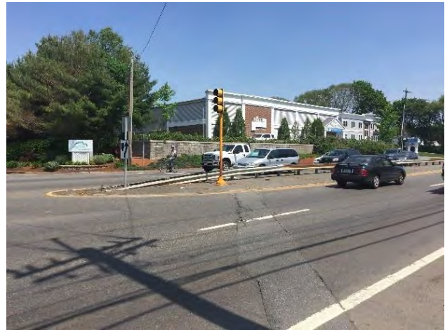
Signal head mounted on a post and unprotected from oncoming traffic by curb or rail.
