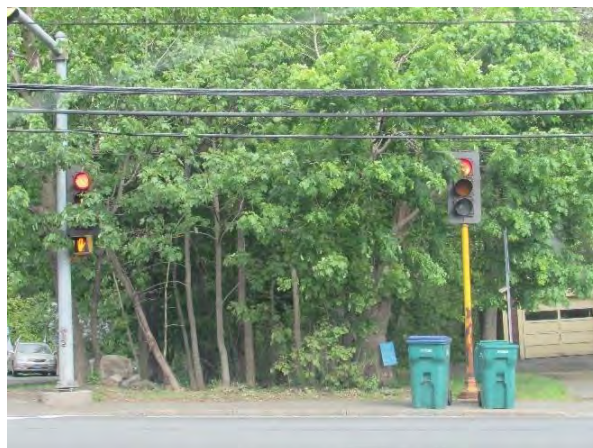
Signal head mounted on a post and blocked by overgrown vegetation.
