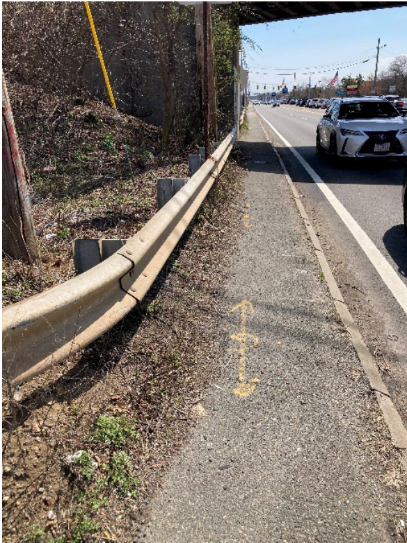
Figure 12. Sidewalk underneath the Danvers Rail Trail Bridge
