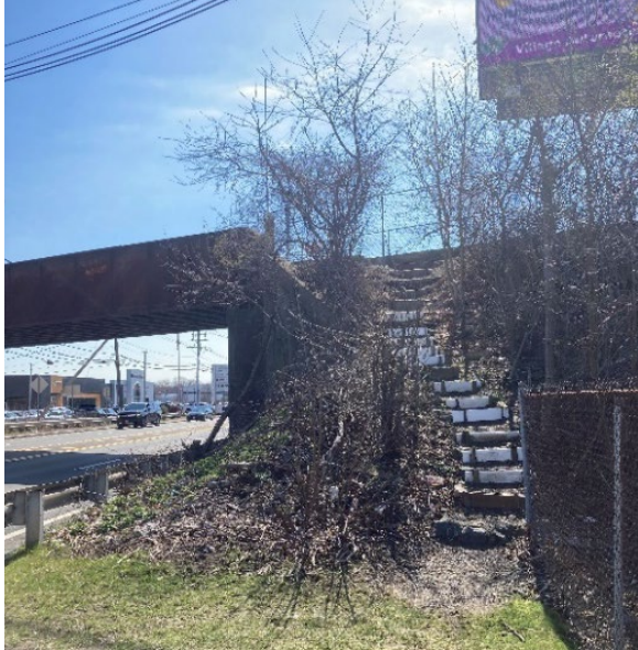
Figure 13. Connection to Danvers Rail Trail from south side of Route 114
