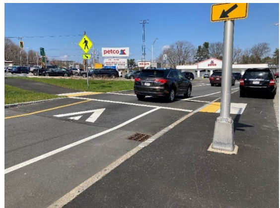
Figure 17. Raised crosswalk across Sylvan Street
