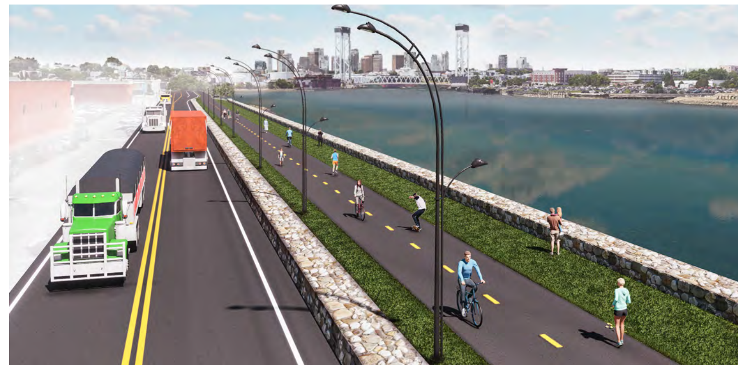
Figure ES-8. Route 1A Along Chelsea Creek – Alternative 2 (Freight Bypass with Shared Use Path)
