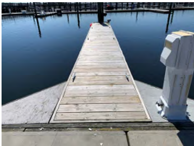
Replacement timber finger float
