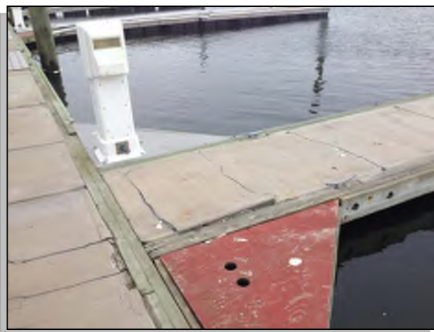
Cracking and displacement of the concrete modules.
