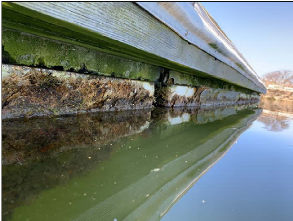
Photo No. 30: Deteriorated concrete encapsulation with exposed polystyrene flotation units.
