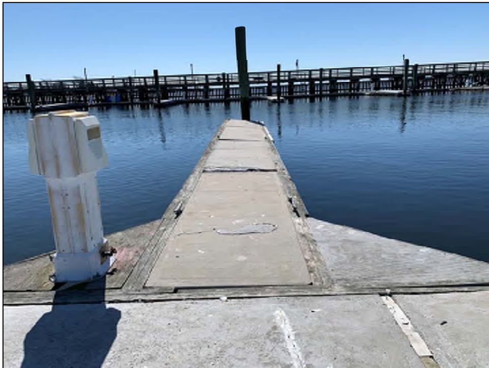
Photo No. 28: Listed and deteriorated concrete float modules with trip hazard.
