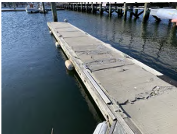
Deteriorated concrete finger float
