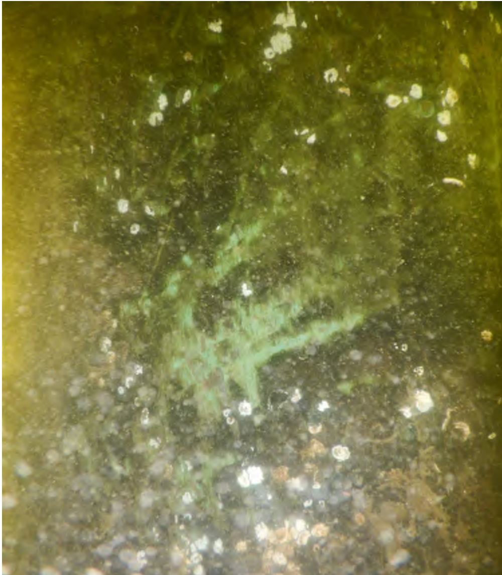
PHOTO #2, This is a photograph of a cleaned pile under the Main Pier. The pile was relatively smooth and undamaged, the green pile treatment can be seen, some barnacle scarring is present.
