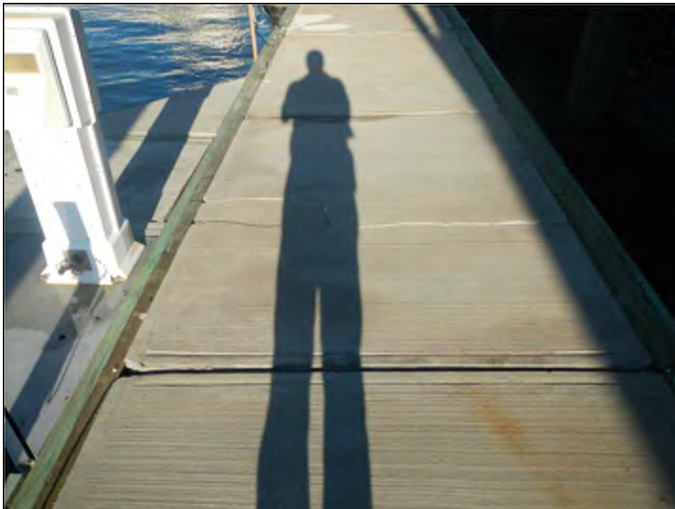
Photo No. 18: Cracking and trip hazards along the concrete deck panels.
