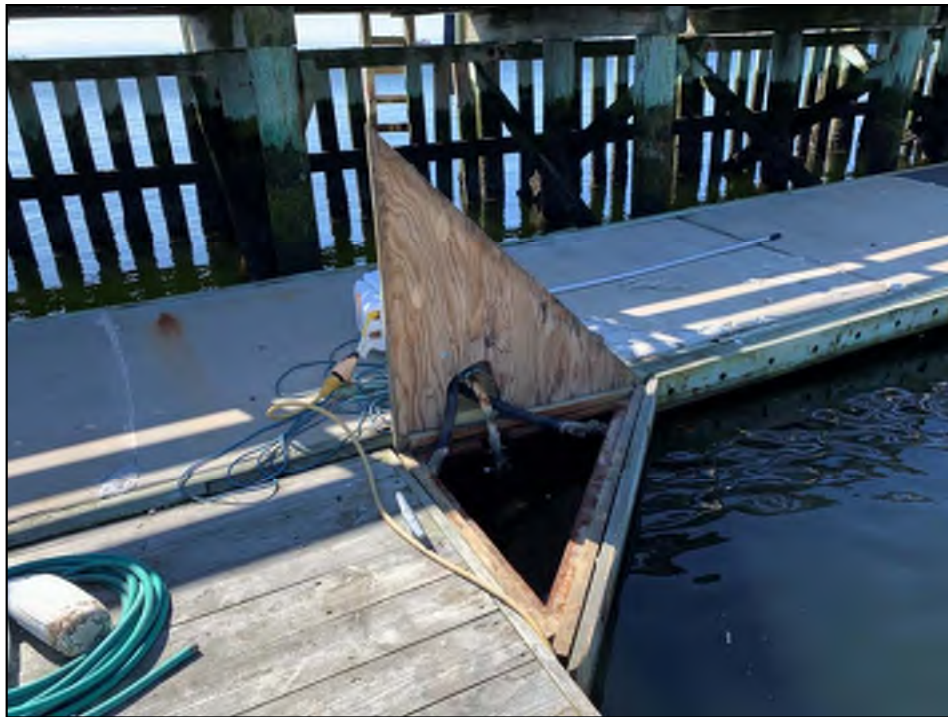
Photo No. 23: Disconnected timber triangle connection and overturned power pedestal.
