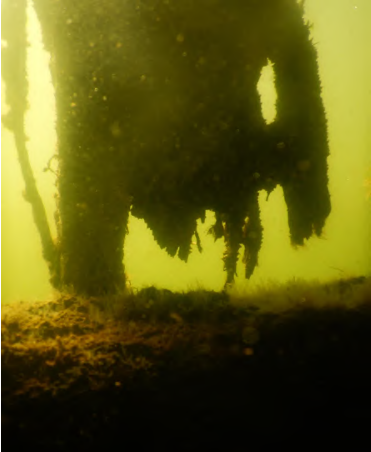
PHOTO #10, showing a wave plank underwater. Many of the planks were in this condition and the whaler-support timber below was rotted and falling down. Low water fasteners holding the planks were poor, fasteners holding the timbers to the piles were poor
