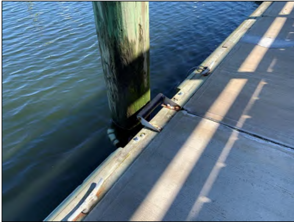
Photo No. 41: Galvanized chain guide with PVC roller.
