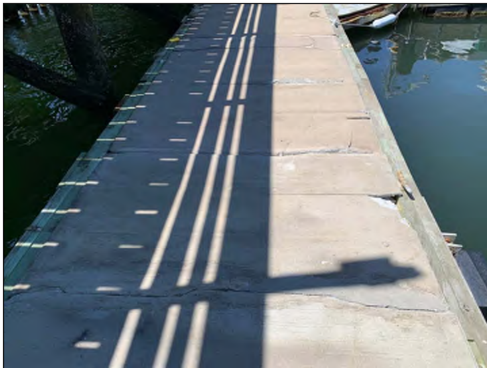
Photo No. 36: Damage to deteriorated concrete main floats on Dock D.
