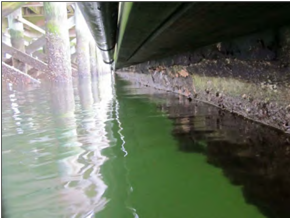
Photo No. 24: Deterioration of the concrete modules near the waterline.
