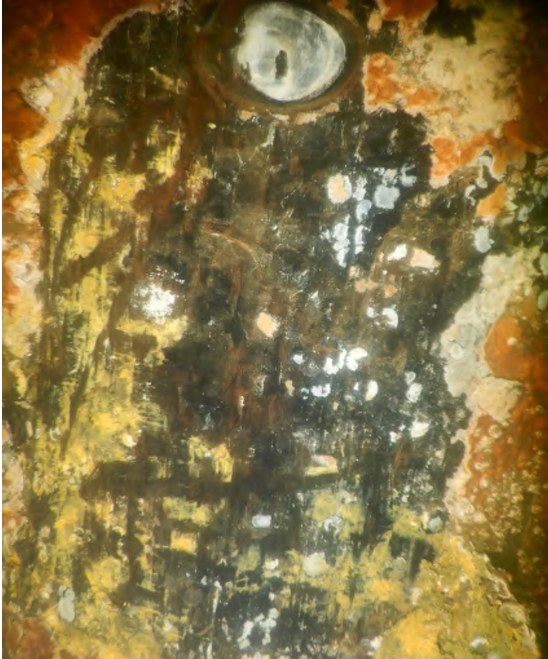
PHOTO #7, showing the surface of a random cleaned pile. The green CCA treatment can be seen, there are barnacle scars on the surface. The pile was hard to a hammer blow and smooth to the touch. The circular area top of photo is a knot in the wooden pile. The knot was not deteriorated and the wood sound. The different colored lines are from the scraping-cleaning process.
