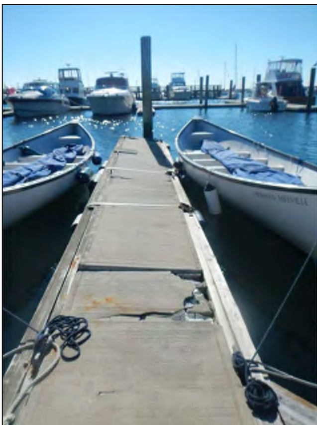
Photo No. 9: Listed finger float with displaced concrete panel creating a trip hazard.
