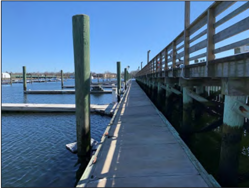
Photo No. 13: Listing of float units along majority of main floats at Dock B.
