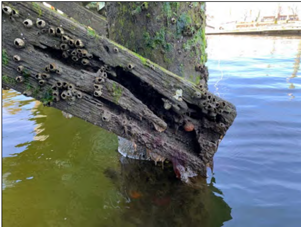
Photo No. 42: Timber cross bracing with up to 90% section loss typical along pile supported pier.
