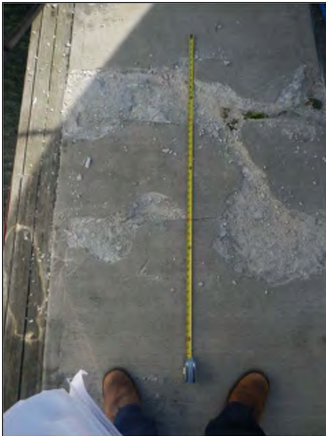
Photo No. 13: Typical trip hazard at the joints between adjacent concrete modules along the main floats.
