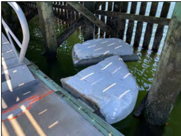
Displaced polystyrene float units after seasonal storm
