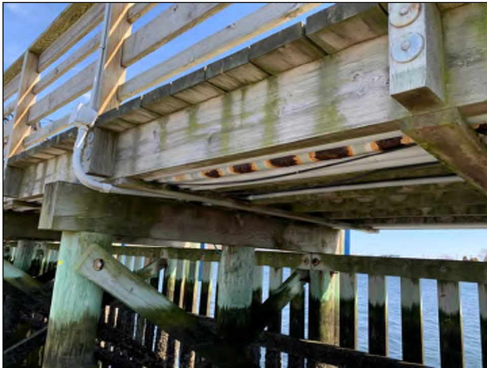
Photo No. 48: Corroded fire line along T-head.
