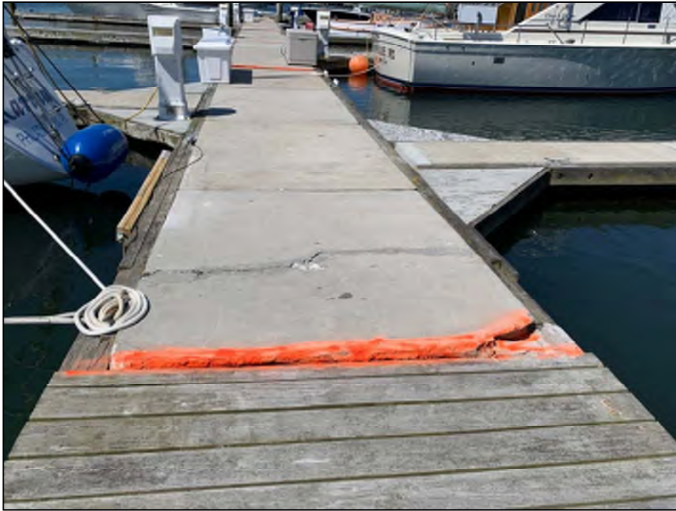
Photo No. 31: Concrete deterioration with trip hazard. Note previously repaired spill with continued deterioration..
