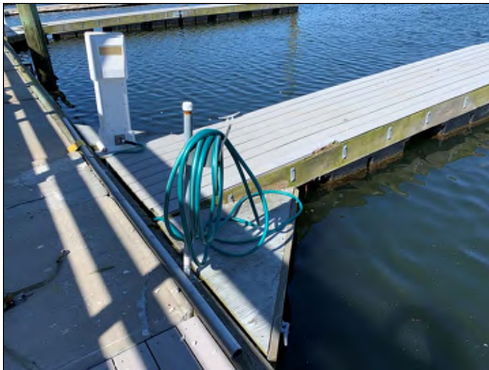
Photo No. 24: Failing timber triangle connection.
