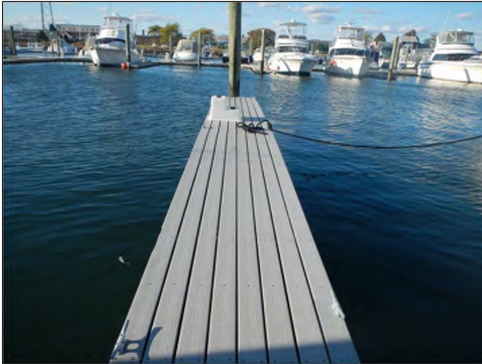
Photo No. 25: New timber float with composite decking.
