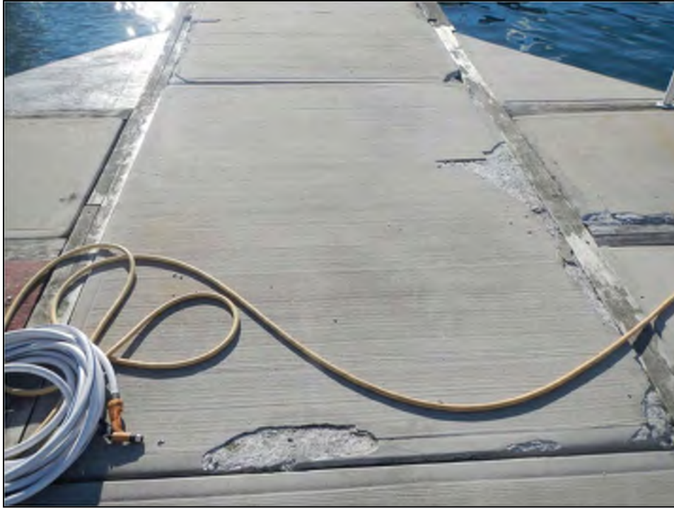
Photo No. 15: Deterioration of the edges of the concrete deck panels creating trip hazards.
