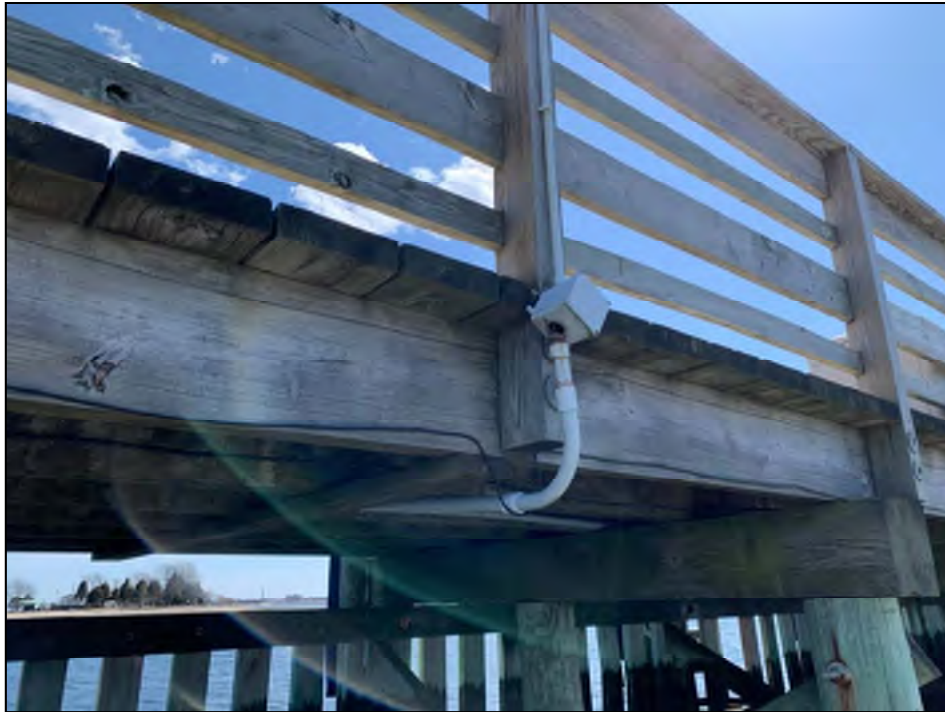
Photo No. 47: Dislocated conduit from light box at T-head.
