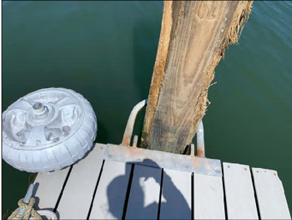
Photo No. 39: Timber pile damage from missing roller after storm.
