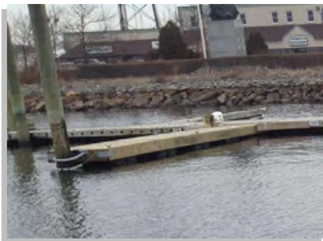
New timber replacement float.
