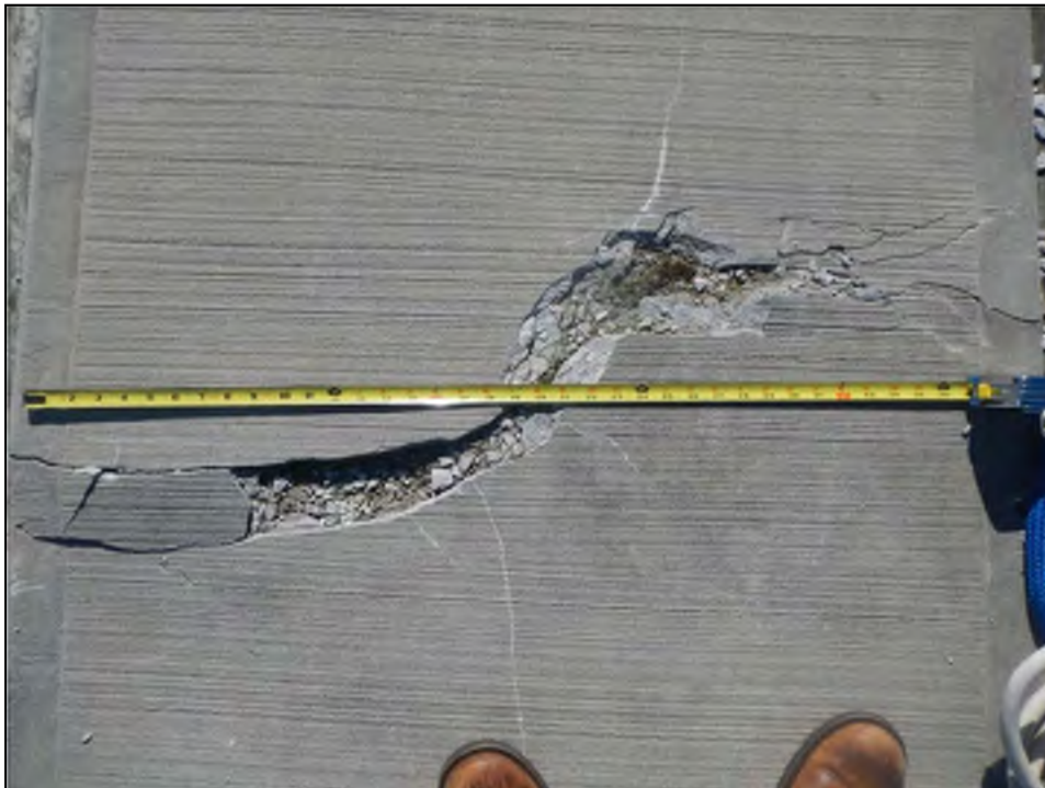
Photo No. 8: Cracking and deterioration of the concrete deck.
