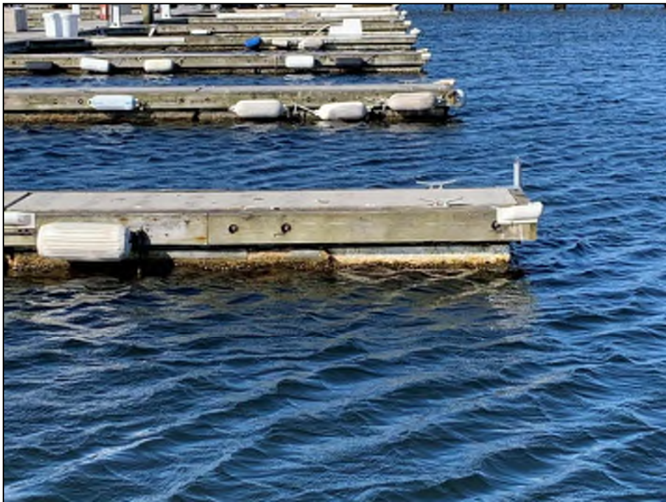
Photo No. 6: Deteriorated concrete encapsulation with exposed polystyrene flotation units.
