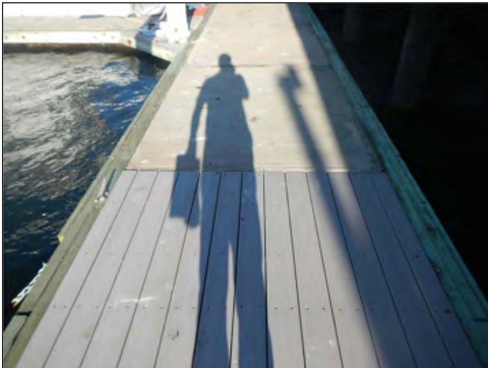
Photo No. 26: Composite decking replacing a concrete deck panel.
