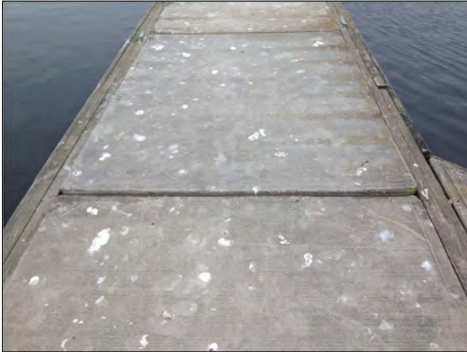
Photo No. 13: Typical trip hazard at the joints between adjacent concrete modules along the main floats.
