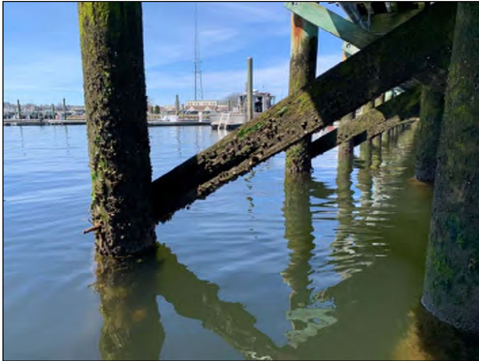
Photo No. 43: Deteriorated cross bracing hardware typical along pile supported pier.
