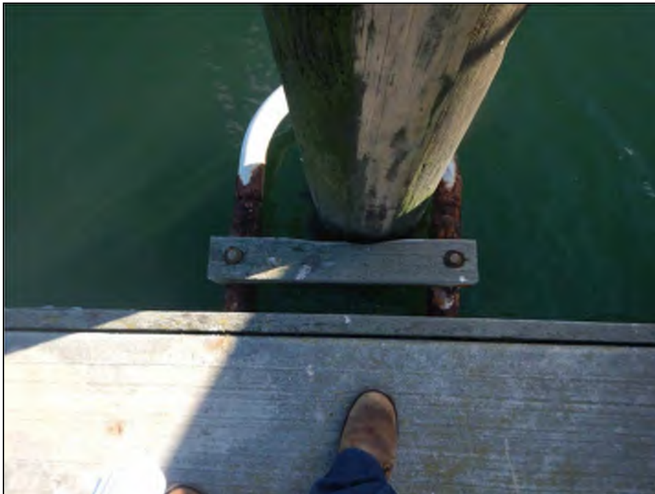
Photo No. 30: Significantly deteriorated steel pile hoop.
