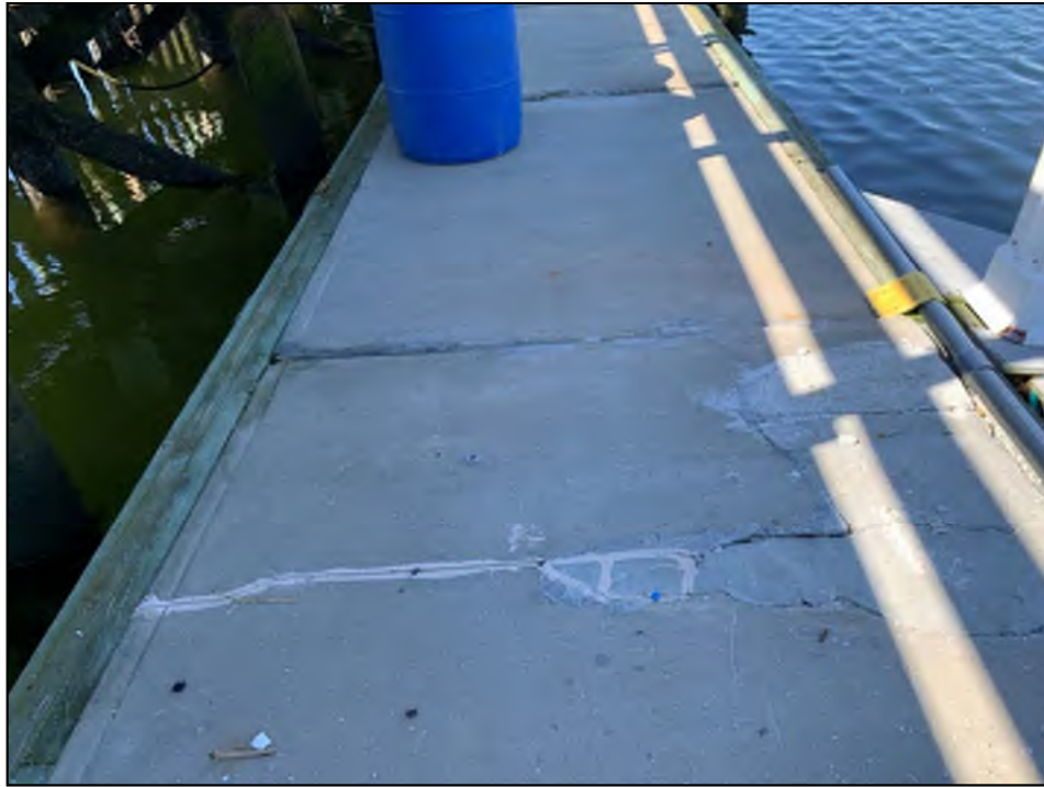
Photo No. 25: Previously repaired spill with trip hazard.
