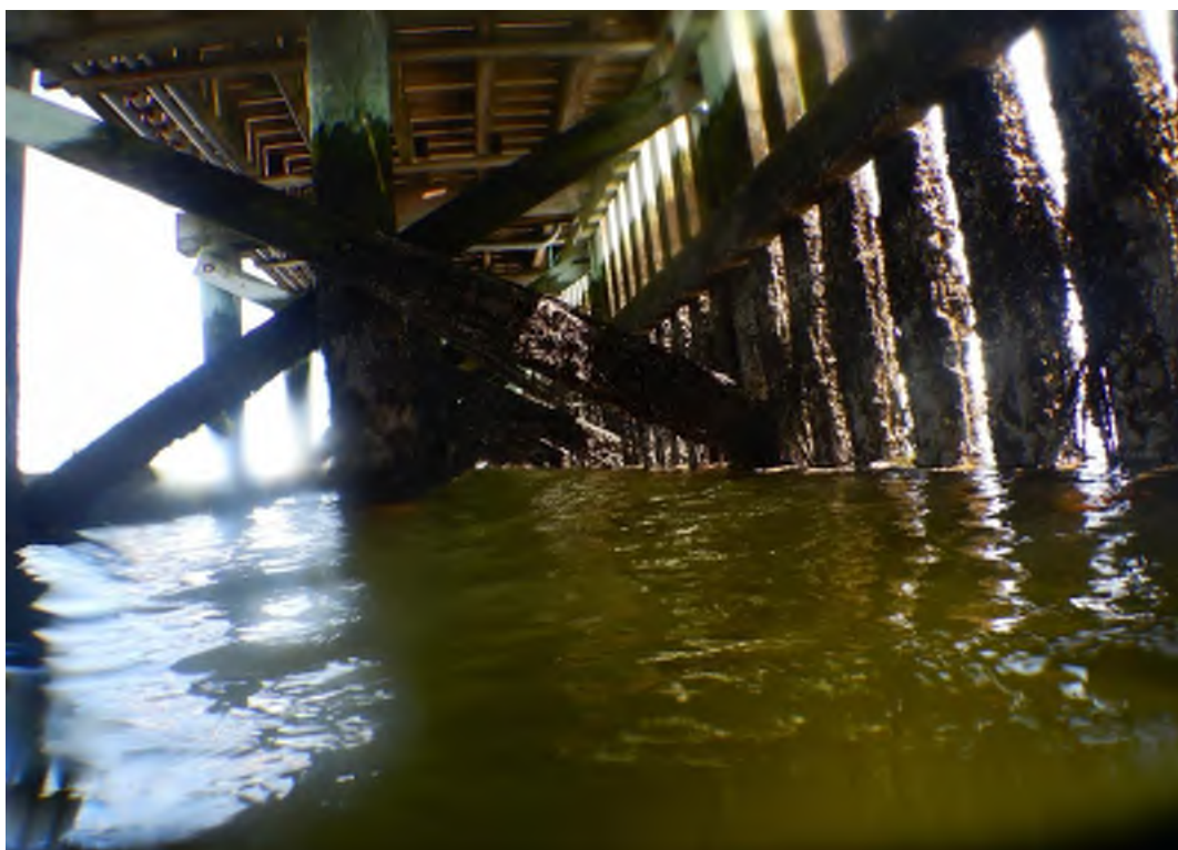
PHOTO #9, taken at low tide. Note the splintered braces at low water and splintered wave barrier blanks
