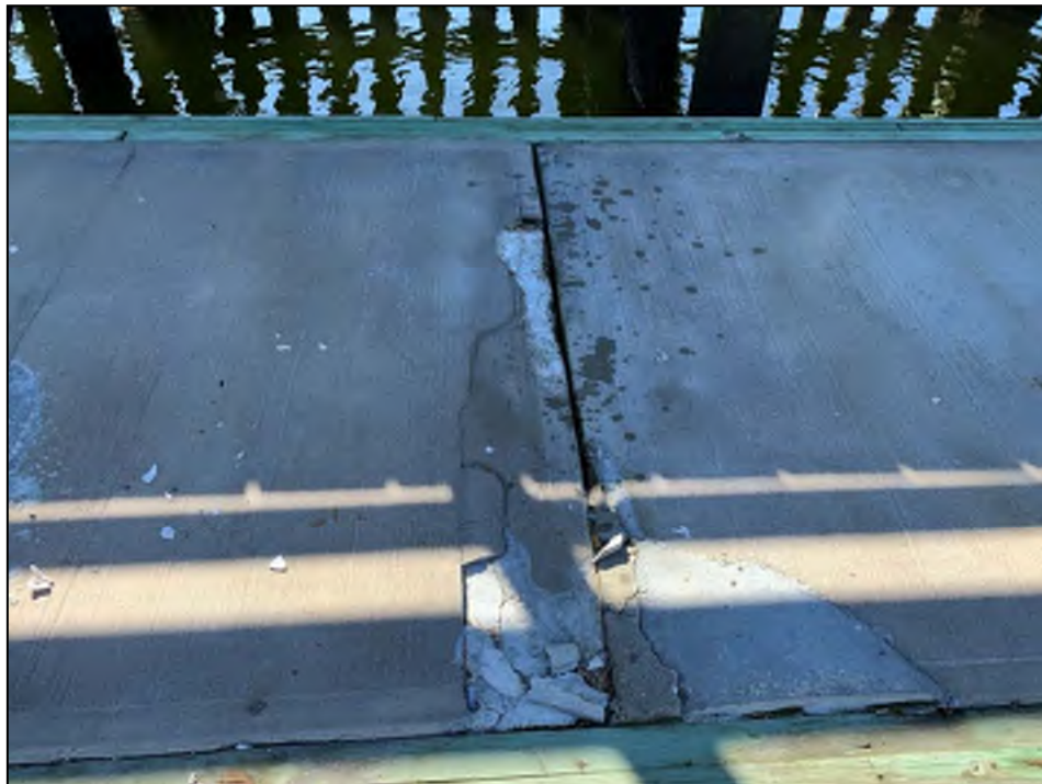
Photo No. 18: Cracking and deterioration of concrete deck with trip hazard and exposed polystyrene float unit. Note deterioration of previously repaired spall.
