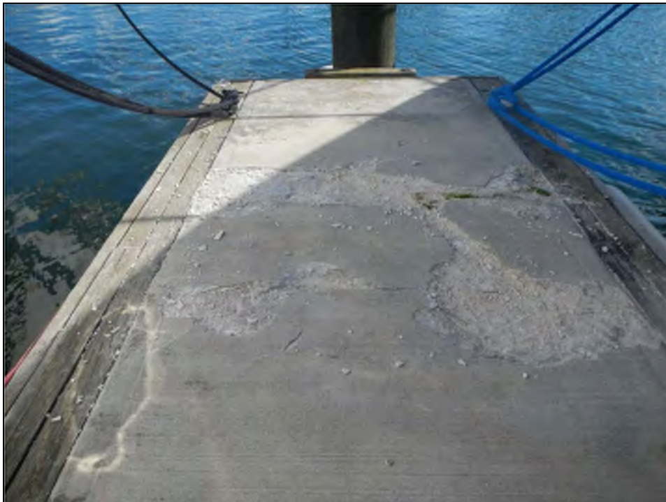
Photo No. 2: Typical spalling, cracking, and deterioration of the fiber reinforced concrete modules.
