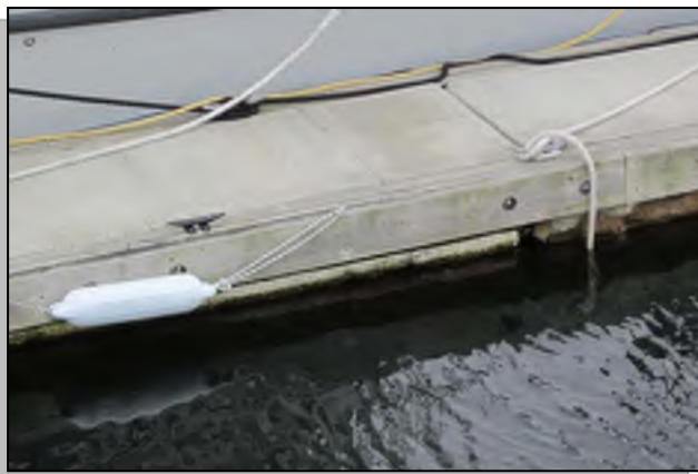
Deterioration of the concrete modules along the waterline.
