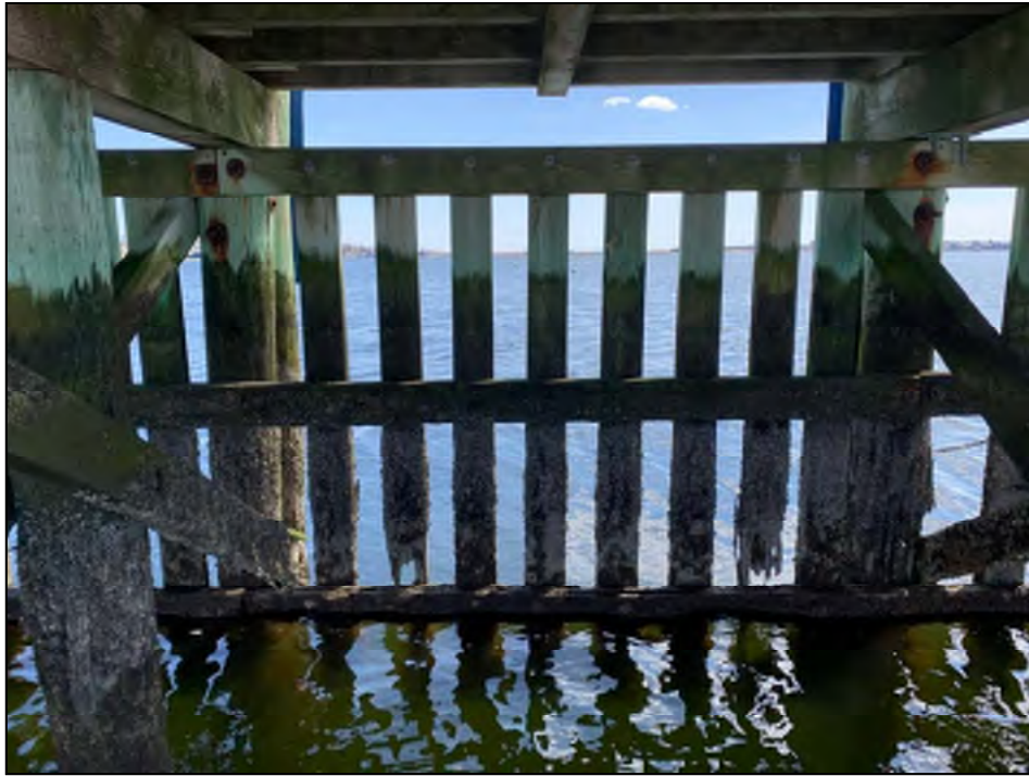
Photo No. 45: Deteriorated timber wave fence.
