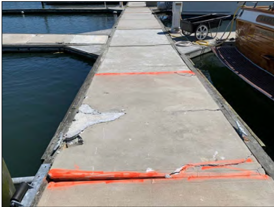
Photo No. 35: Additional damage to concrete after storm.
