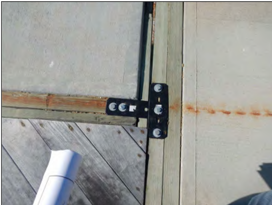
Photo No. 28: Steel plate float connection bolted to timber edge boards.
