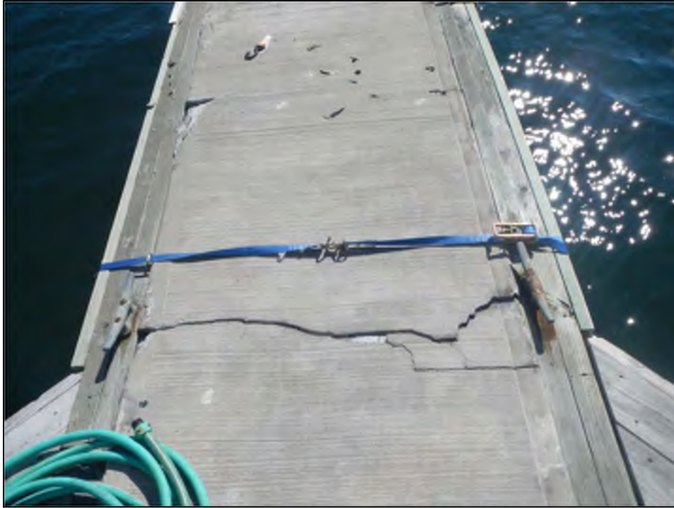
Photo No. 7: Cracking and deterioration of the concrete deck with a trip hazard.
