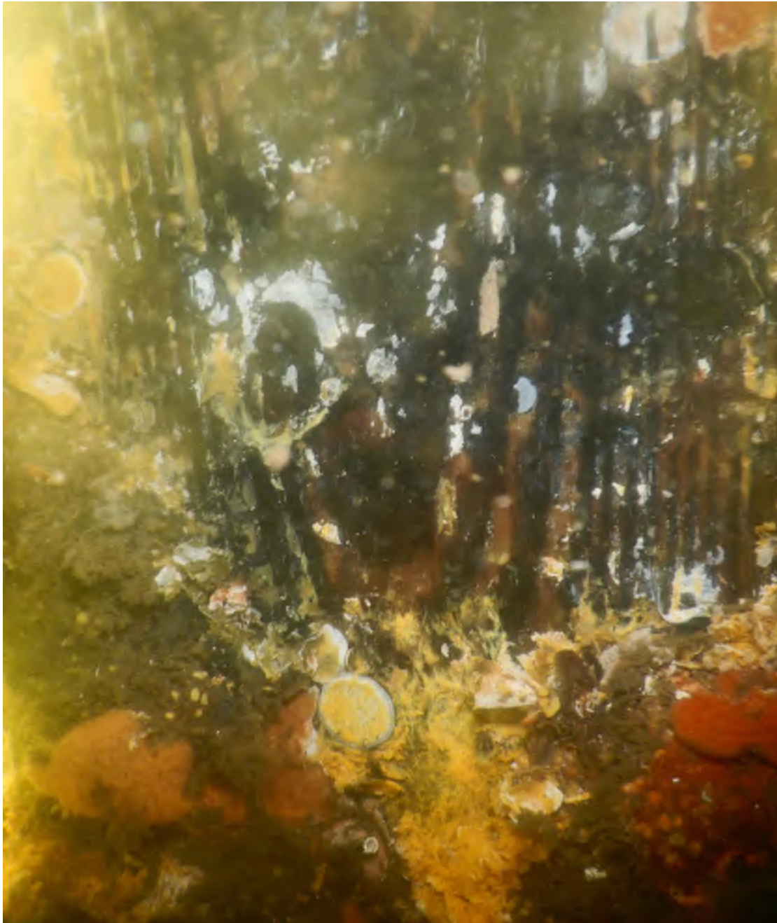
PHOTO #5, Another picture of a pile in the West section of the Marina, the camera gives a close-up view. The wood was hard and smooth to the touch, there is some superficial marine organism damage on the surface of the pile. The circular area mid photo is a "knot" in the wood, which was intact.
