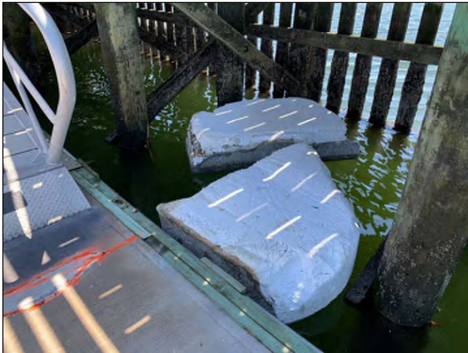
Photo No. 40: Displaced polystyrene float units after storm on Dock D.
