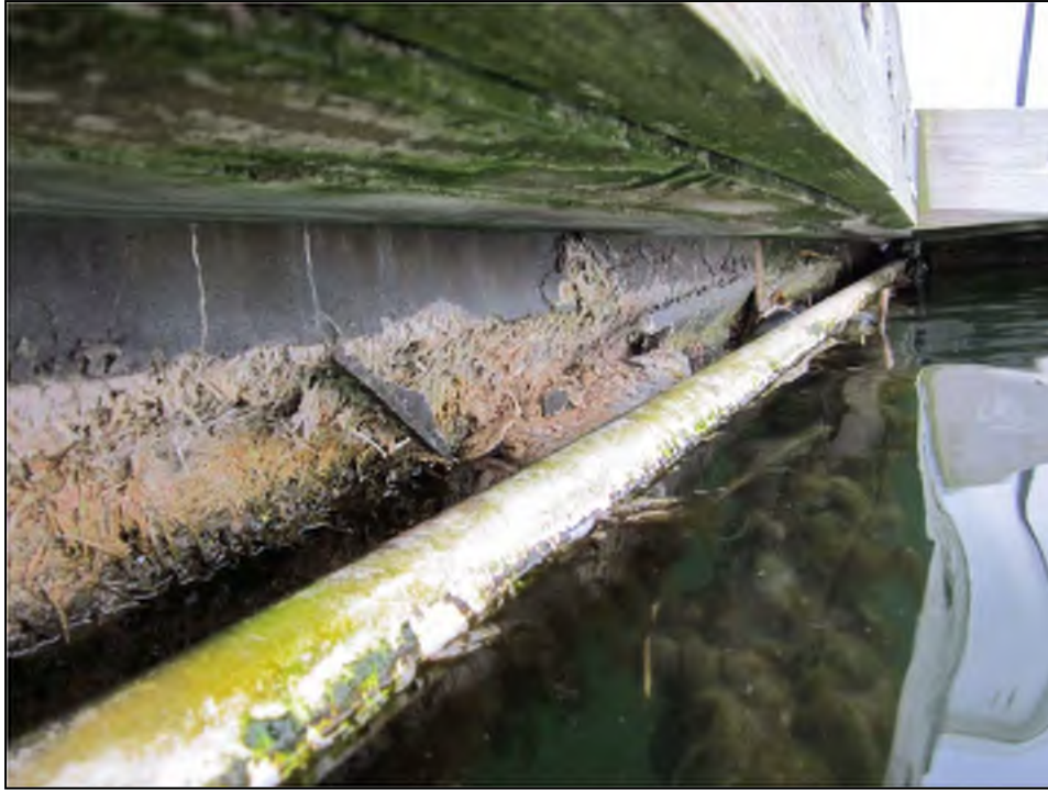
Photo No. 23: Deterioration of the concrete modules near the waterline. Note fiber reinforcement.
