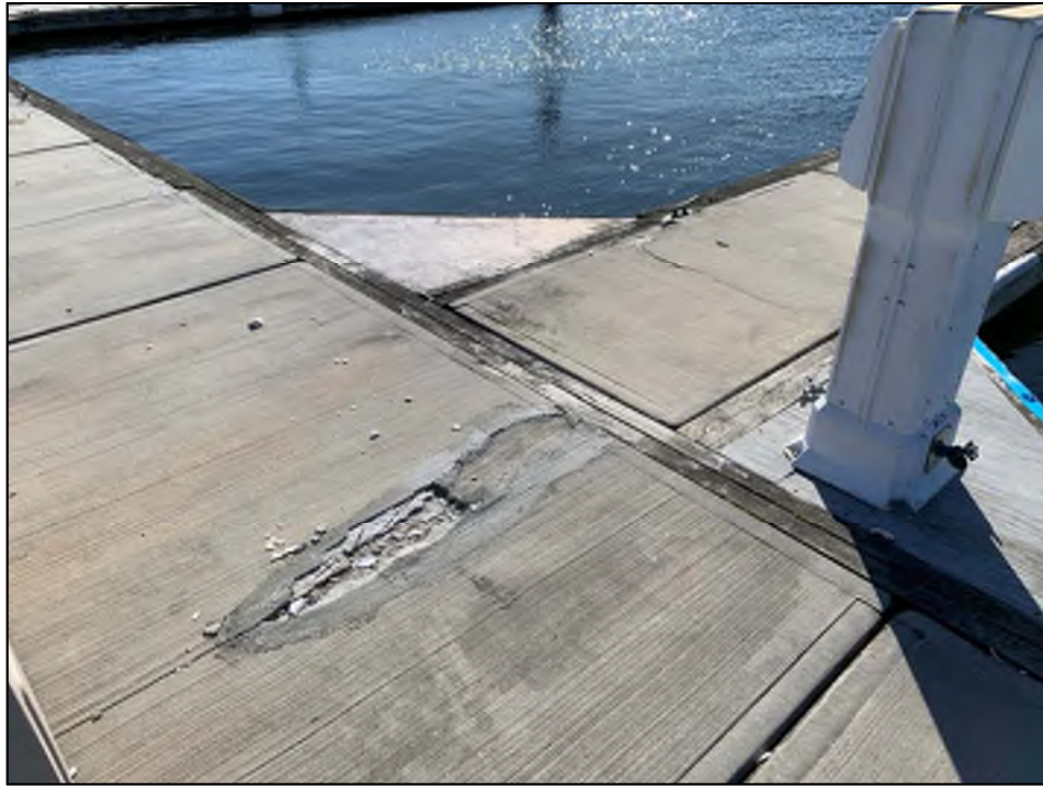
Photo No. 5: Typical deterioration of previously repaired spill
