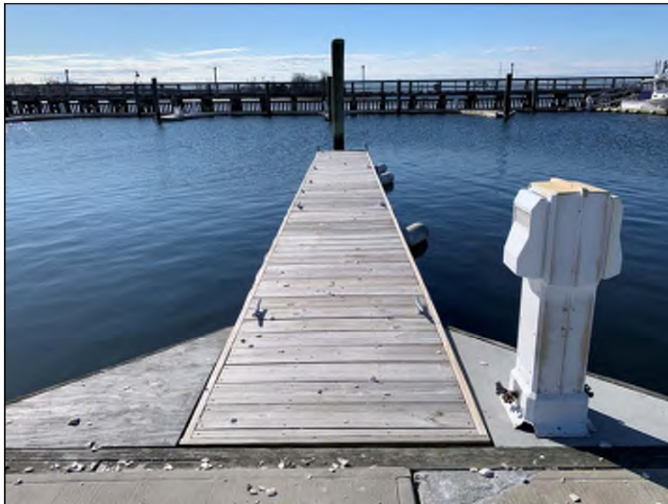
Photo No. 10: Replacement timber finger float.
