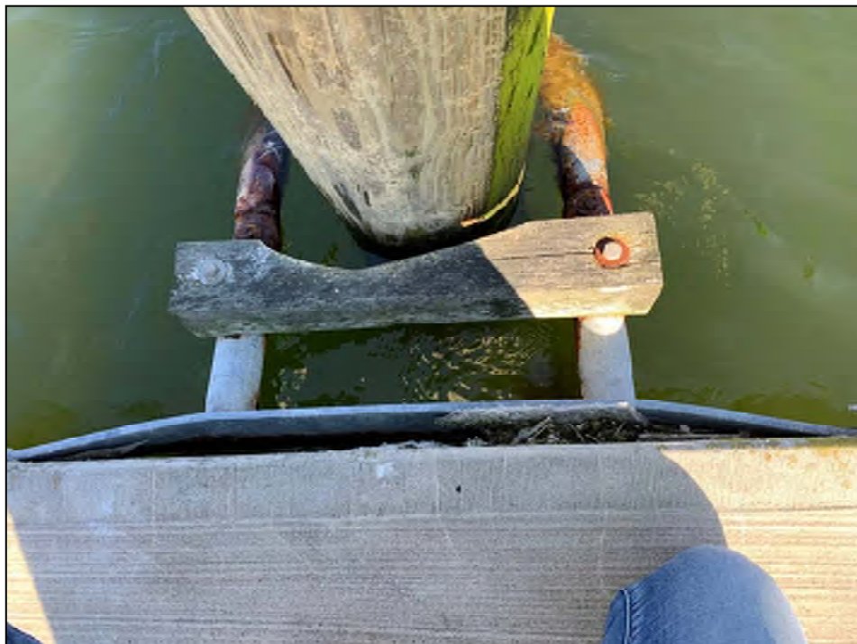
Photo No. 12: Deterioration at end of concrete module with exposed polystyrene flotation unit. Note displacement of pile guide hardware.
