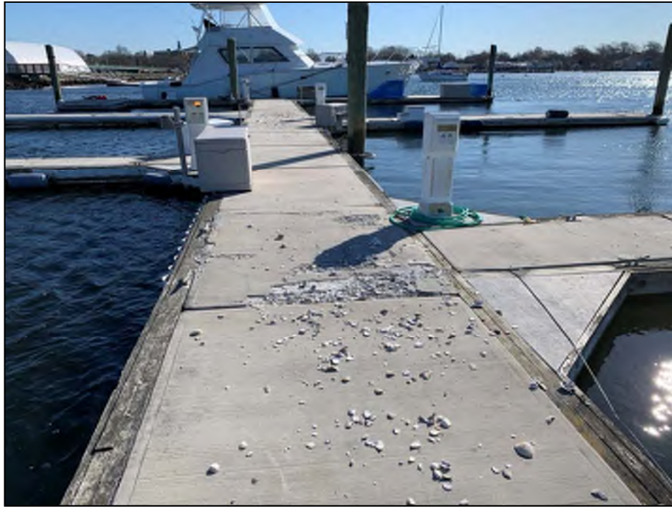
Photo No. 7: Cracking and deterioration of concrete deck with trip hazard.
