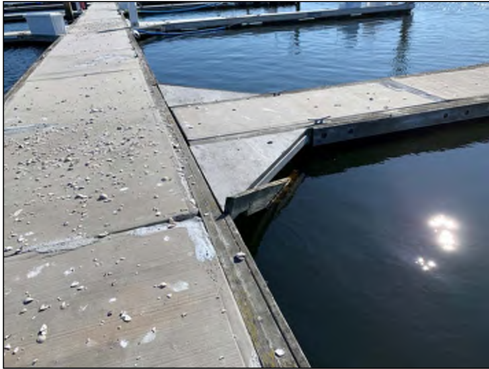
Photo No. 11: Displaced timber skirt board at Dock B.
