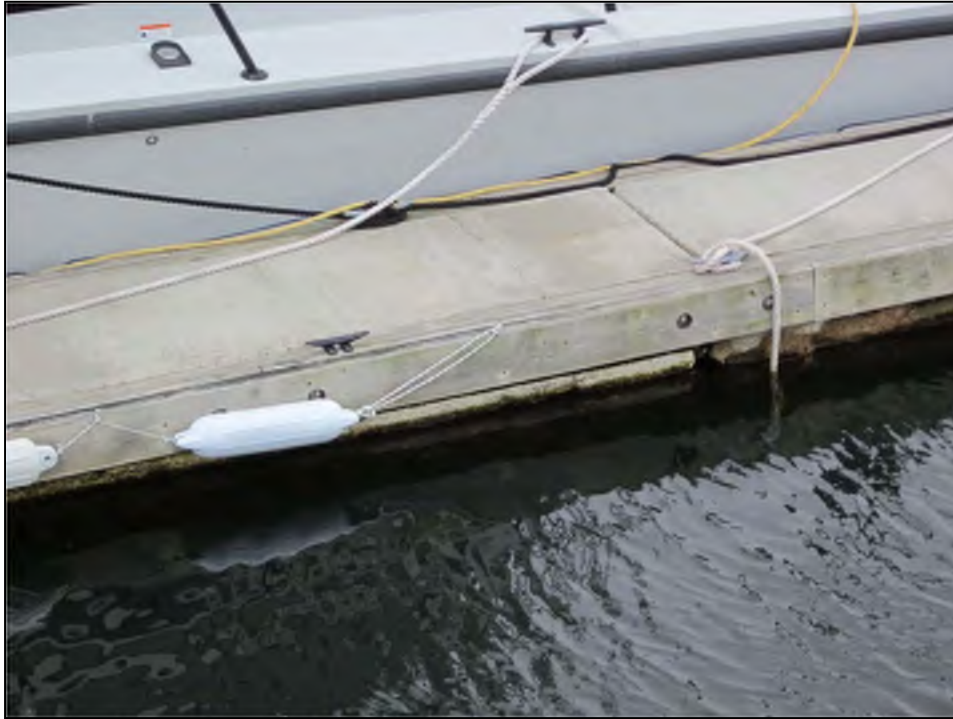
Photo No. 1: Deteriorated concrete encapsulation with exposed polystyrene floatation units.
