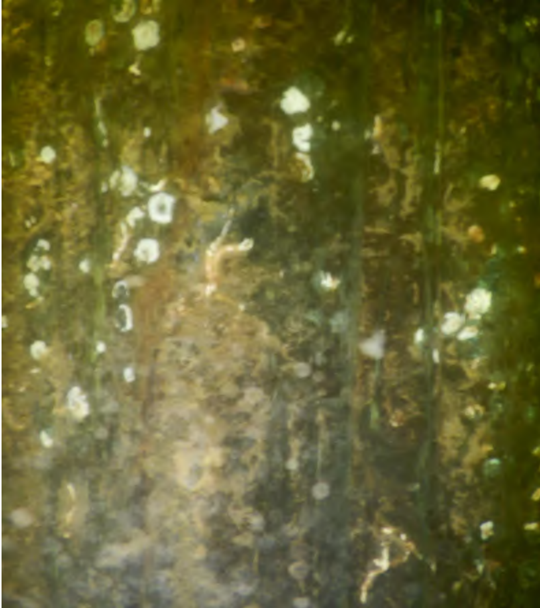
PHOTO #4, Typical pile in the West section. Piles were relatively smooth with some barnacle scars. The vertical scrapes in the picture are from the cleaning tool, the green wood treatment can be seen.
