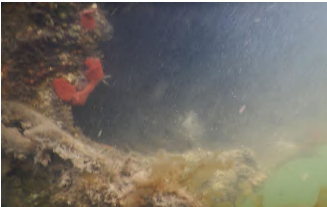
PHOTO #11, showing the deteriorated end of a float with the interior visible, many of the floats in this area were like this.
