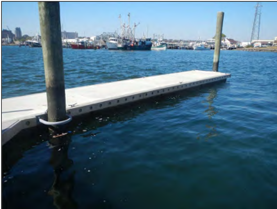
Photo No. 4: New concrete float at the end of F-dock.
