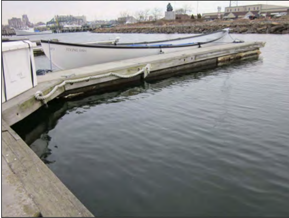
Photo No. 21: Deterioration of the concrete modules with exposed polystyrene at a finger float.
