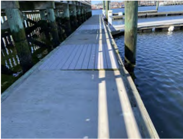
Main float modules replaced with timber/composite floats with tripping hazard
