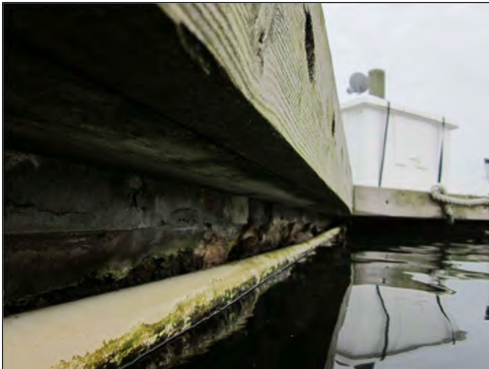
Photo No. 22: Deterioration of the concrete modules near the waterline.
