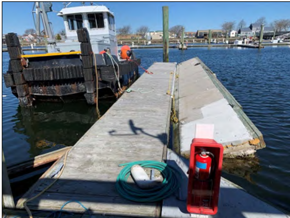
Photo No. 22: New timber finger float with abandoned concrete finger float at Dock D.
