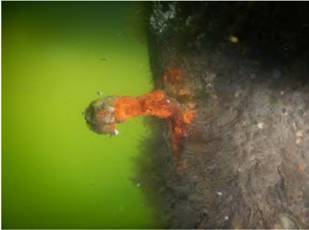
Photo No. 51: Bottom cross bracing hardware below water.
