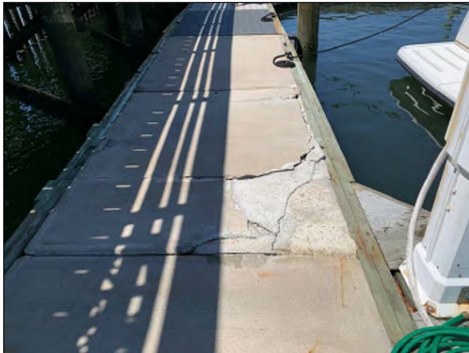
Photo No. 38: Deteriorated concrete main float along Dock D after storm with additional damage and trip hazard.
