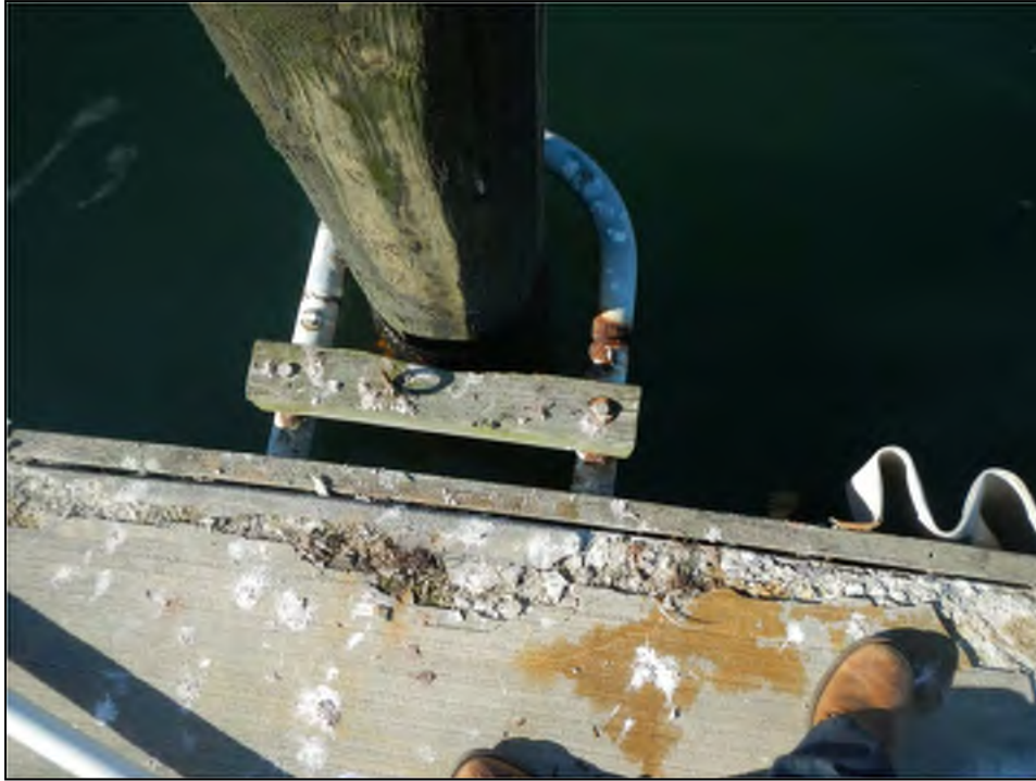
Photo No. 29: Typical existing pile hoop. Note corroded connection hardware.
