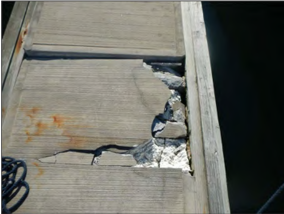
Photo No. 11: Concrete deck deterioration.
