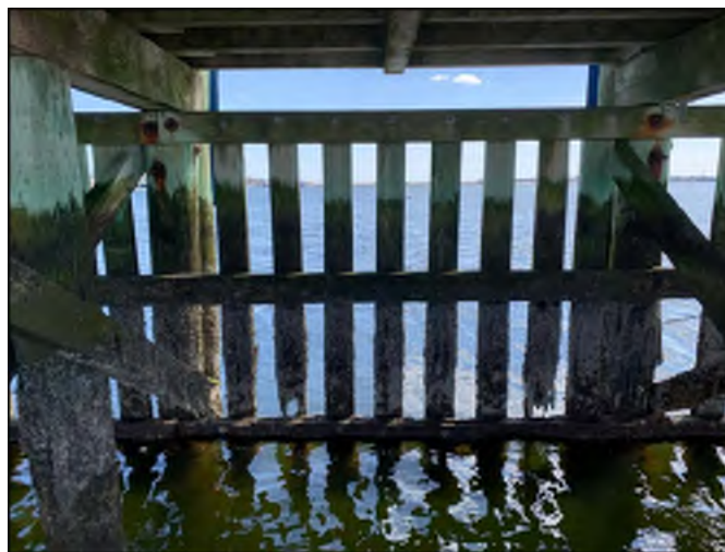
Timber wave fence along T-head of pier
