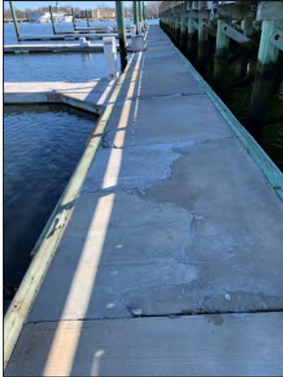
Photo No. 17: Previously repaired spalls with additional deterioration.
