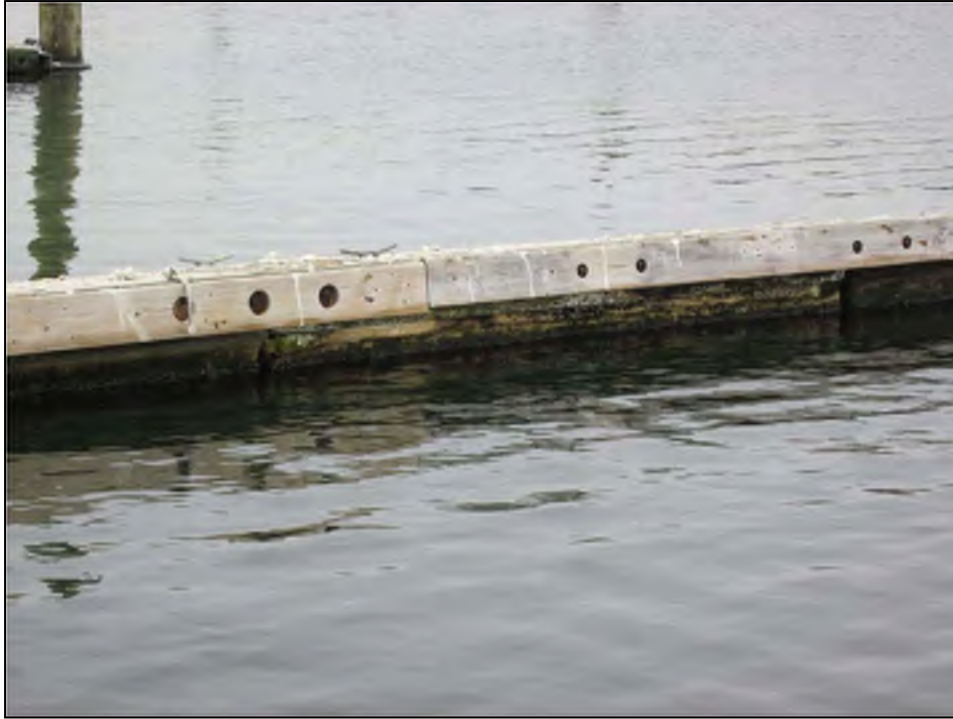
Photo No. 19: Deterioration of the concrete modules with exposed polystyrene at a finger float.
