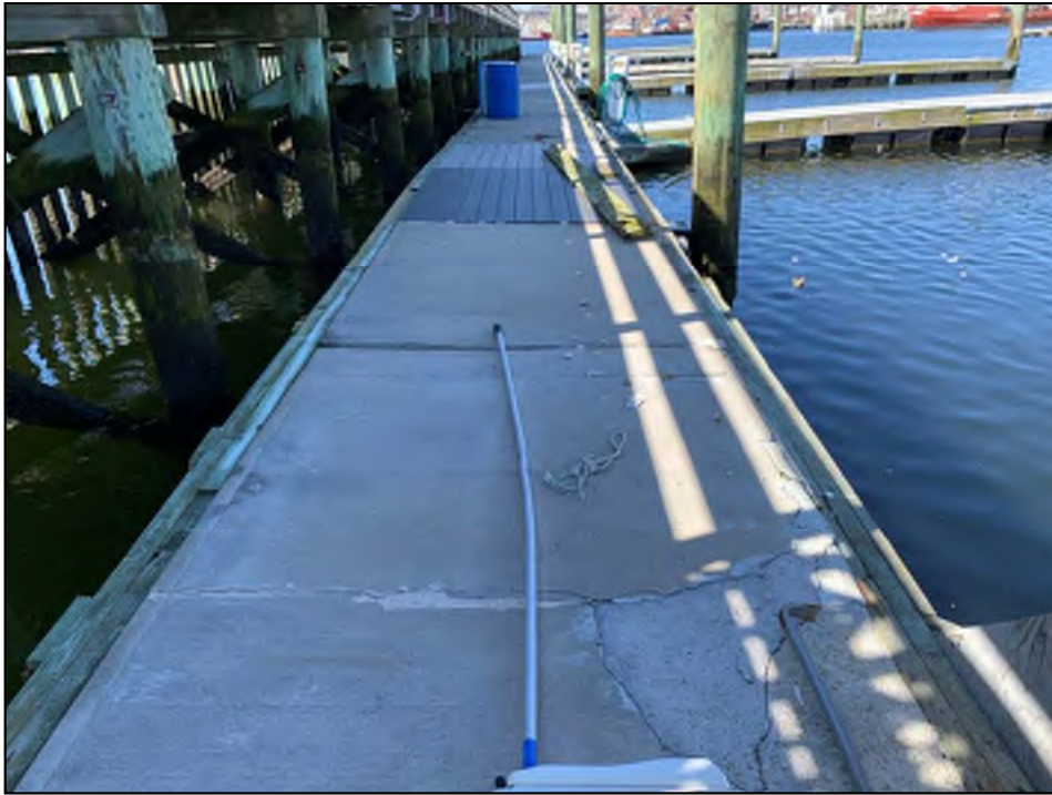
Photo No. 37: Deteriorated concrete main float along Dock D before storm.
