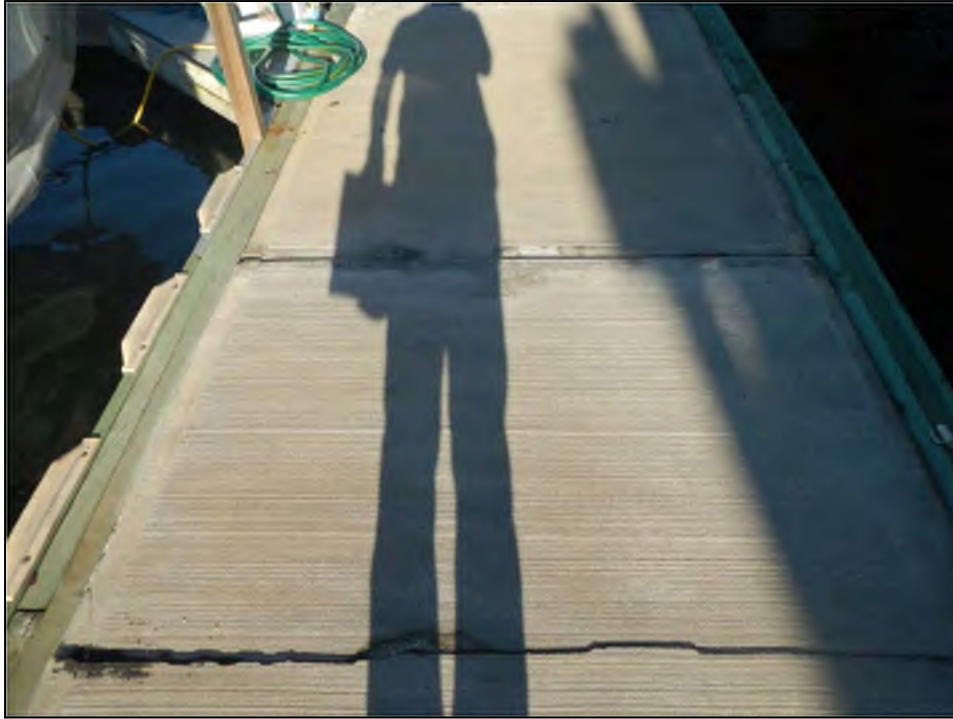
Photo No. 17: Cracking and trip hazards along the concrete deck panels.
