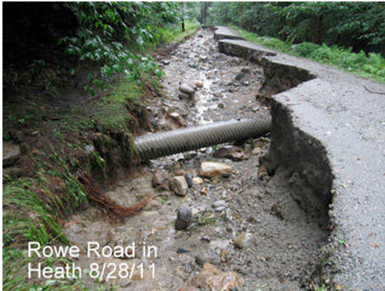
Photo: Failed culverts resulting in road washout on Rowe Road/Dell Road between Rowe and Heath after Tropical Storm Irene.
