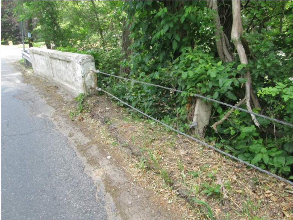
Photo 21: Southeast Transition Two Steel Wire Transition Rail
