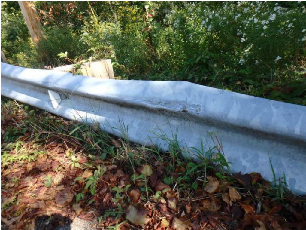
Photo 6: Northeast guardrail has minor scrapes and dents near buried end treatment.
