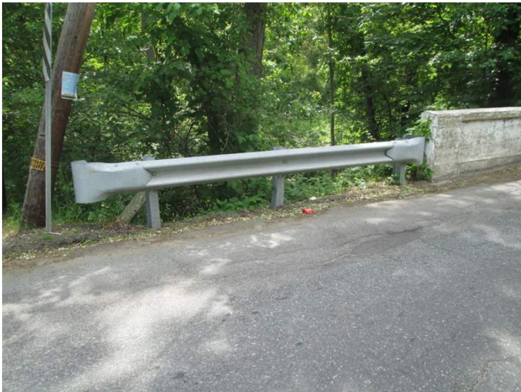
Photo 20: Northeast Transition Rail Does Not Connect with Bridge Rail (Parapet)
