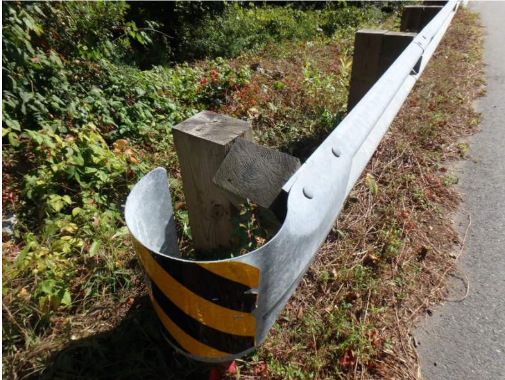
Photo 7: Northwest guardrail end with loose misaligned spacer block.
