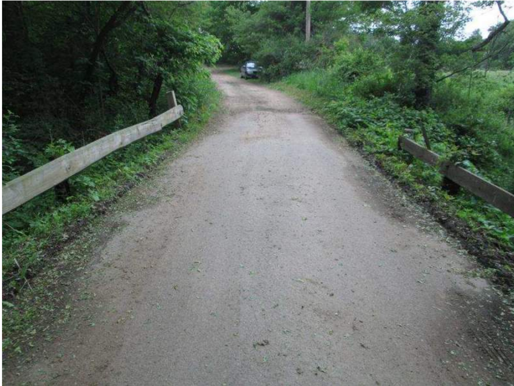
Photo 1: Typical Bridge Wearing Surface Tire Wear
