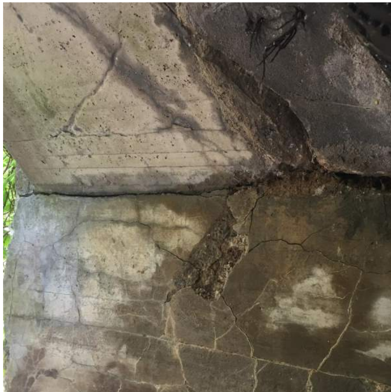
Photo 12: North Spring Line Near West Fascia Crack/Spall with Active Leakage
