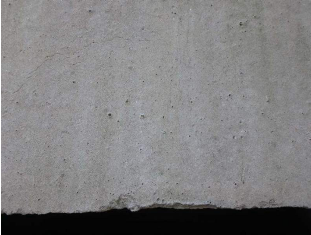
Photo 5: North face of rigid frame section 4 has minor hairline cracks at midspan
