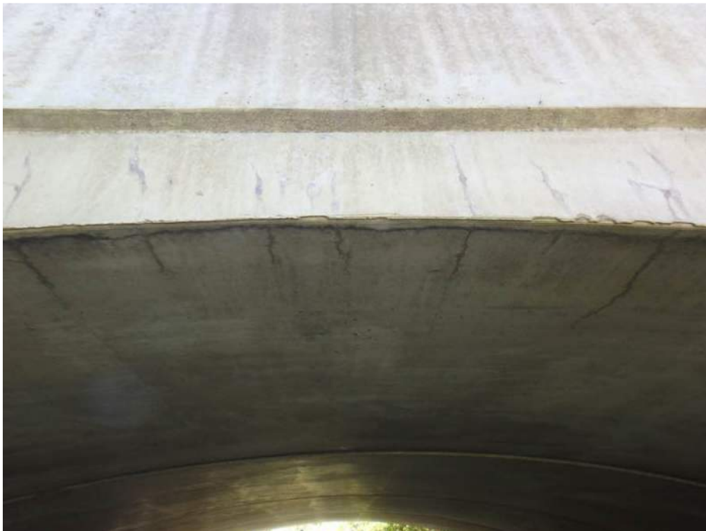
Photo 2: Cracking at north face of Span 1 Section 4 (typical)
