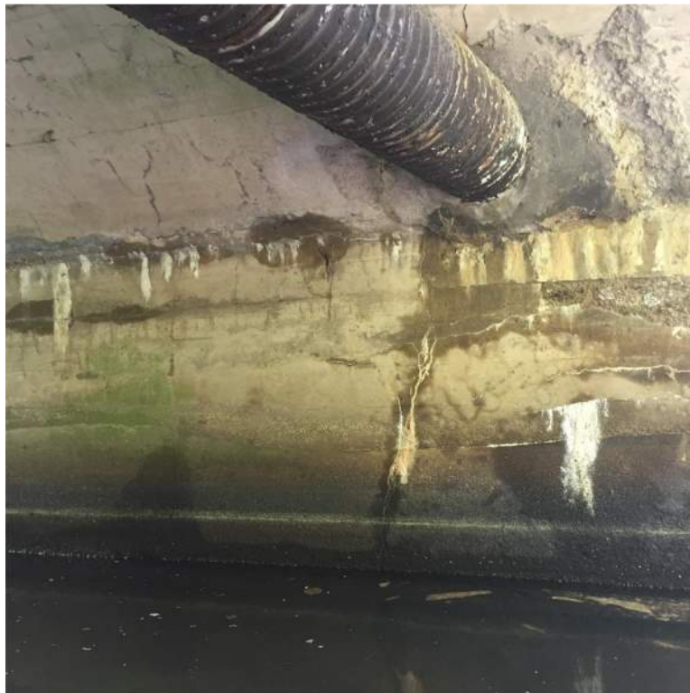
Photo 4: South Spring Line Utility Patch Spall with Crack
