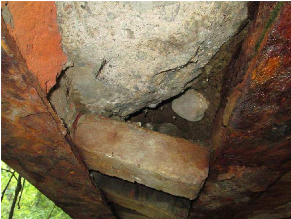
Photo 4: East Fascia Deck Underside Between Rails R-19 and R-20 Spall
