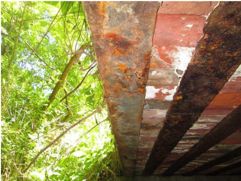
Photo 8: West Fascia Rail R-1 Bottom Flange Typical Span Heavy Rusting
