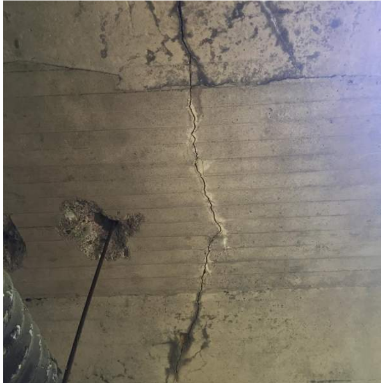
Photo 9: Typical Utility Support Embedded in Arch with Spall
