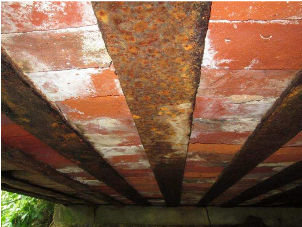
Photo 18: Rail R-16 Bottom Flange Typical Span Surface Rusting
