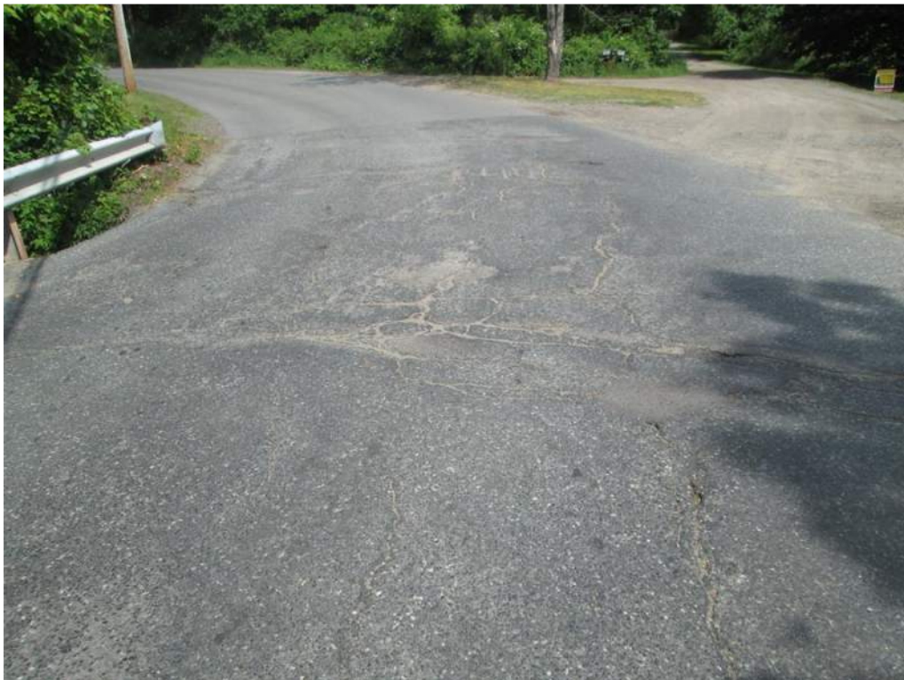
Photo 6: North Approach Pavement with Map Cracking
