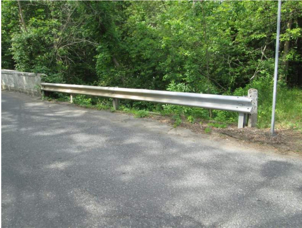
Photo 19: Northwest Transition Rail Does Not Connect to Bridge Rail (Parapet)
