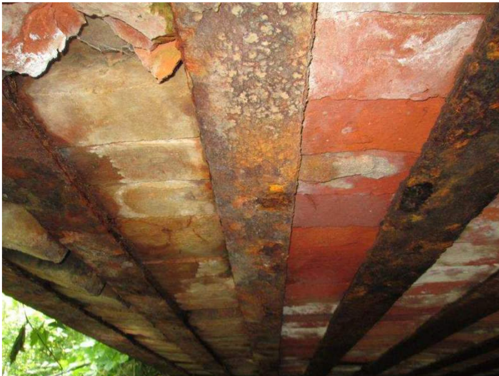
Photo 20: Rail R-18 Bottom Flange Typical Span Heavy Deterioration
