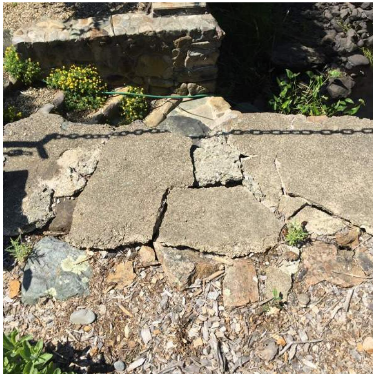
Photo 8: South Bridge Rail Concrete Leveling Pad Deteriorated/Broken Section
