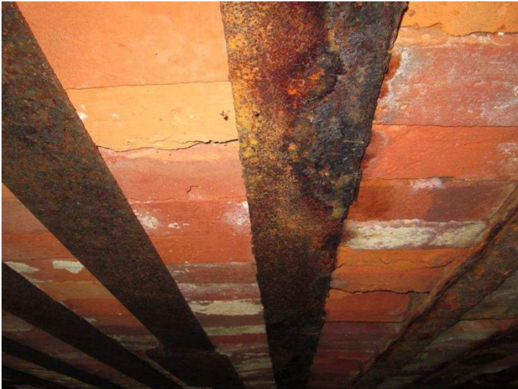
Photo 16: Rail R-12 Bottom Flange Typical Span Heavy Deterioration
