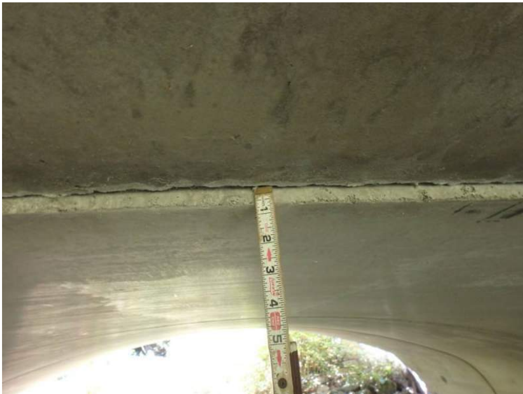
Photo 4: Span 1, Section 3/Section 4 interface: Section 3 is 3/4" lower than Section 4 at crown.
