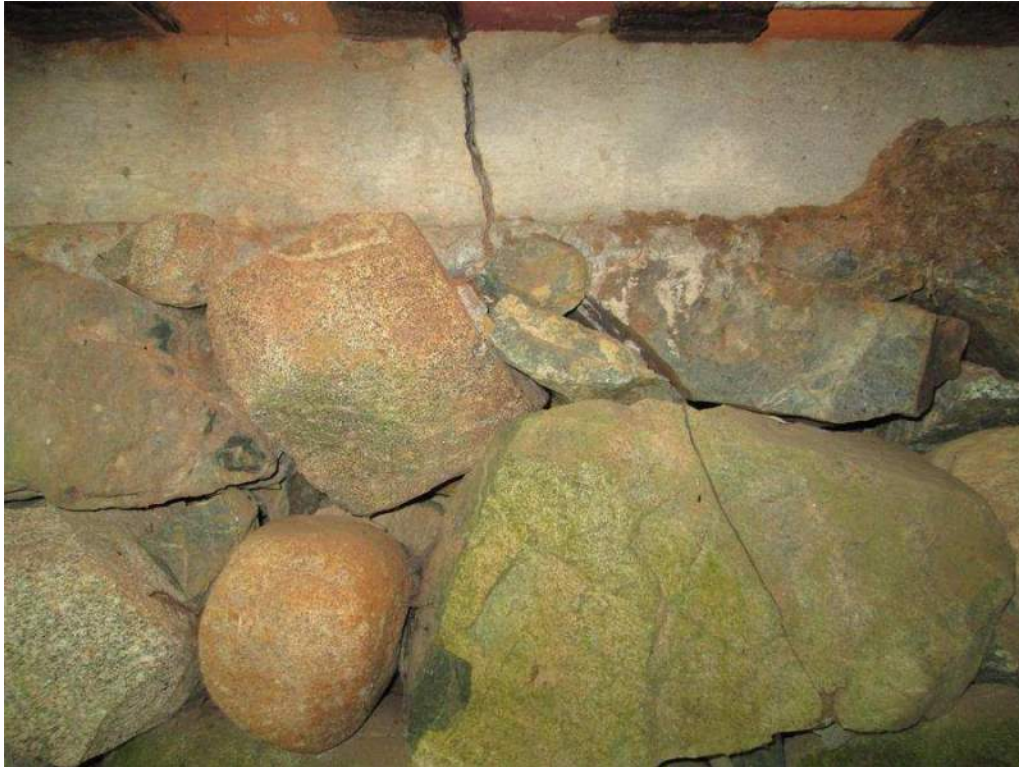
Photo 23: South Abutment Cracked Stone Below Rail R-15
