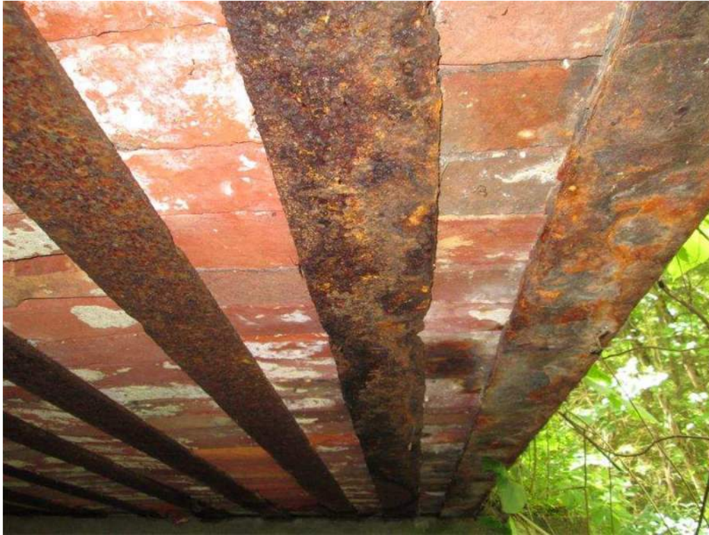
Photo 9: Rail R-2 Bottom Flange Typical Span Heavy Deterioration
