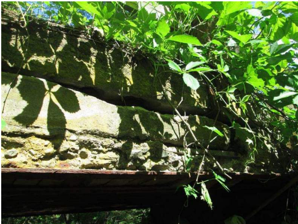
Photo 2: East Fascia Heavy Spalling
