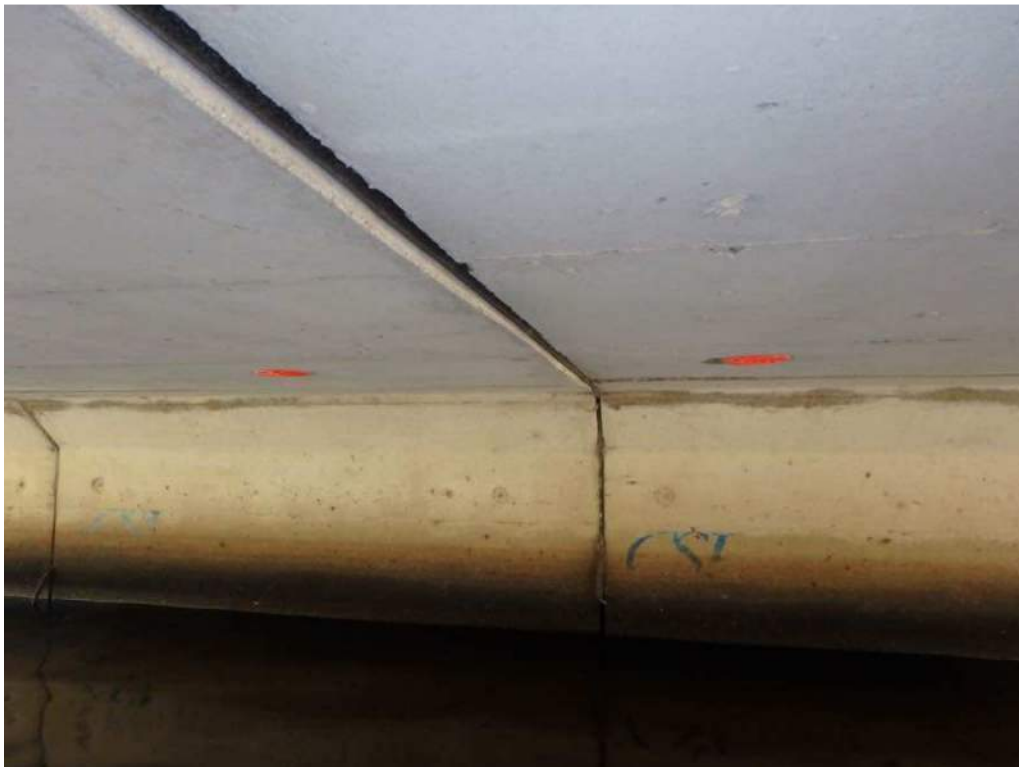
Photo 6: Misalignment of approx. 1/2" at the interface of rigid frame sections 2 and 3 near east wall
