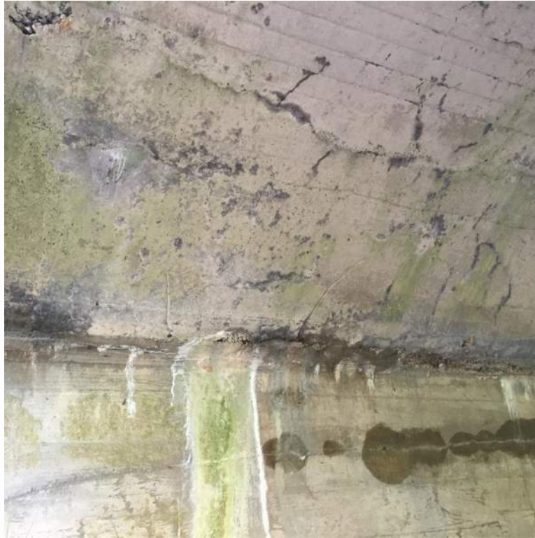
Photo 11: South Spring Line near East Fascia Spring Line Spall with Active Leakage and Efflorescence
