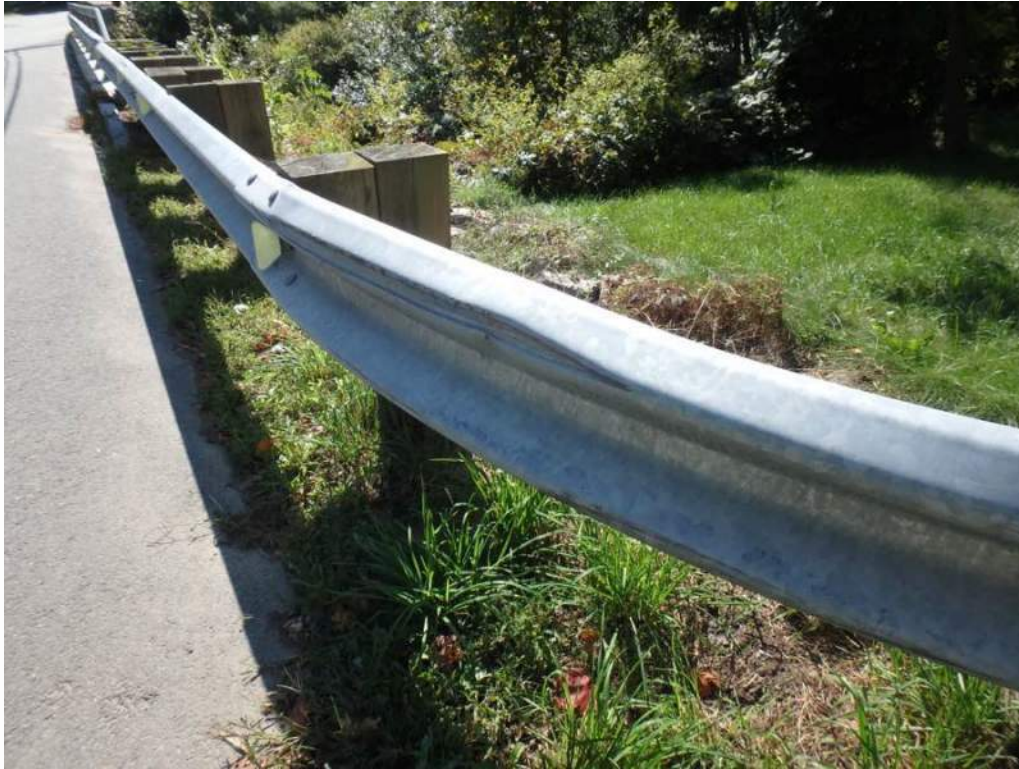
Photo 5: Southwest approach guardrail minor scrapes and dents.
