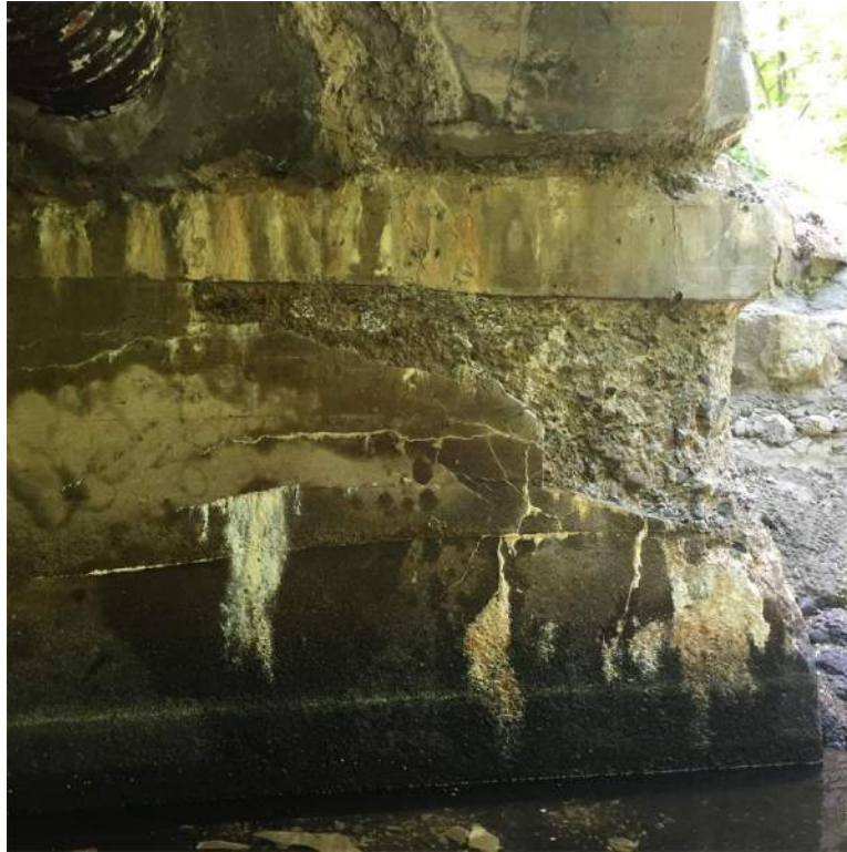
Photo 15: South Breastwall at West Fascia Spalled Concrete that Extends into Southwest Wingwall
