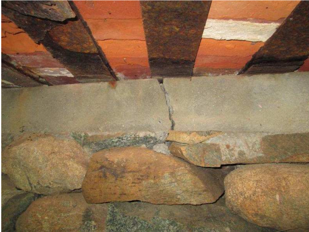
Photo 25: North Abutment Concrete Bridge Seat Crack Below Rail R-8
