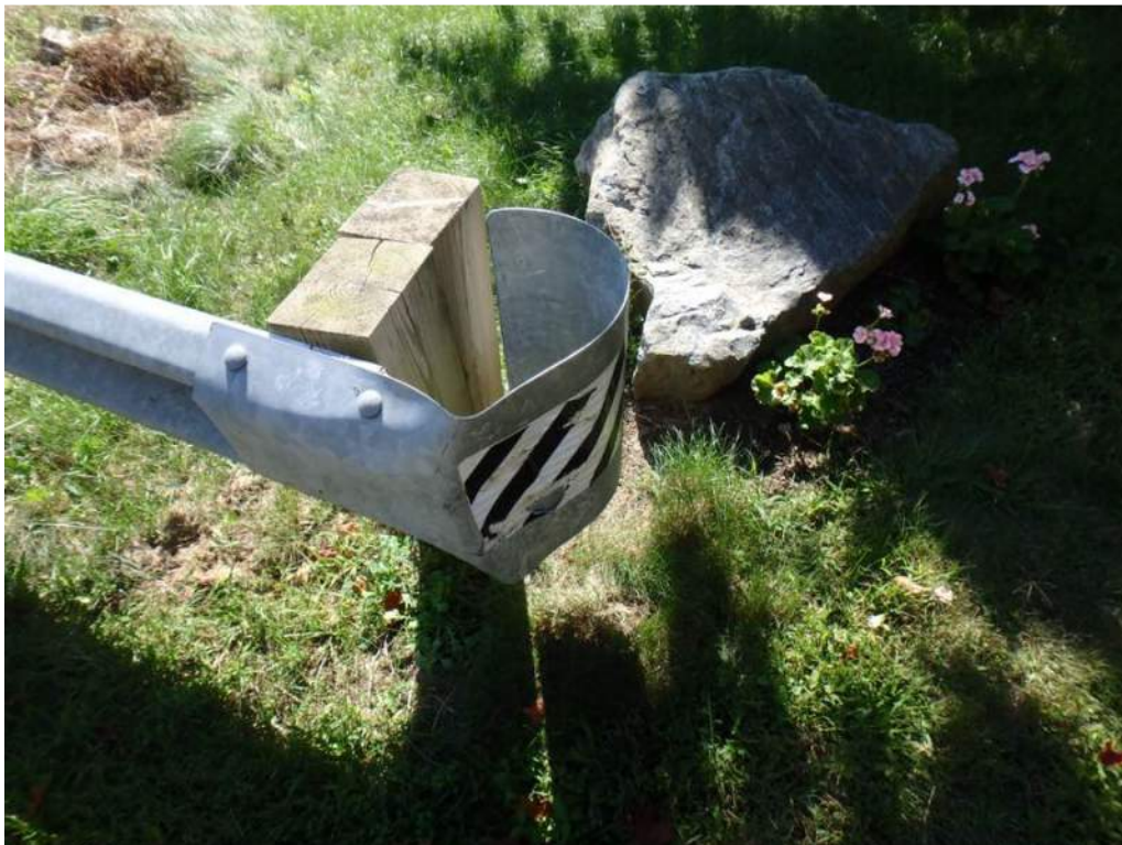
Photo 8: Southwest boxing glove end treatment has minor damage.
