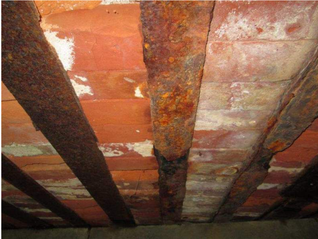
Photo 13: Rail R-10 Bottom Flange Typical Span Heavy Deterioration
