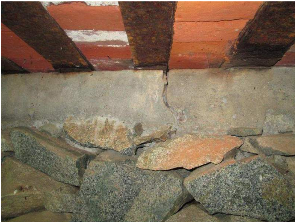
Photo 26: North Abutment Concrete Bridge Seat Crack Below Rail R-13
