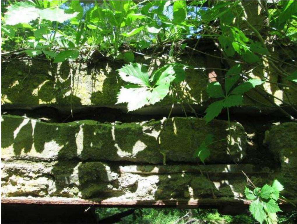
Photo 3: East Fascia Spalling with Exposed Outside Face of Rail R-20
