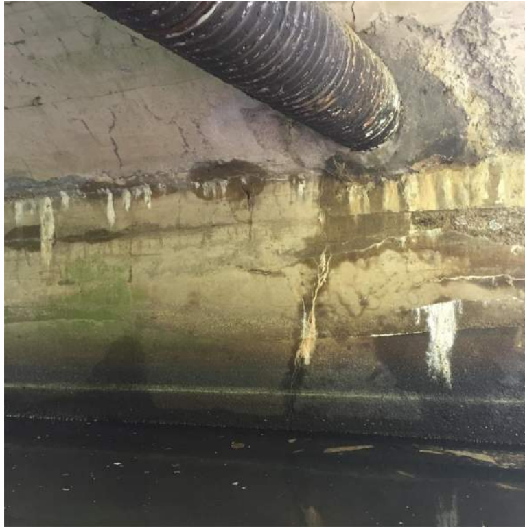
Photo 13: Southwest Breastwall Map Cracking with Efflorescence and Active Leakage
