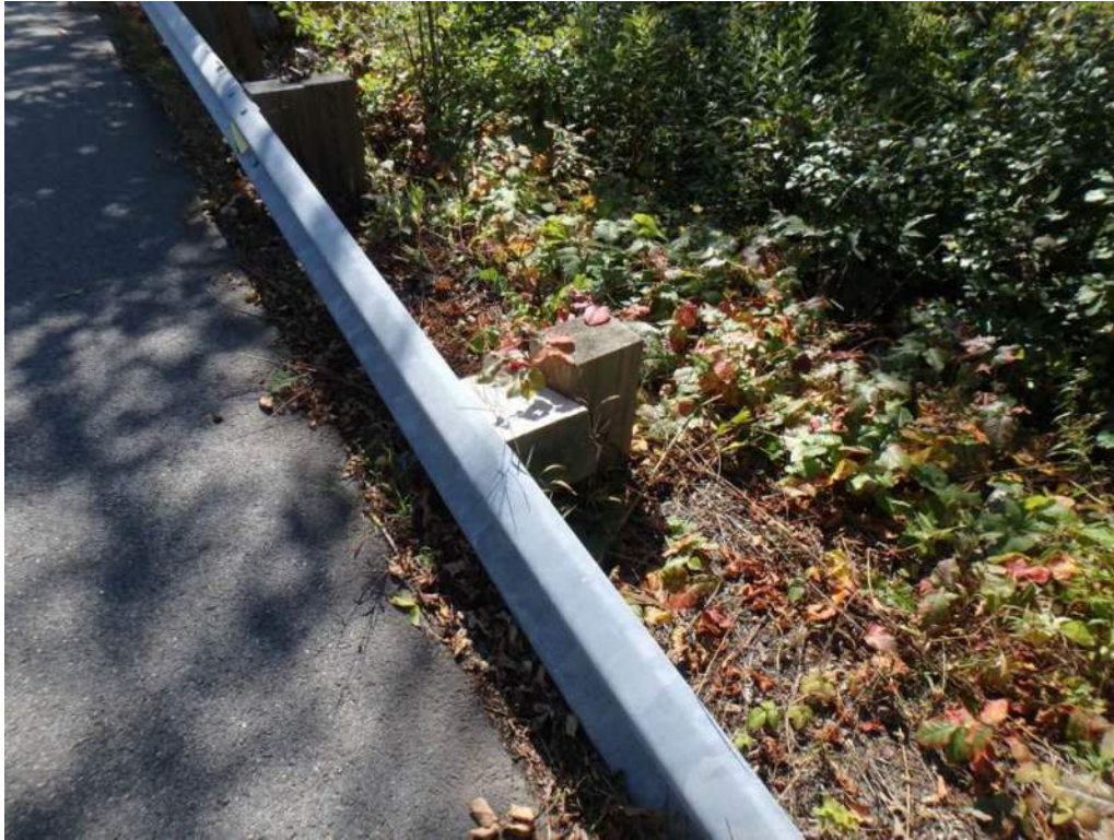
Photo 1: Loose and misaligned guardrail spacer block.
