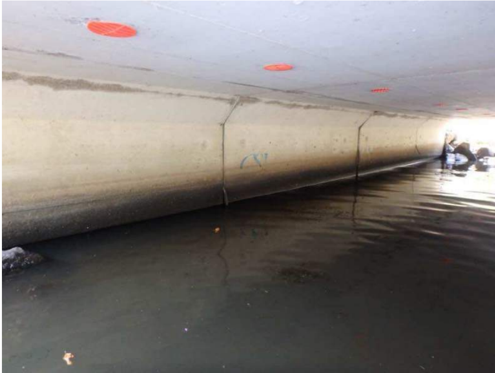
Photo 3: East wall has loose joint filler between rigid frame sections 1 and 2, 2 and 3, and 3 and 4.
