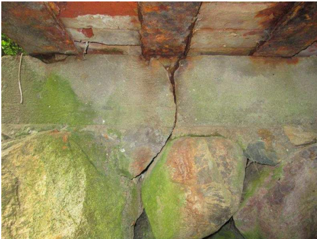
Photo 24: South Abutment Concrete Bridge Seat Full Depth Crack Under Rail R-19
