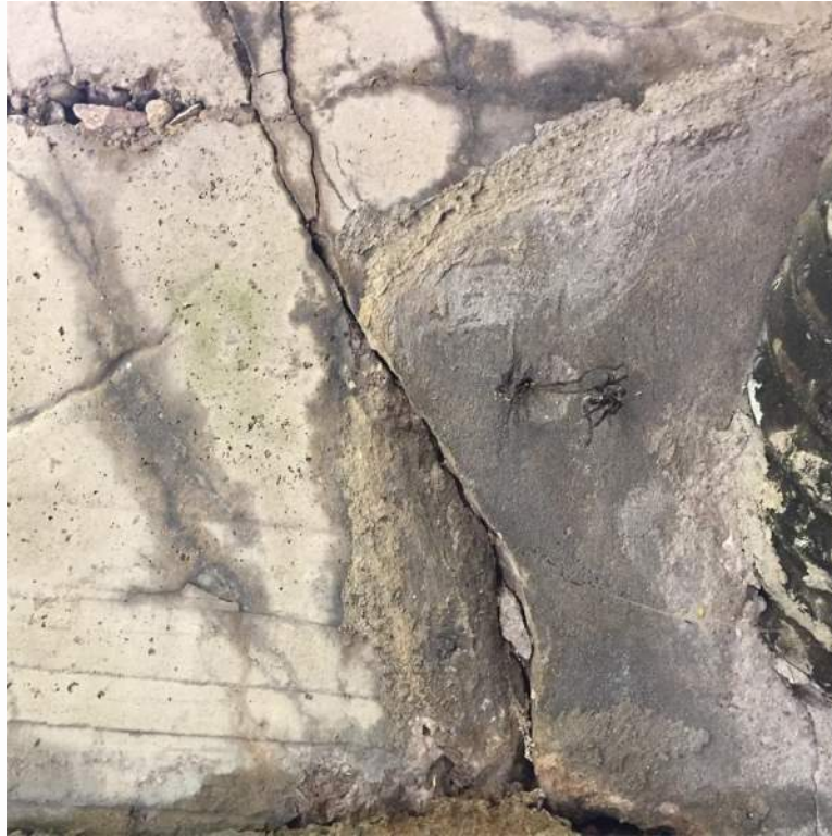
Photo 5: North Spring Line Utility Patch Spall with Crack Propagating into Arch
