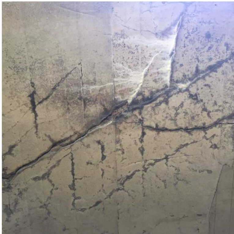
Photo 8: West Arch Underside Crack from Utility Patch to Utility Patch with Cracks Propagating off Main Crack
