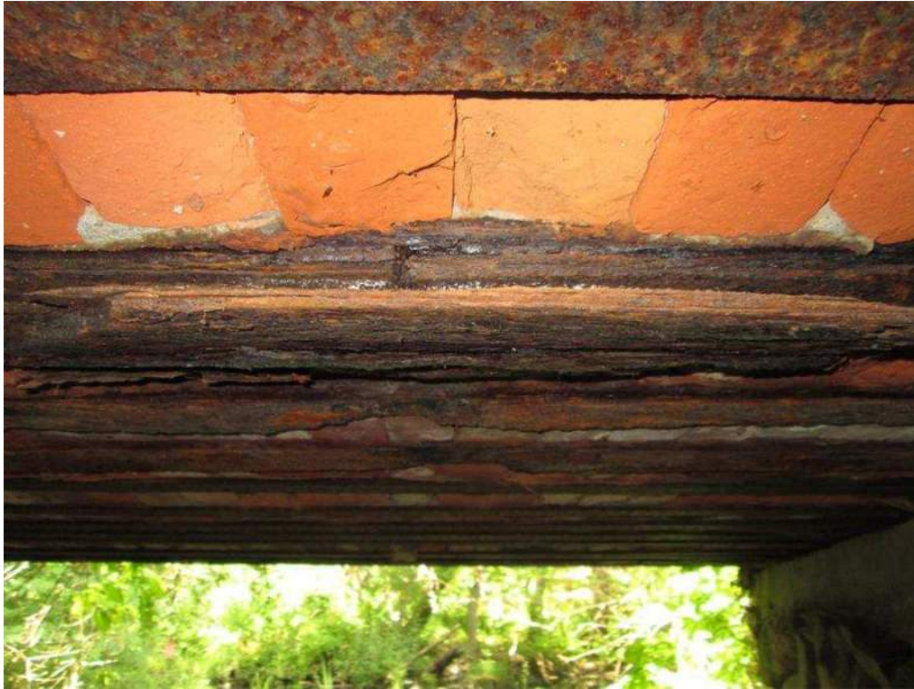
Photo 17: Rail R-12 at North End Bottom Flange Splice and Heavy Deteriorated Splice Plate
