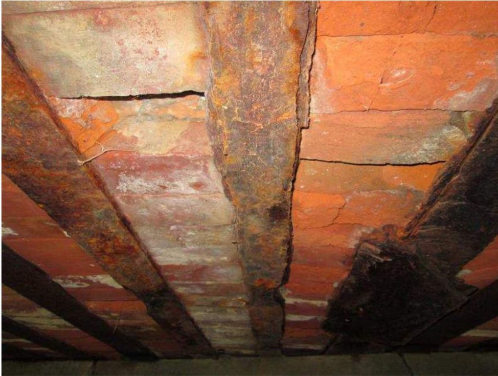
Photo 15: Rail R-11 Bottom Flange Typical Span Heavy Deterioration
