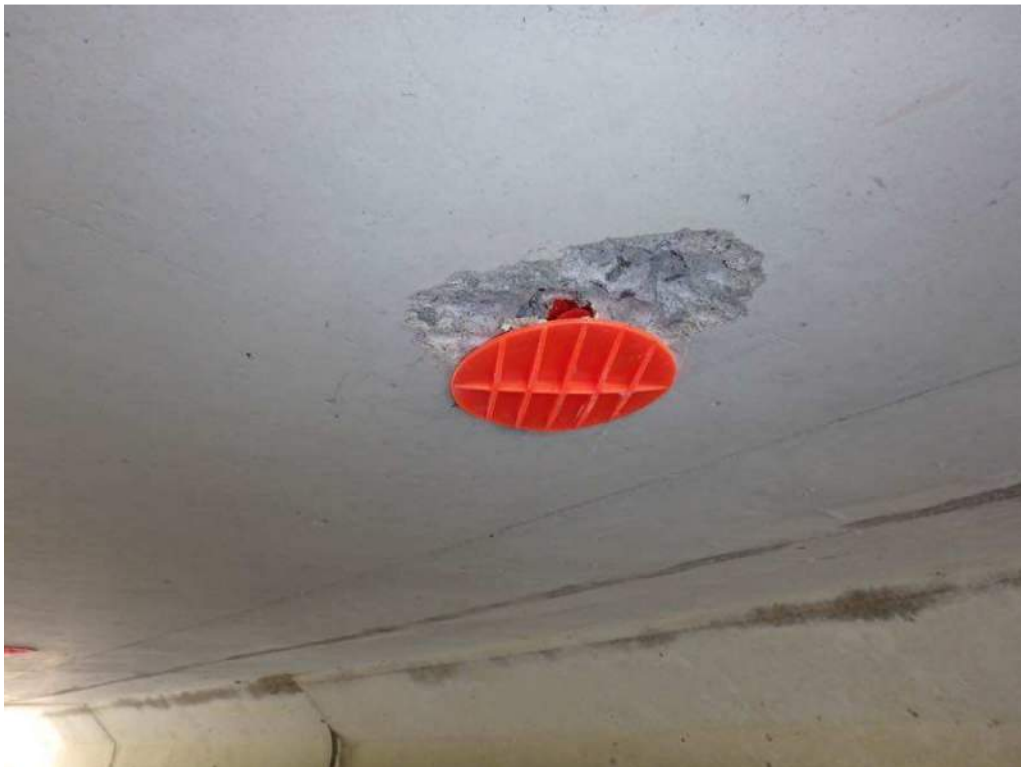
Photo 4: Spall at plastic insert in rigid frame section 3 near north east corner
