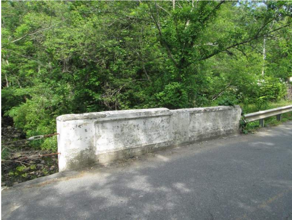
Photo 3: West Bridge Rail (Parapet) with Northwest Top Concrete Section Spalled
