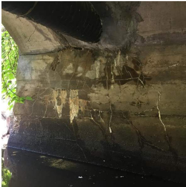
Photo 14: Northwest Breastwall Map Cracking
