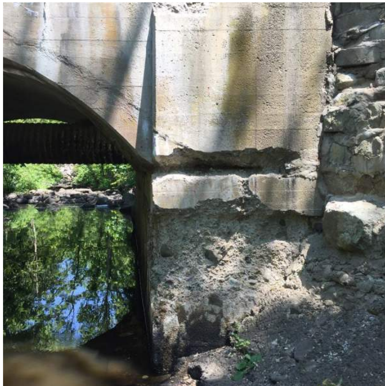
Photo 16: Southwest Wingwall Spall
