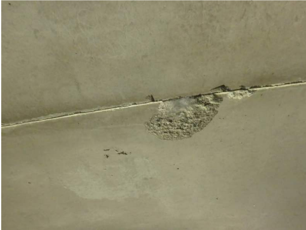
Photo 3: Spall at Span 1 Section 3: 8" Diameter x 1" deep.
