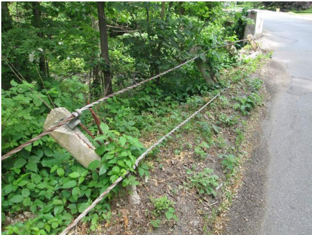
Photo 22: Southwest Approach Two Wire Cable Steel Rail and Concrete Posts Bent/Broken with up to 100% Loss of Section
