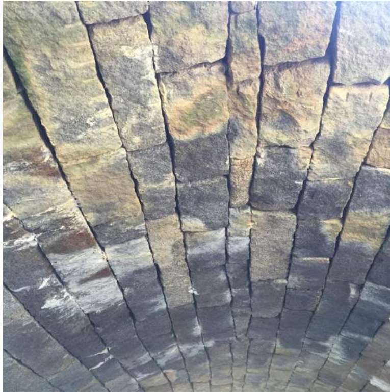
Photo 1: Arch Crown Underside Exposed Efflorescence
