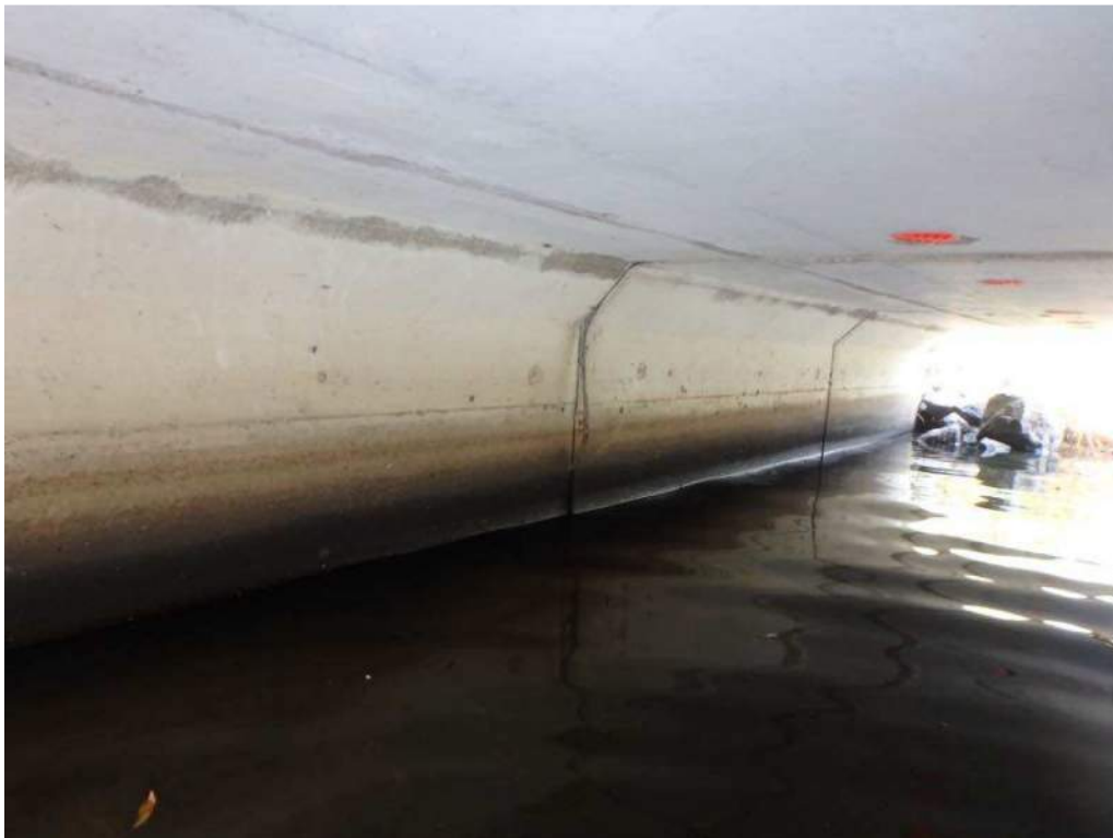
Photo 2: West wall has loose joint filler between rigid frame sections 2 and 3.
