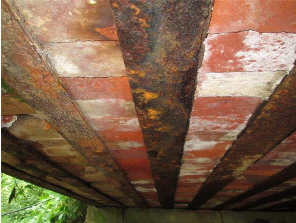
Photo 19: Rail R-17 Bottom Flange Typical Span Heavy Deterioration
