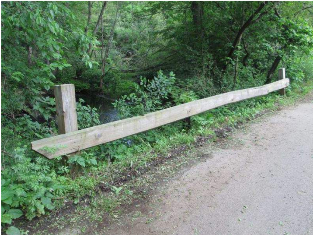
Photo 30: West Bridge Rail Span Over Bridge Without Posts on Bridge
