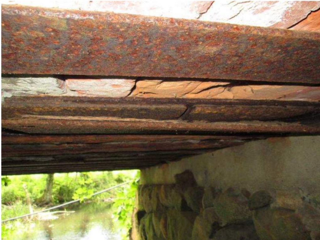
Photo 12: Rail R-9 Bottom Flange Splice and Splice Plate
