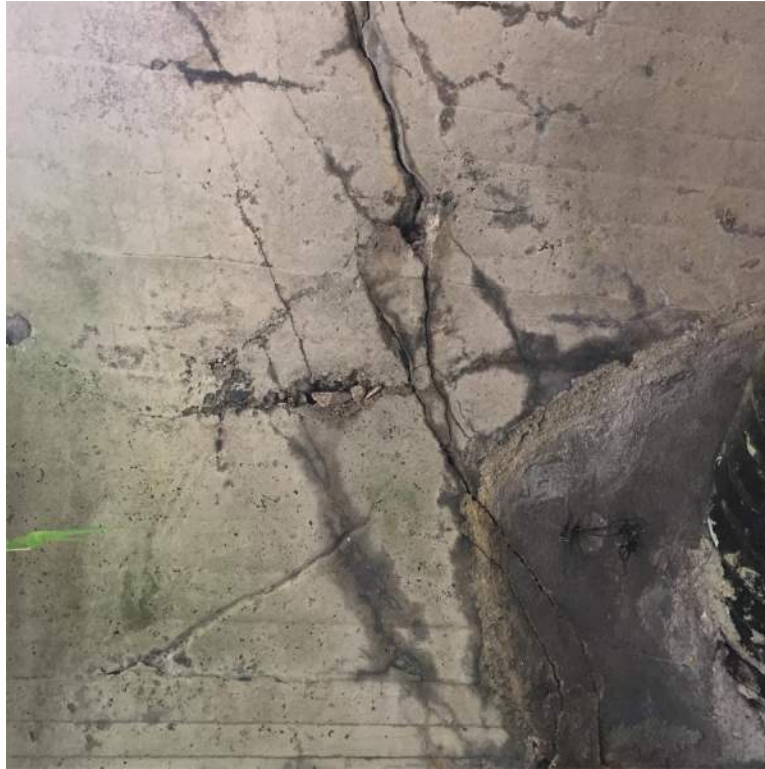
Photo 7: Northwest Arch/Arch Ring Crack Propagating from Utility Patch
