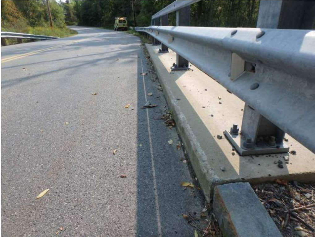
Photo 1: South curb has minor scrapes throughout
