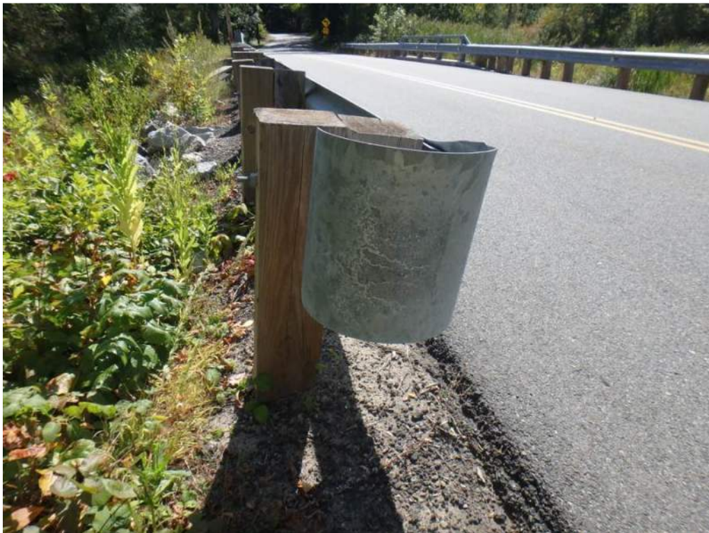
Photo 2: Northwest guardrail end post rotated towards roadway.
