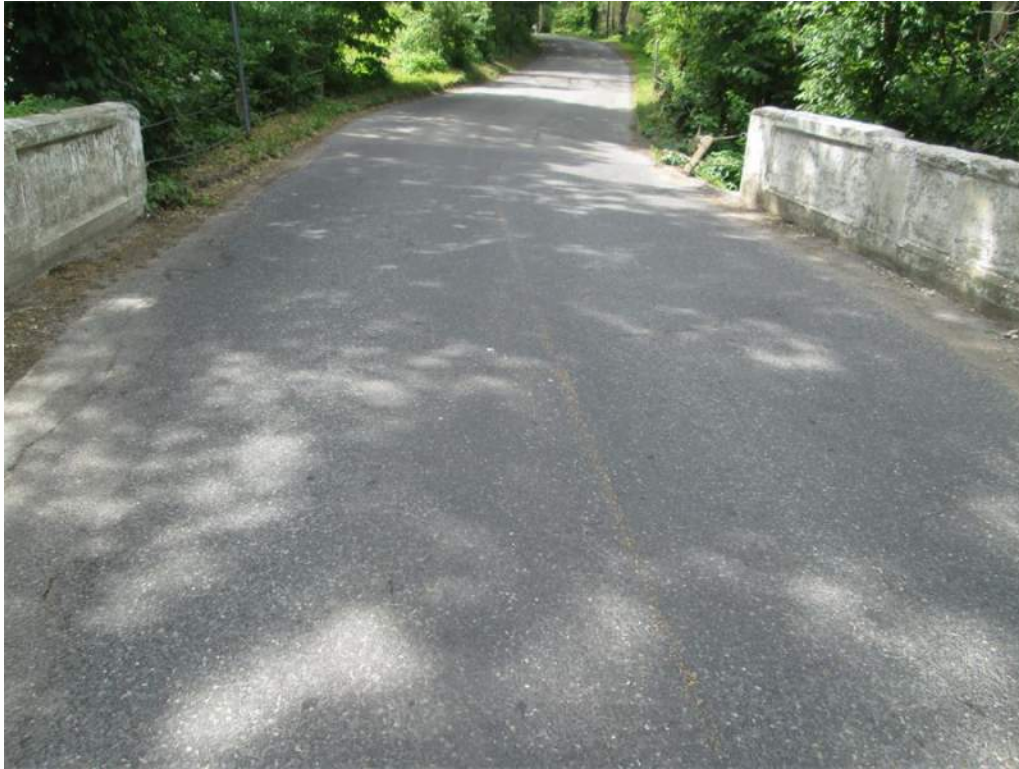
Photo 1: Bridge Wearing Surface Transverse Cracking with Tire Wear
