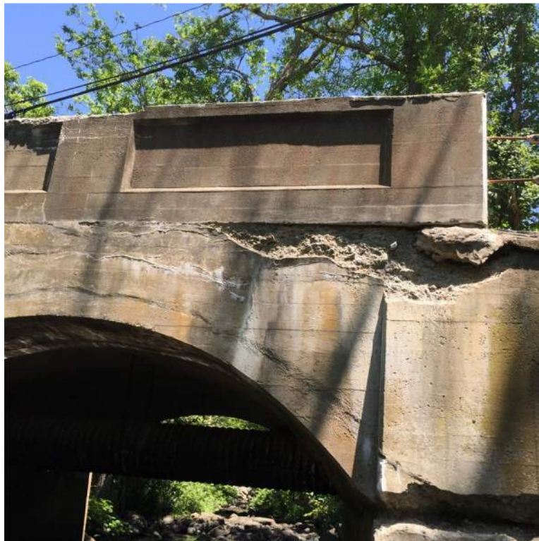
Photo 10: Southwest Spandrel Wall Spall Under Parapet Extending into Southwest Wingwall
