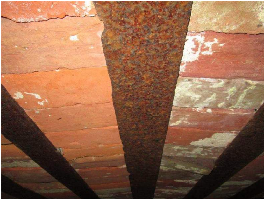
Photo 10: Rail R-5 Bottom Flange Typical Span Surface Rusting
