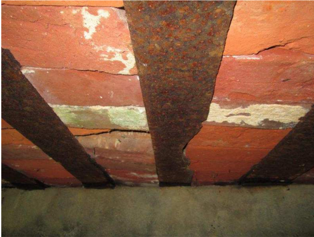
Photo 11: Rail R-6 Bottom Flange Typical Span Surface Rusting and Notched Area
