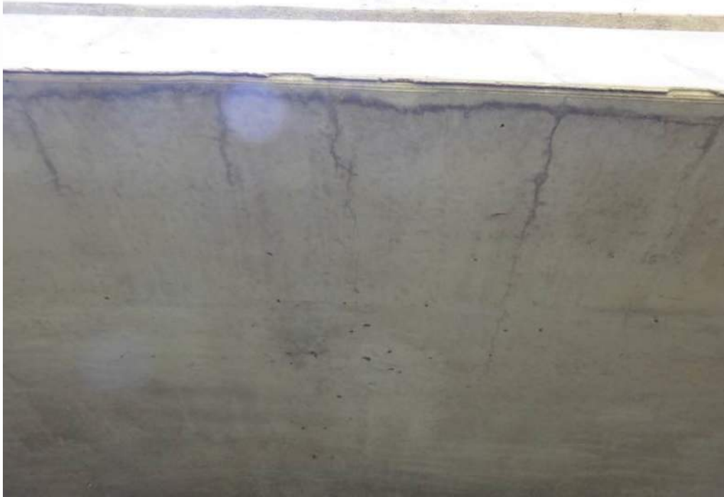
Photo 1: Cracking at Span 1 Section 4 intrados. (Typical throughout both spans)
