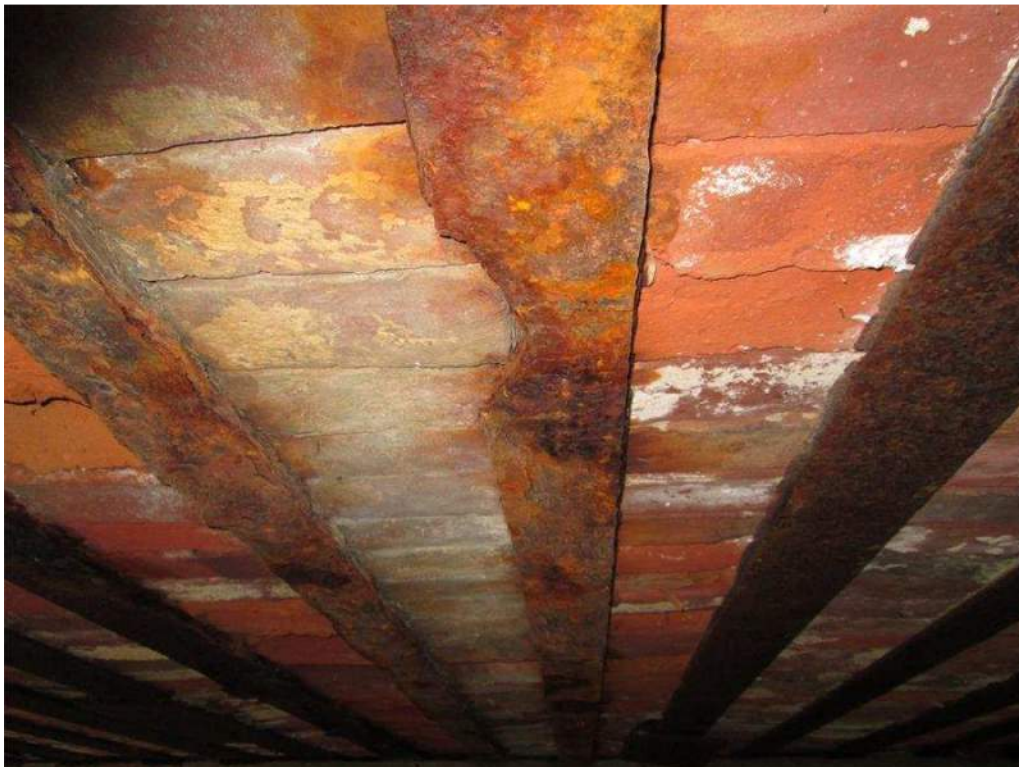
Photo 14: Rail R-10 at Midspan Bottom Flange Partial Loss of Section
