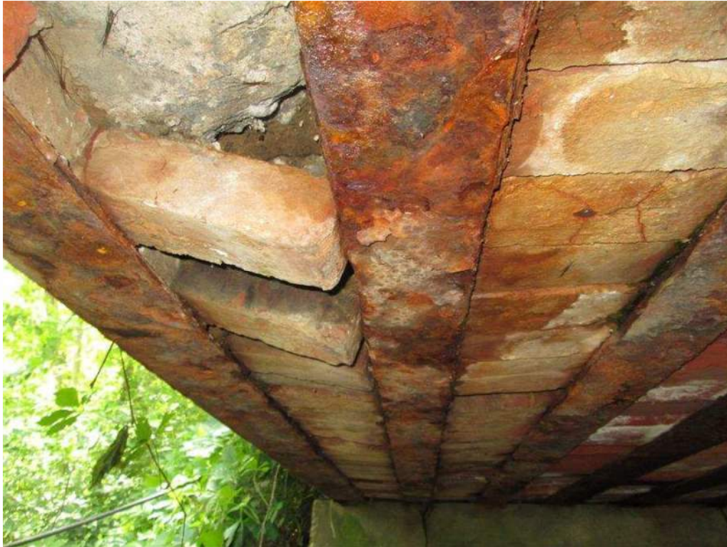
Photo 21: Rail R-19 Bottom Flange Typical Span Heavy Deterioration with Active Leakage
