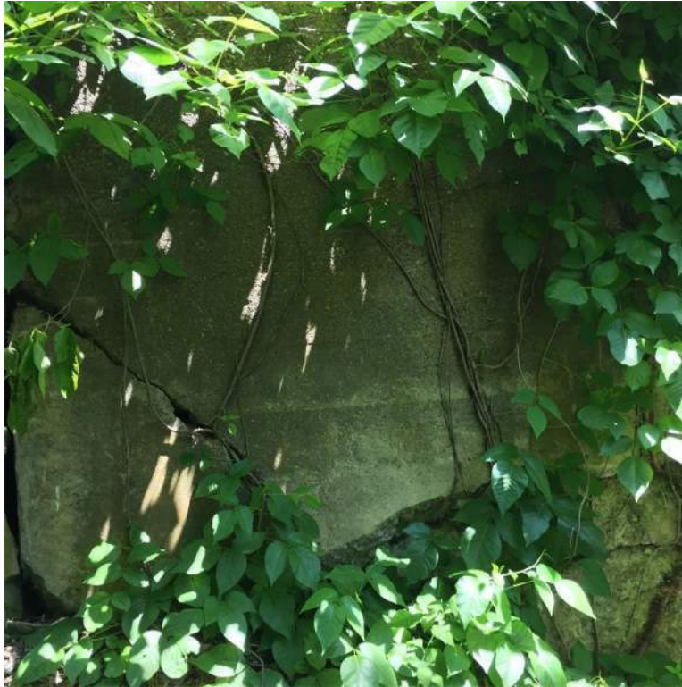
Photo 17: Northwest Wingwall Cracked/Broken Section
