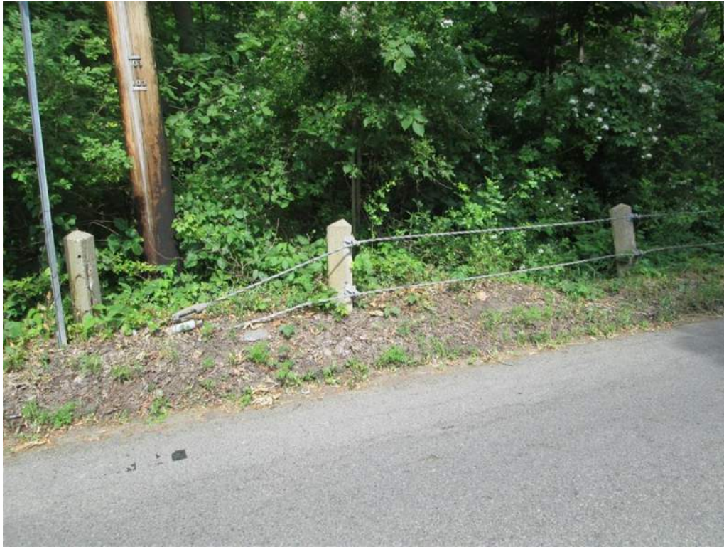
Photo 23: Southwest Approach Two Wire Cable Steel Guardrail Buried End
