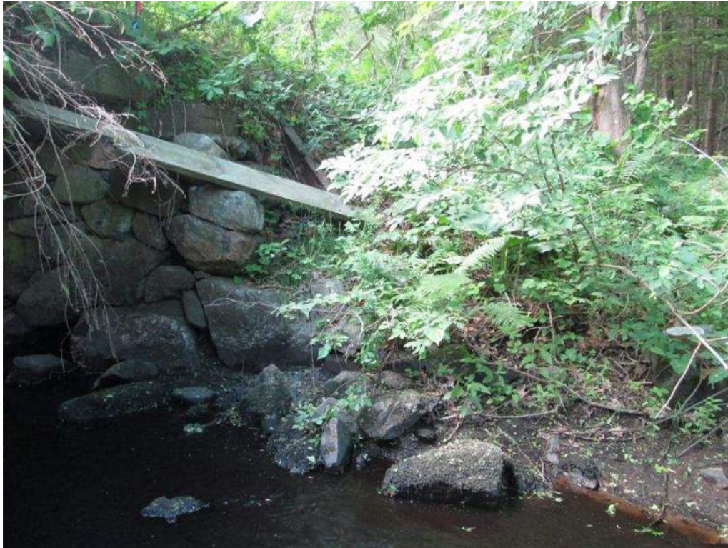
Photo 27: Northeast Wingwall Dislodged Stones
