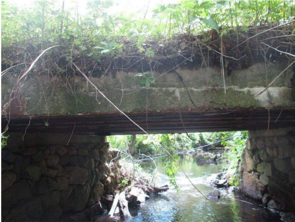
Photo 5: West Fascia Cold Joint Crack with Efflorescence and Rust Staining
