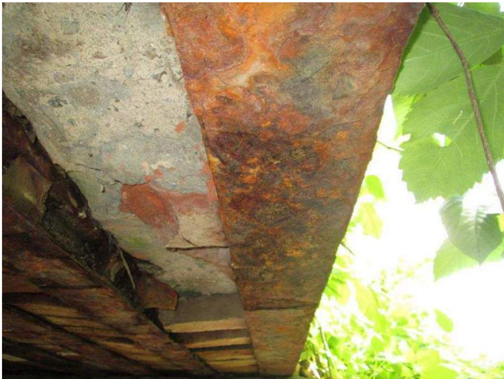
Photo 22: Rail R-20 Bottom Flange Typical Span Heavy Deterioration
