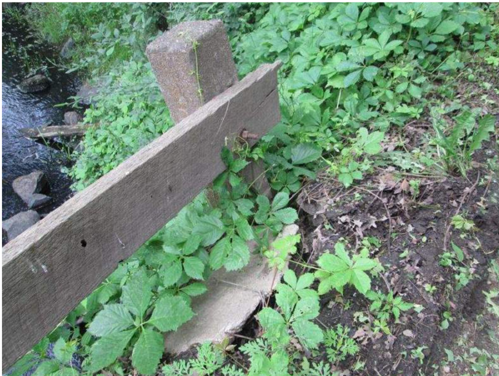
Photo 28: Southeast Bridge Rail Concrete Post Base Separation
