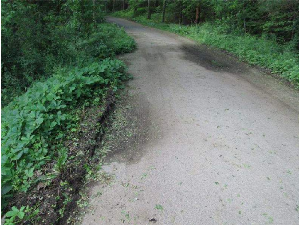
Photo 7: South Approach Pavement Settlement (Looking South) at Southeast Side of Road
