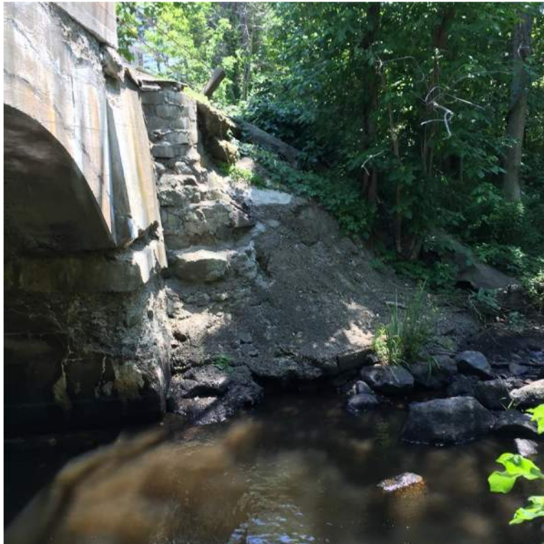
Photo 18: Southwest Embankment Slope Paving that is Cracked/Deteriorated
