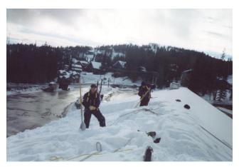
A method to protect workers from falling is required. One example of Fall Protection is a full-body harness with a shock-absorbing lanyard attached to a rope grab and vertical lifeline that is attached to a separate 5000-pound anchor point per worker.
