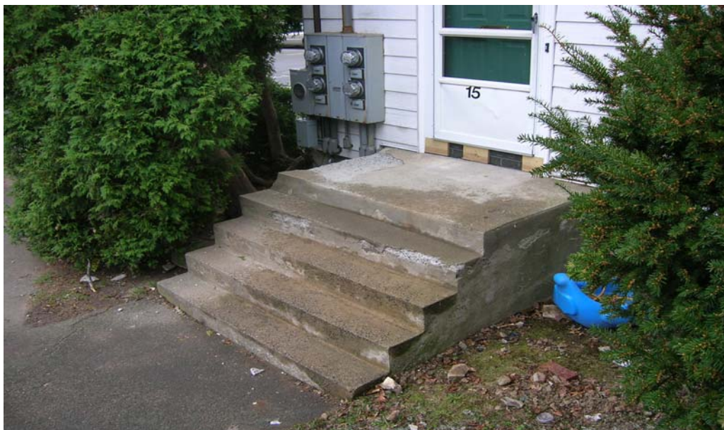
200-2 Family Housing Development, 15 Rainbow Terrace Building Exterior – Cement Stairs Deteriorating
