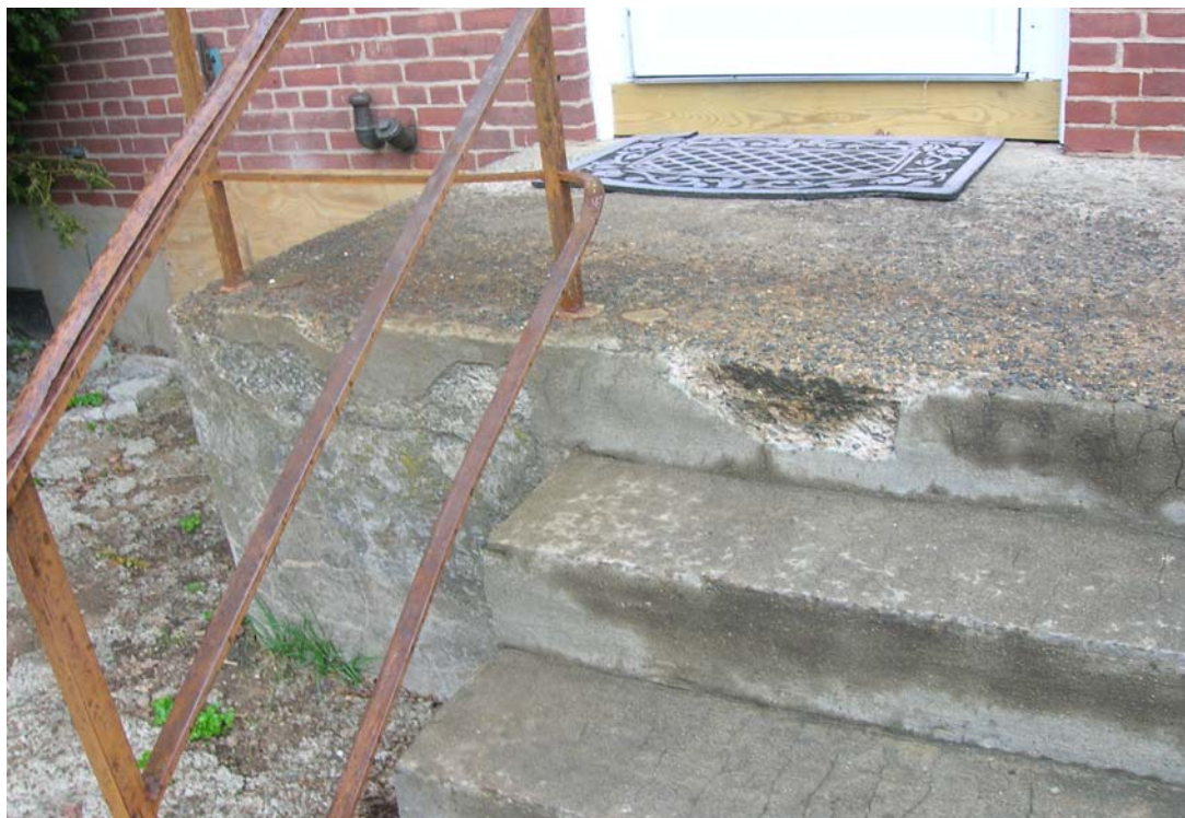
200-2 Family Housing Development, 75 Rainbow Terrace Building Exterior – Cement Stairs are Deteriorating
