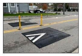
The fraction of vehicles exceeding the speed limit (25 mph) fell from 78% to 5% after the speed cushions were installed, though that fraction rose to 75% during the winter when they were removed. The number of vehicles going faster than 40 mph fell by 93%. Average speed fell from 29 to 20 mph (and then rose to 28 mph when the cushions were removed for the winter). Once the speed cushions were installed, there was no more parking on the sidewalk.
