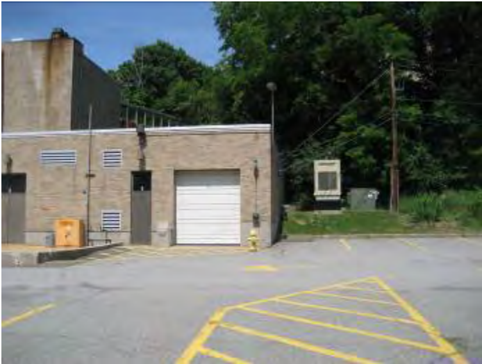
Side C, Doors 7 and 8
