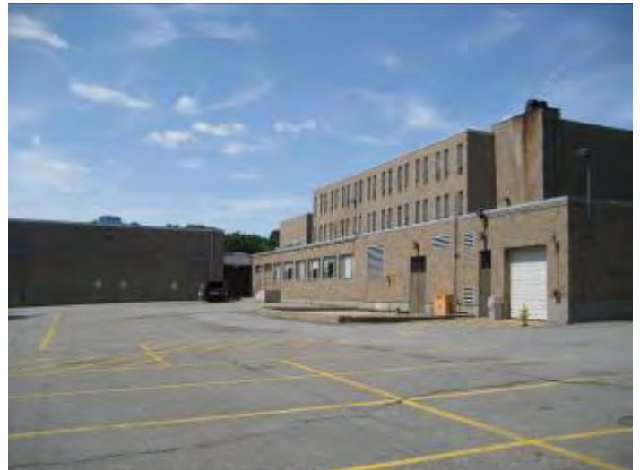
Side C, Rear of Building
