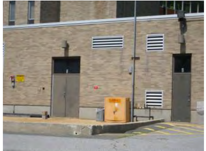
Side C, Doors 8 and 9
