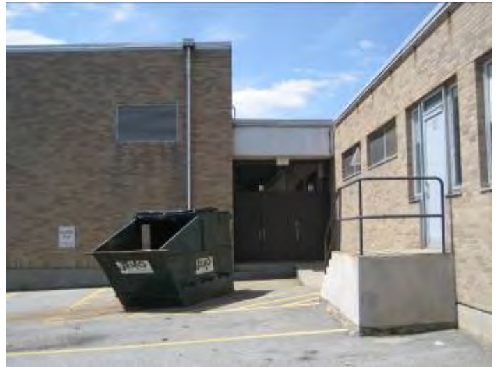
Side C, Doors 11 and 12
