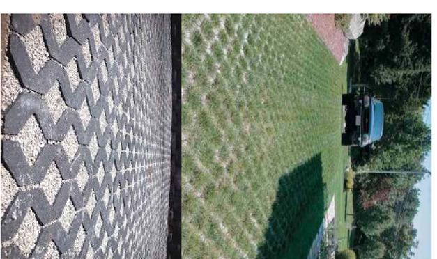
Pavers allow infiltration while providing structure for cars
