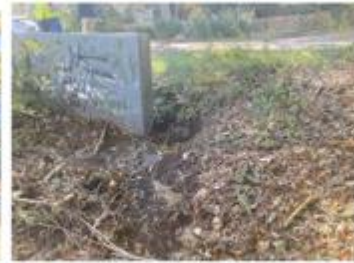
Stormwater bypass of existing catch basin (left) and erosion and sediment inputs to Pond (right) at Timberlane Drive/Lantern Lane site.
