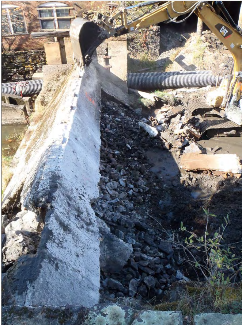
Figure 16. Rubblestone and cobble core exposed during concrete removal, view northwest.
