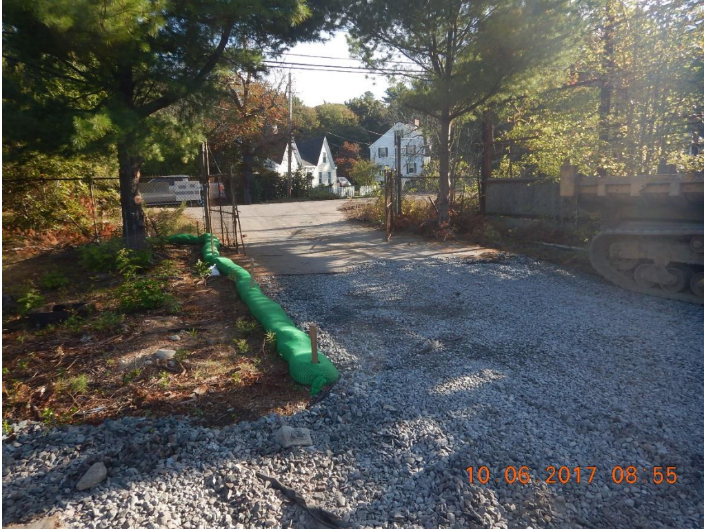
Photo 11: Stabilized Construction Entrance (mid-construction) (Gomez and Sullivan, 10/6/17)
