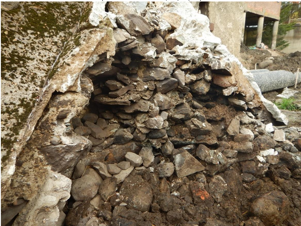
Photo 14: Partially removed dam with exposed material (mid-construction) (Gomez and Sullivan, 10/24/17)
