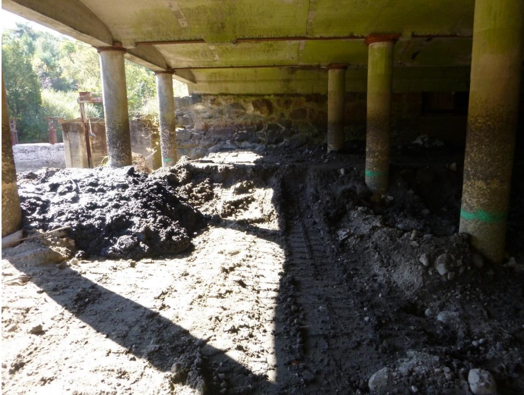
Photo 22: Looking upstream at constructed channel and removed dam (post-construction) (Gomez and Sullivan, 12/13/17)
