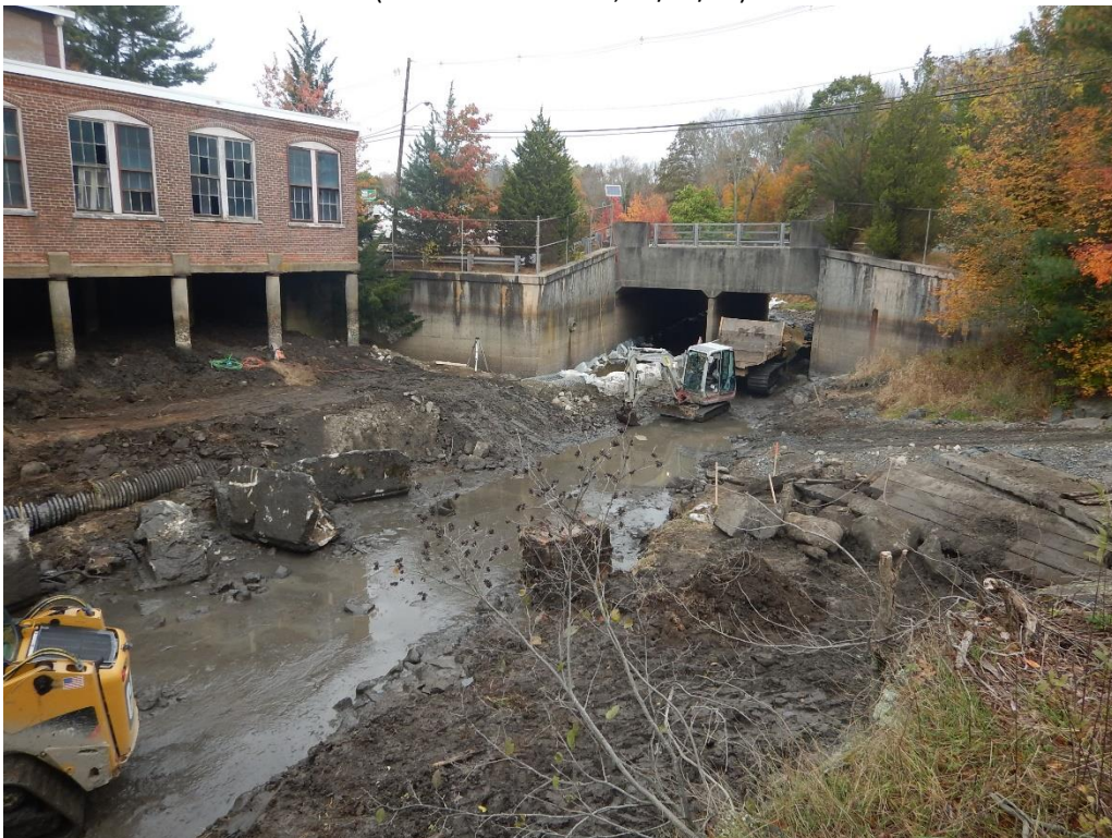
Photo 16: Looking upstream at channel excavation (mid-construction) (Gomez and Sullivan, 10/24/17)
