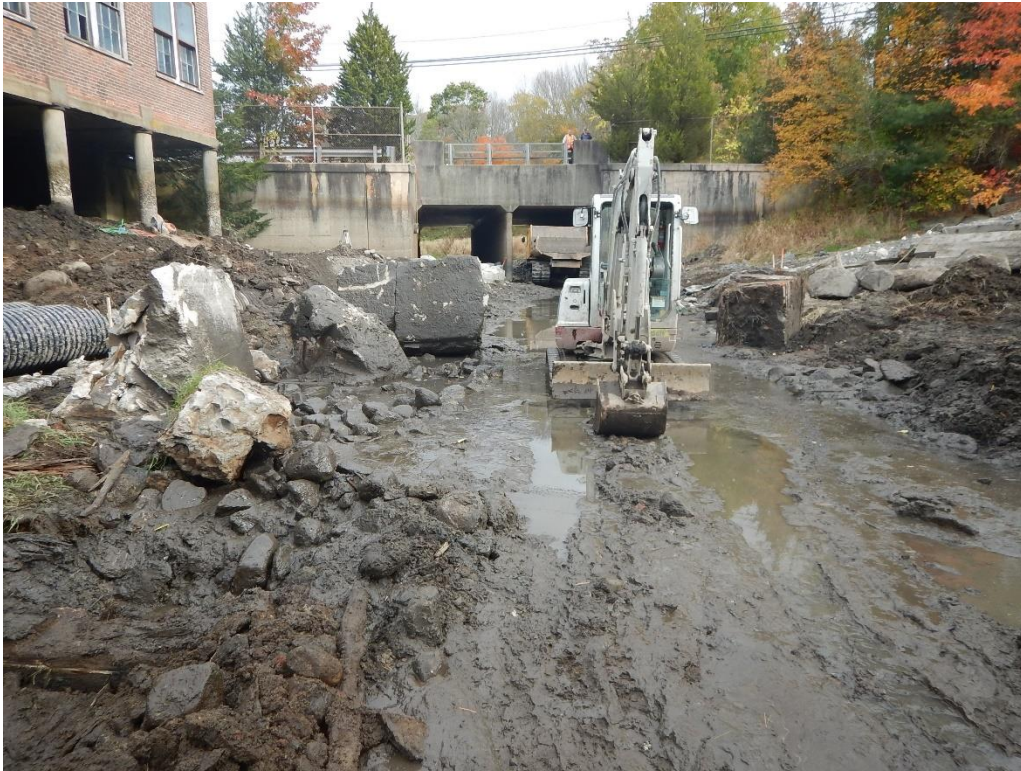
Photo 16: Looking upstream at channel excavation (mid-construction) (Gomez and Sullivan, 10/24/17)
