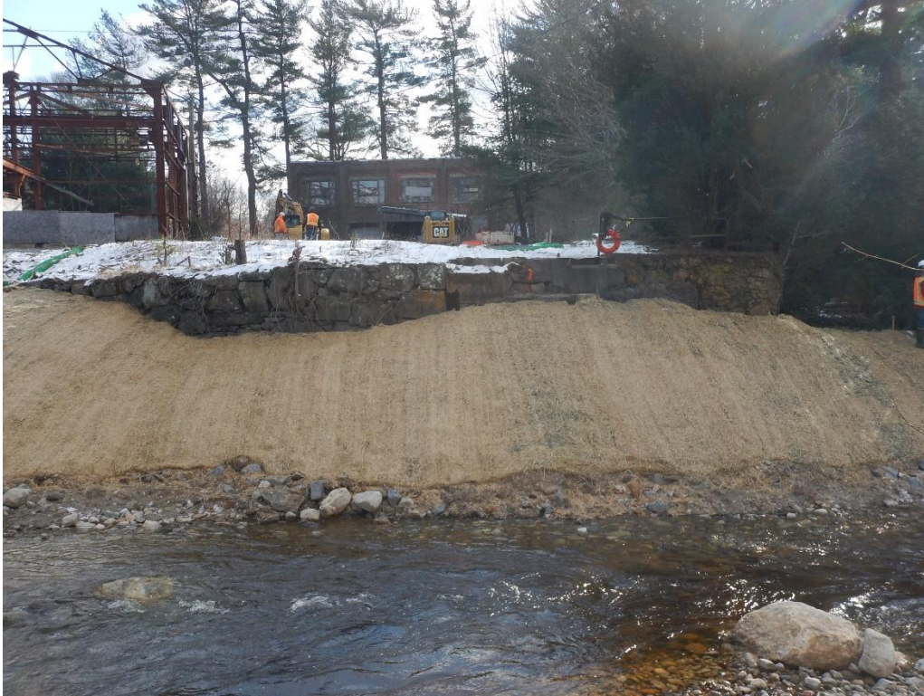
Photo 28: River left pipe outfalls and slope loamed and seeded (post-construction) (Gomez and Sullivan, 12/13/17)
