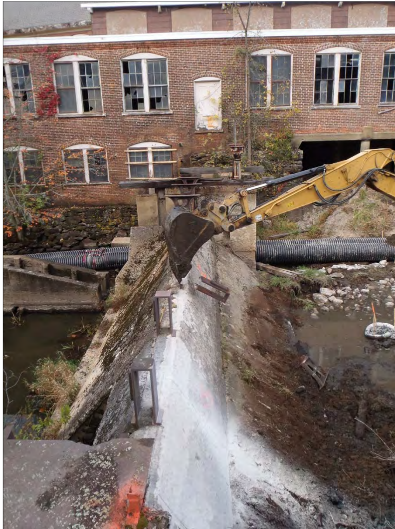
Figure 14. Removal of cast-iron stanchions from the dam crest, view northwest.
