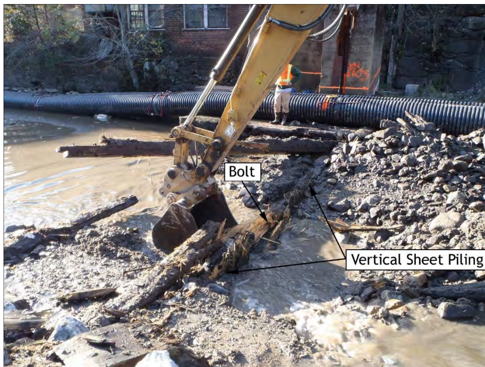
Figure 26. Excavation of two northern longitudinal timbers and attached vertical sheet piling, view west.
