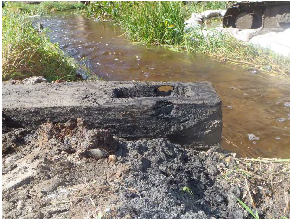
Figure 31. Mortise joint and bolt holes at one end of the intact timber exposed upstream of the Carver Cotton Gin Company Dam.
