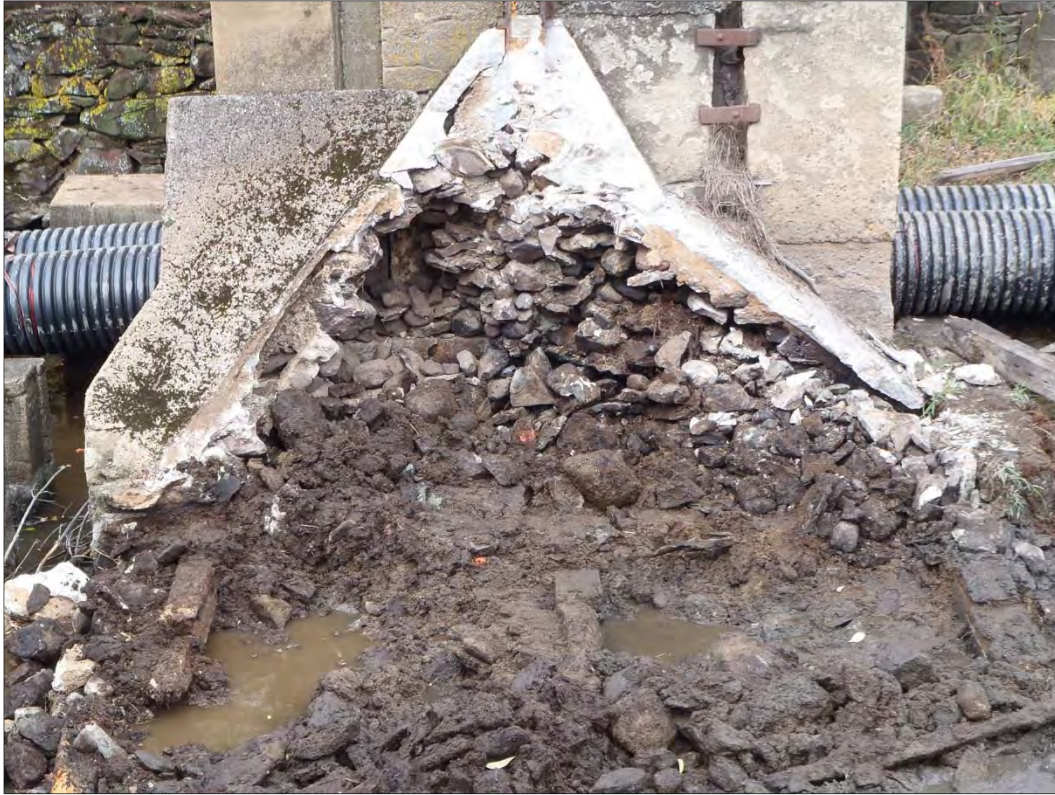
Figure 20. Western end of exposed longitudinal timbers anchored into concrete sluiceway floor, view northwest.
