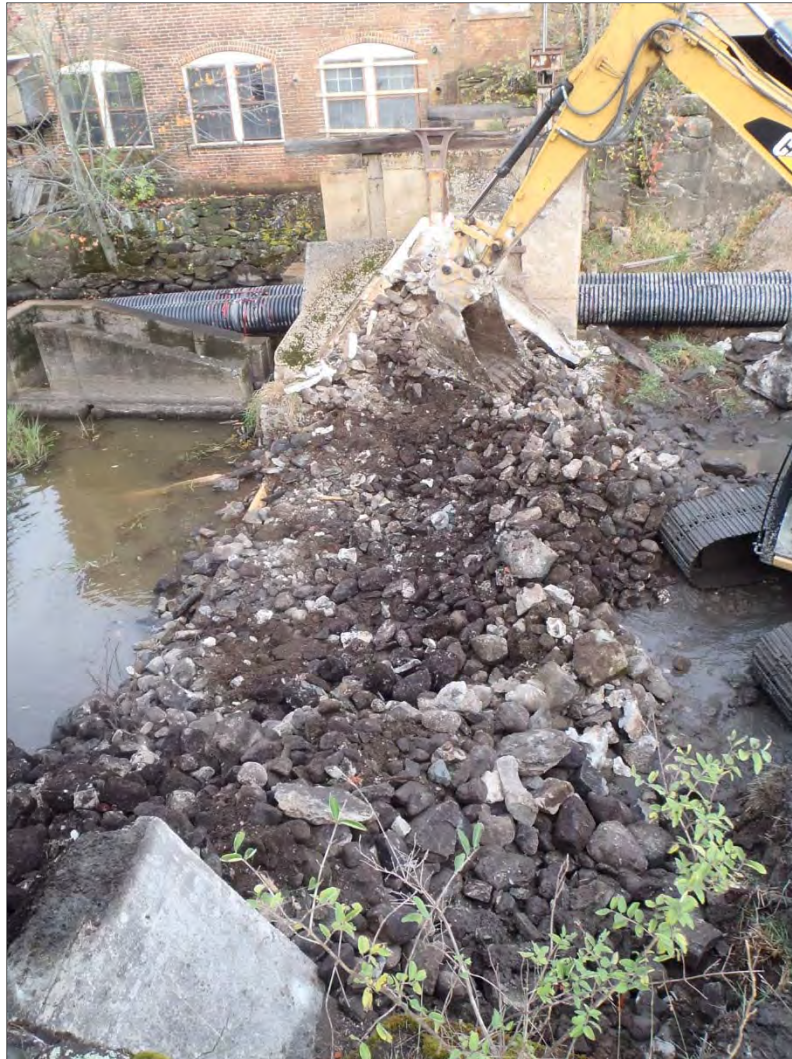
Figure 17. Excavation of rubblestone and cobble core of dam, view northwest.
