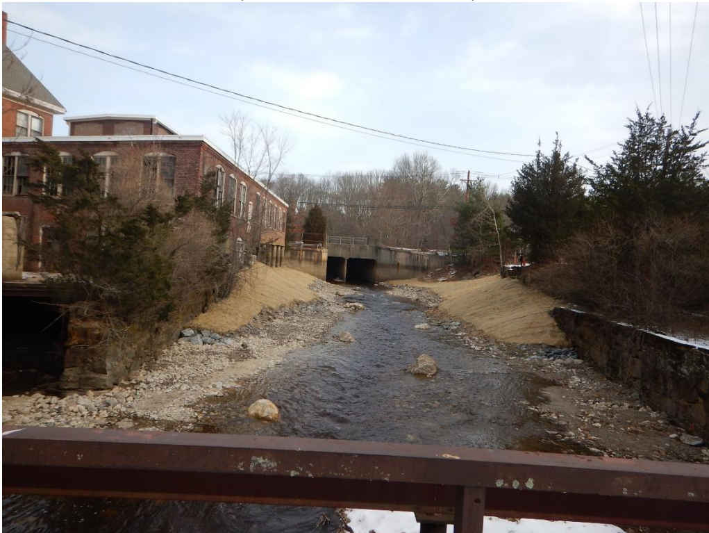
Photo 22: Looking upstream at constructed channel and removed dam (post-construction) (Gomez and Sullivan, 12/13/17)
