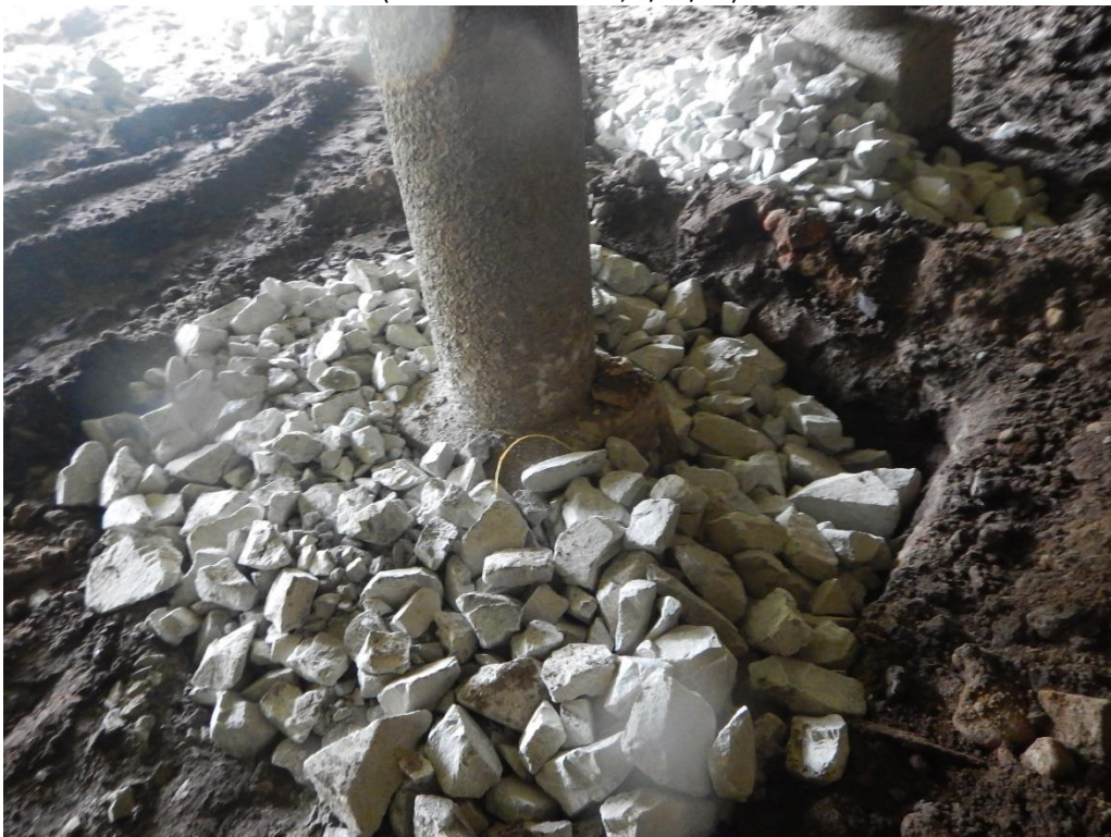
Photo 20: Mill building pier foundation protection (mid-construction) (Gomez and Sullivan, 9/22/17)
