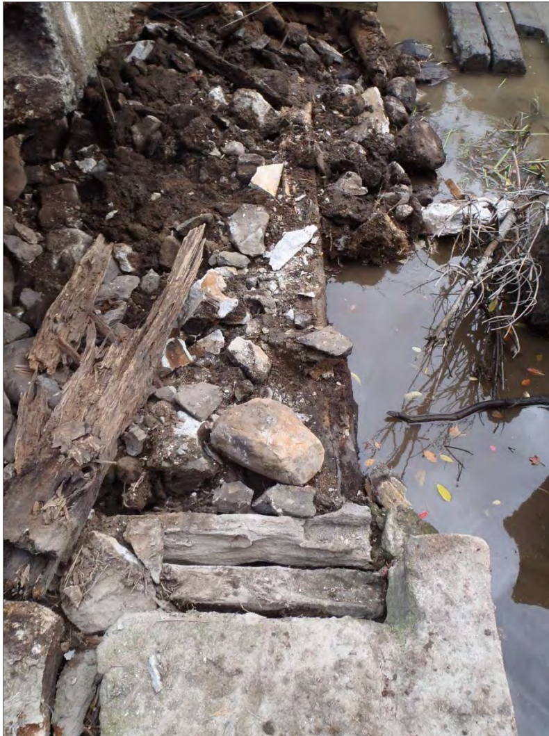
Figure 21. Detail of west end of longitudinal timber anchored into concrete sluiceway floor, view southeast.
