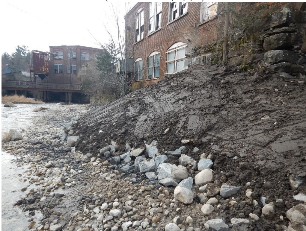
Photo 23: Looking downstream at river right stabilized abutment (mid-construction) (Gomez and Sullivan, 12/8/17)
