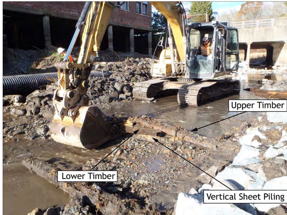
Figure 23. Removal of northern longitudinal timbers showing vertical truncated sheet piling, and upper and lower timbers, view northeast.
