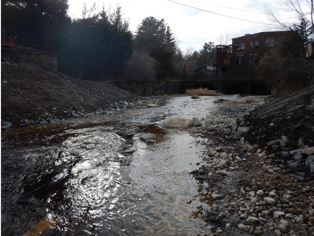
Photo 26: River right stabilized abutment, loamed, and seeded with loam (post-construction) (Gomez and Sullivan, 12/13/17)
