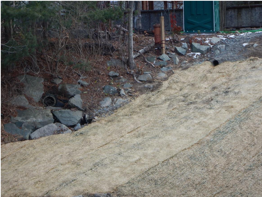
Photo 28: River left pipe outfalls and slope loamed and seeded (post-construction) (Gomez and Sullivan, 12/13/17)
