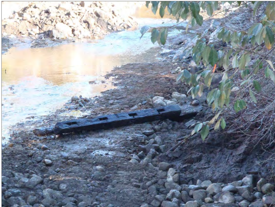
Figure 36. Mortise joints on one of the timbers exposed downstream of the Carver Cotton Gin Company Dam.
