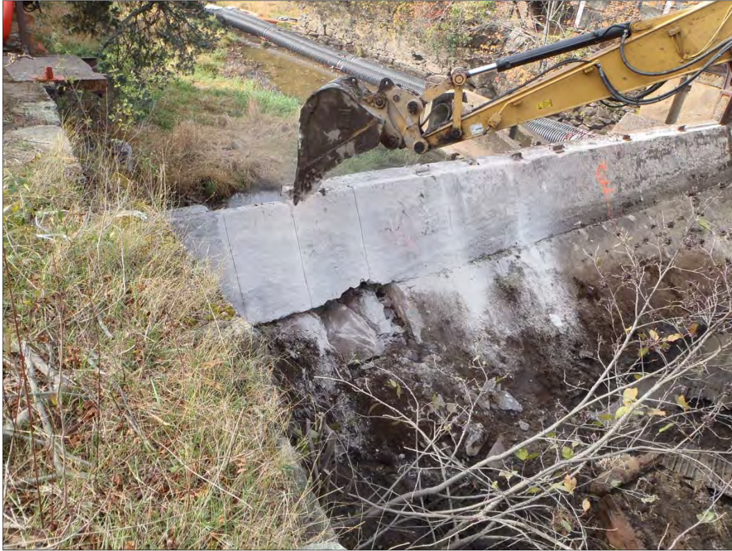
Figure 15. Removal of saw-cut concrete from dam spillway, view southwest.
