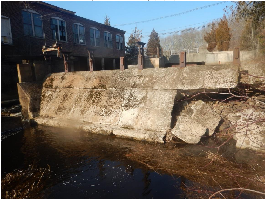
Photo 2: Downstream face of dam looking at rubble fill exposed on right (pre-construction) (Gomez and Sullivan, 3/18/16)
