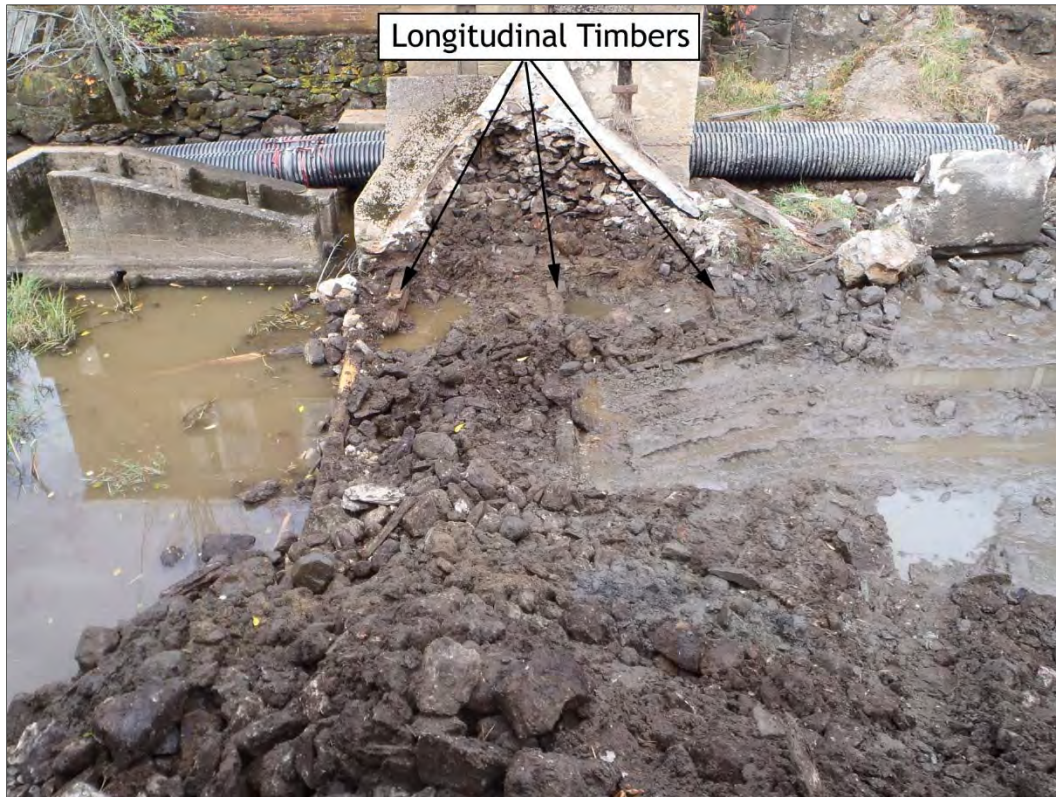
Figure 18. Three longitudinal timbers exposed below the rubblestone and cobble core of the dam, view northwest.
