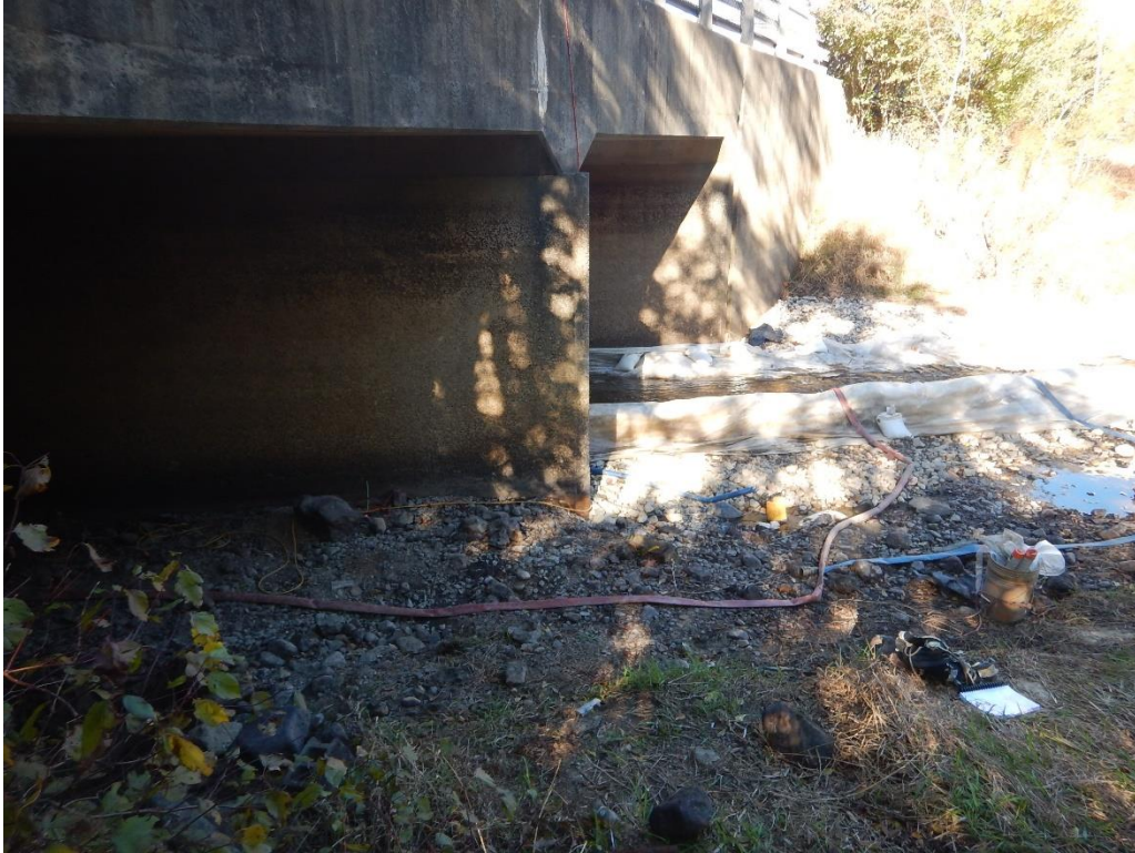
Photo 14: Partially removed dam with exposed material (mid-construction) (Gomez and Sullivan, 10/24/17)
