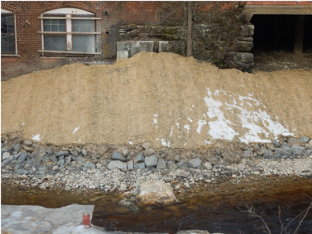
Photo 26: River right stabilized abutment, loamed, and seeded with loam (post-construction) (Gomez and Sullivan, 12/13/17)
