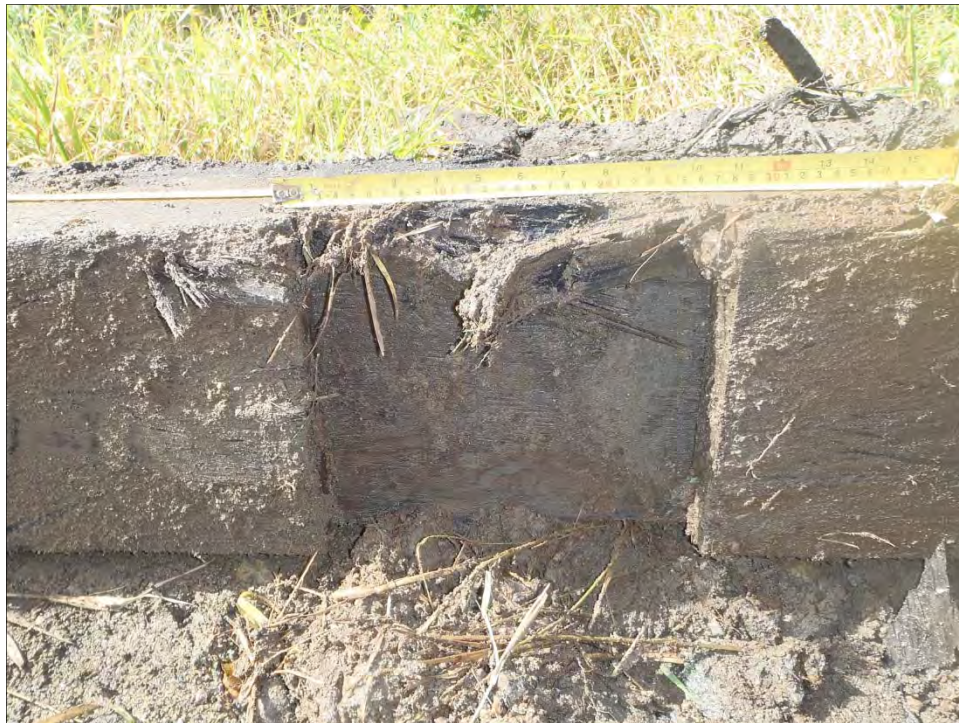
Figure 32. Rectangular notch on one side of the intact timber exposed upstream of the Carver Cotton Gin Company Dam.
