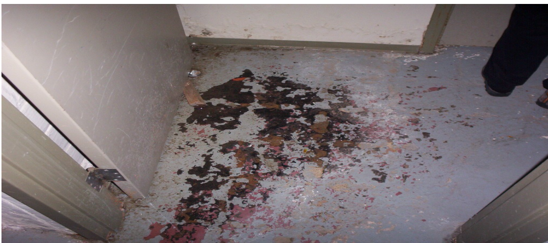
705-1 Family Housing Development, Armitage Arms Common Area, Laundry Room – Paint Peeling From Floor Due to Water Leak
