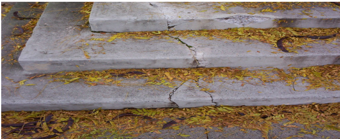
705-1 – Family Housing Development, Armitage Arms Common Area, Rear Entrance – Stairs Cracked and in Need of Repair
