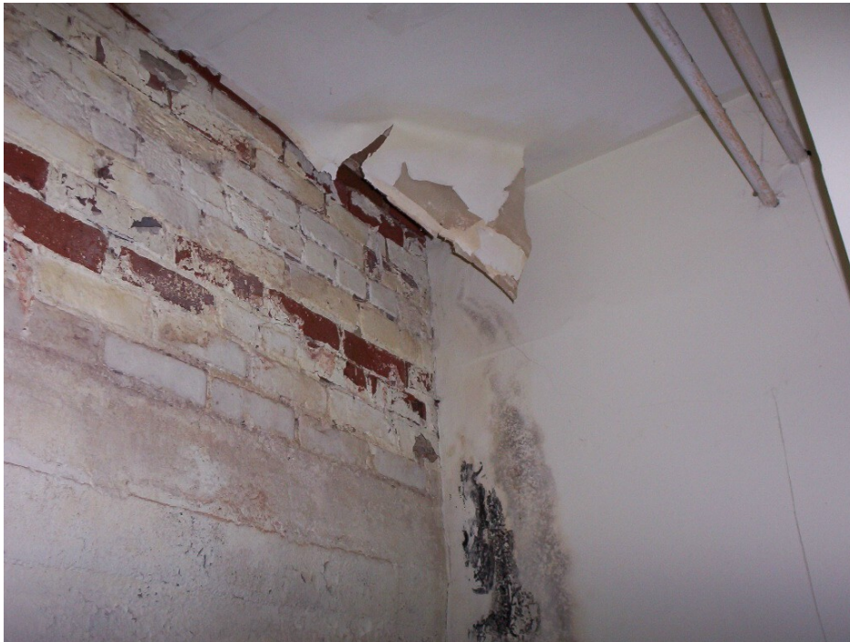
705-1 Family Housing Development, Armitage Arms Common Area, Laundry Room – Paint Peeling From Floor Due to Water Leak
