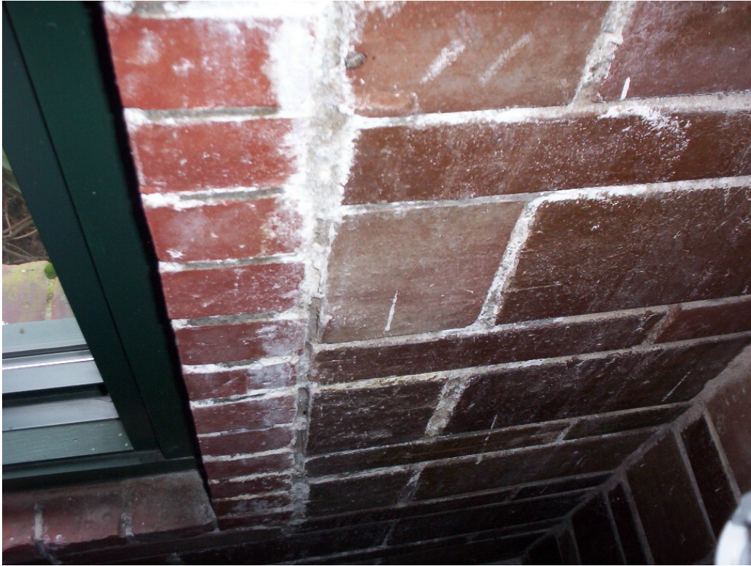
705-1 – Family Housing Development, Armitage Arms Common Area, Rear Entrance – Stairs Cracked and in Need of Repair
