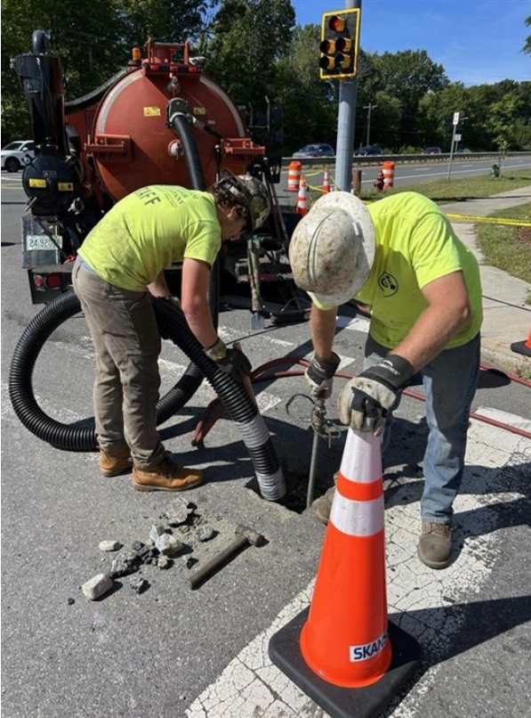
Test pit sampling Rourke Bridge, Lowell
