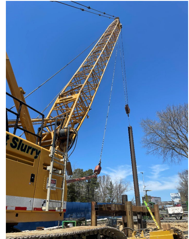
Piles driven 75-90ft deep to gather data for foundation design
