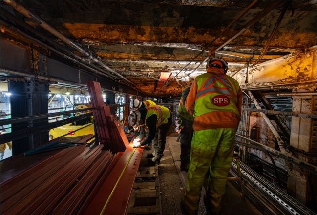
MBTA Green Line trough work
