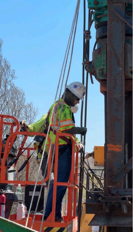
Sagamore Bridge Foundation load testing
