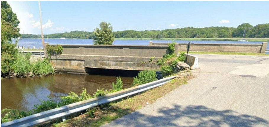
Dighton: Pleasant Street over Muddy Cove bridge replacement of 100+ year old structure
