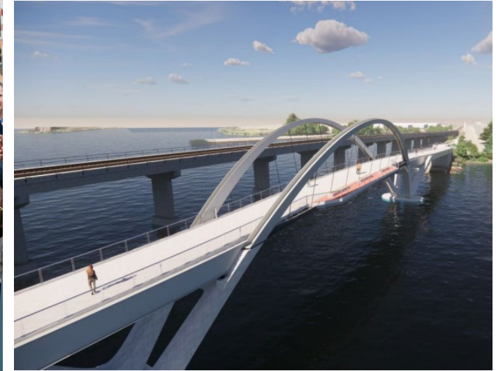
Mystic River Bicycle / Pedestrian Bridge
