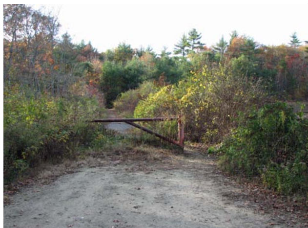
Road across West Meadow Pond Dam; note the extent of vegetation to both the downstream (left) and pond (right) sides of the dam. (See Appendix K for photo information.)
