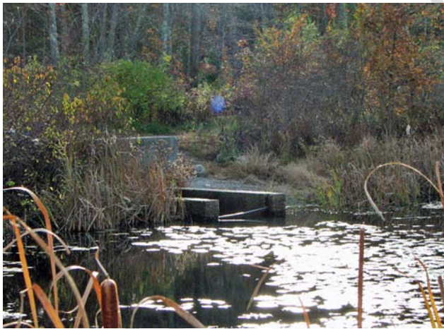
Spillway of West Meadow Pond Dam; the vegetation along the dam is visible to both sides of the spillway. (See Appendix K for photo information.)
