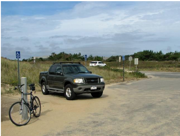
HP parking at Left Fork lot; note the absence of pavement markings, access aisles, and signs identifying van accessible spaces. (See Appendix G for photo information.)
