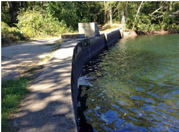
Upstream face of Pud's Pond Dam. This dam and associated dikes are in Poor condition and have over 30 identified deficiencies (Weston & Sampson 2008a). (See Appendix K for photo information.)
