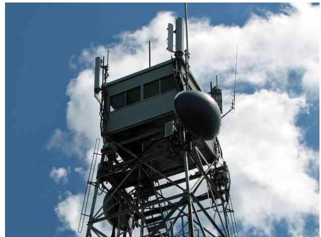
Typical fire observation tower cabin; note the telecommunications equipment mounted on the cabin and top of the tower. (See Appendix G for photo information.)
