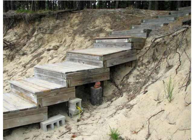
Stairs from the shore to campsites are repeatedly undermined by storms, resulting in an ongoing maintenance need. (See Appendix G for photo information.)
