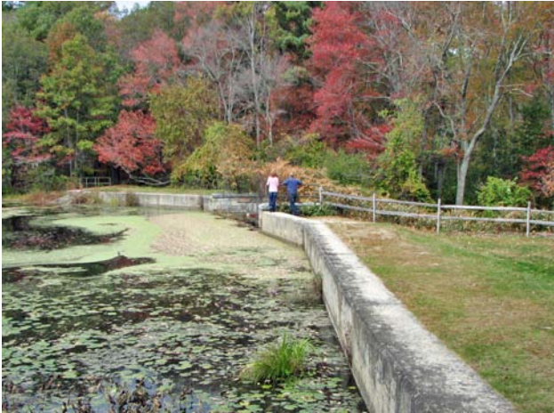
Stony Brook Dam was reconstructed in the mid-1960s following a breach. It currently maintains water levels in Stony Brook Pond. (See Appendix K for photo information.)
