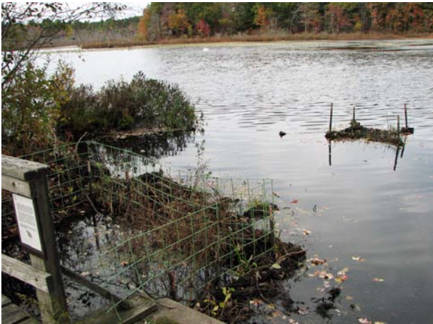
Beaver deceiver showing materials blocking both the main flow under Spillway #2 and the offshore culvert. (See Appendix K for photo information.)
